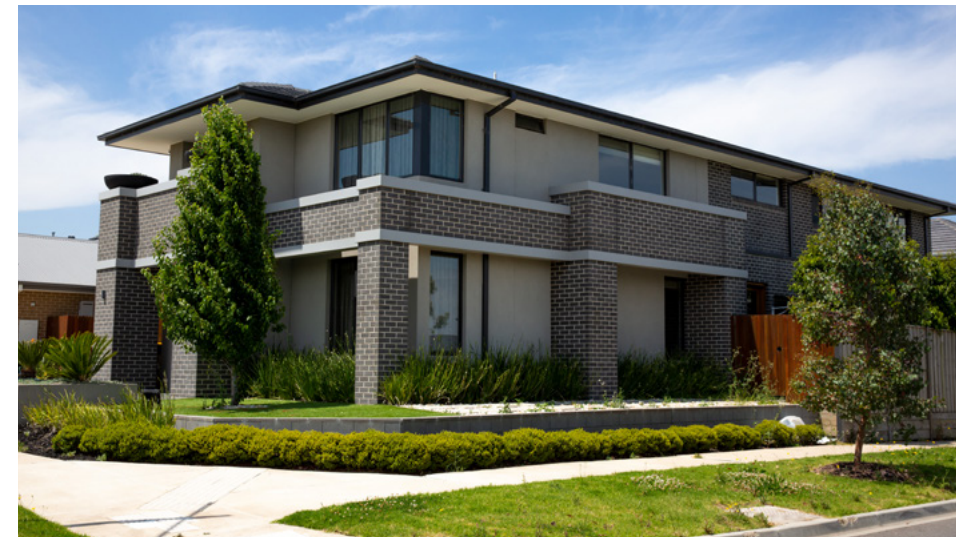
Double Storey Corner Treatment. Credit: Porter Davis
