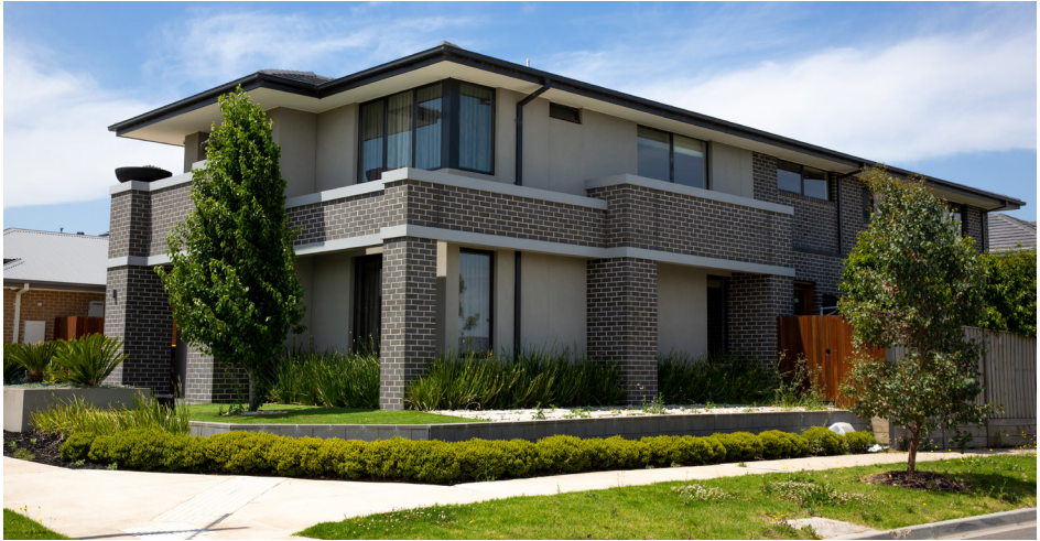
Double Storey Corner Treatment. Credit: Porter Davis
