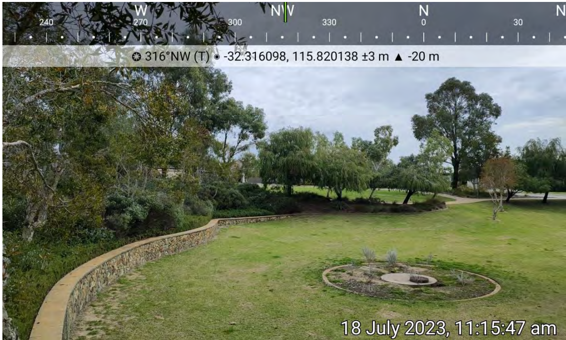
Plate 11: Evidence of external POS and landscaping areas being maintained to low threat as per clause 2.2.3.2 (f) in AS 3959.
