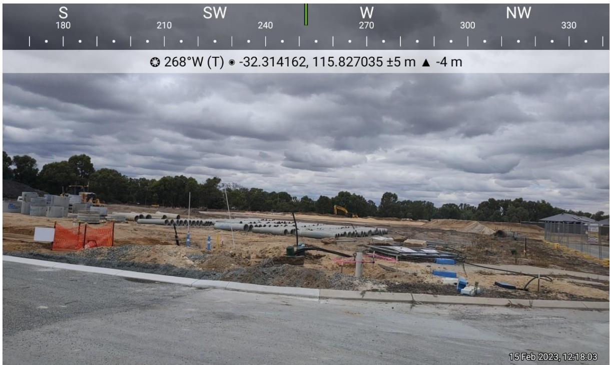
Plate 7: Evidence of installation of reticulated water within construction site is underway.
