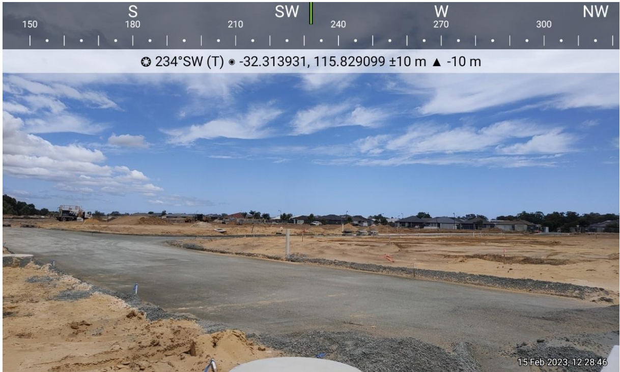
Plate 5: Evidence of construction of roads in accordance with Roadworks layout plan.
