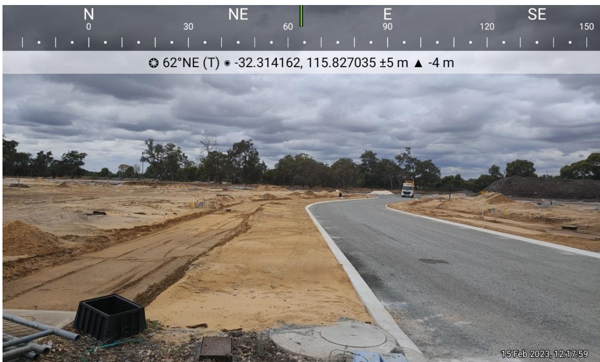
Plate 4: Evidence of construction of roads in accordance with Roadworks layout plan.
