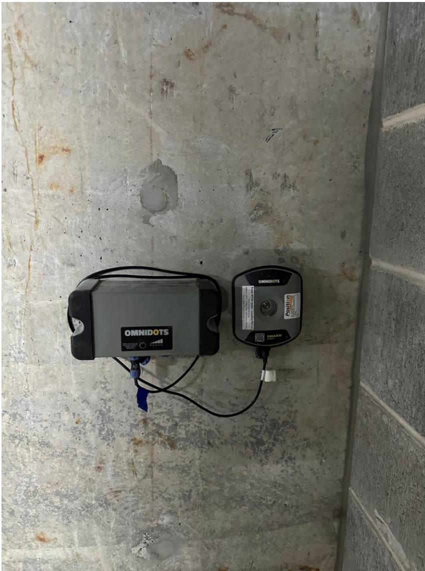
Figure 3 Location 1 – Building C1, B2 Carpark – vibration monitoring.
