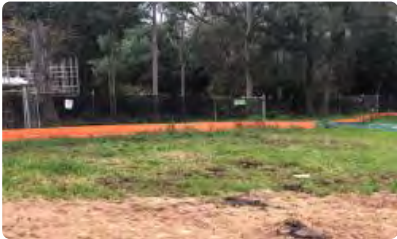
Sediment fence and tree protection zone arc
