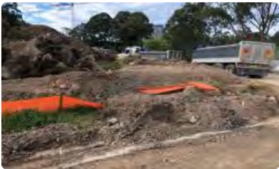
Repair silt fence around stockpile
