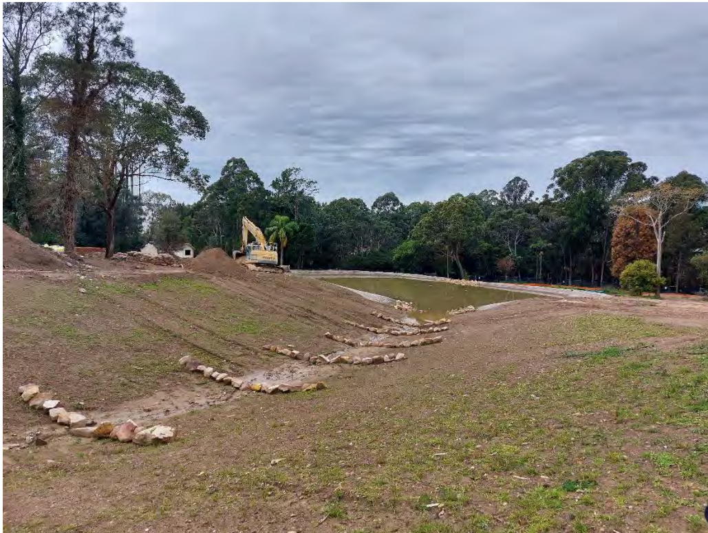
6. Swale in northern portion of site.
