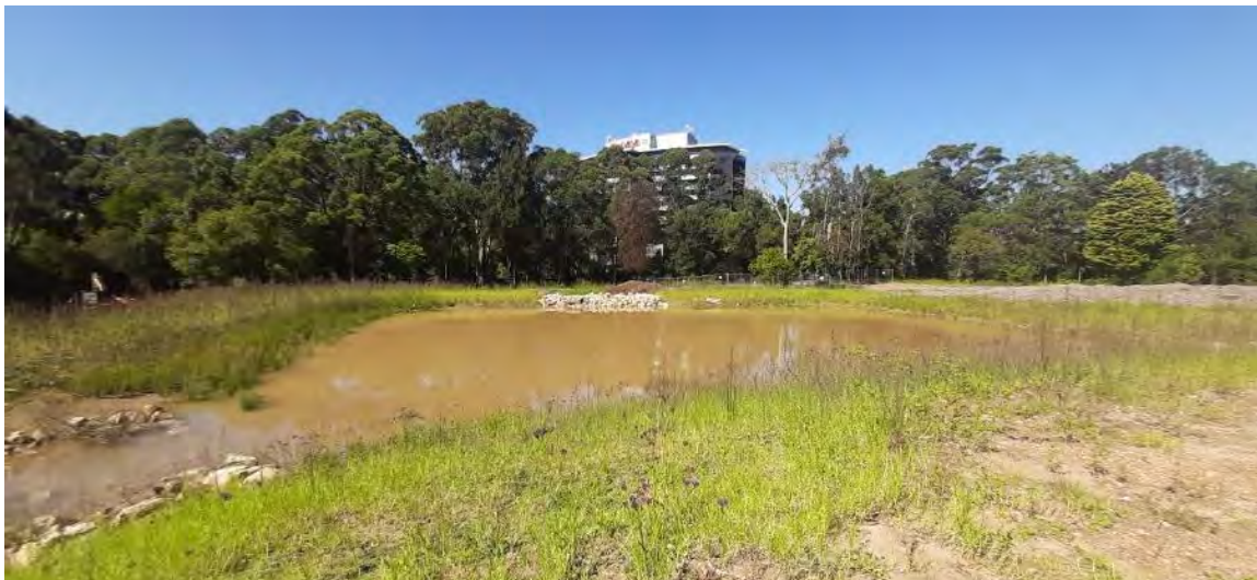
15. Sedimentation basin – facing south south south west.
