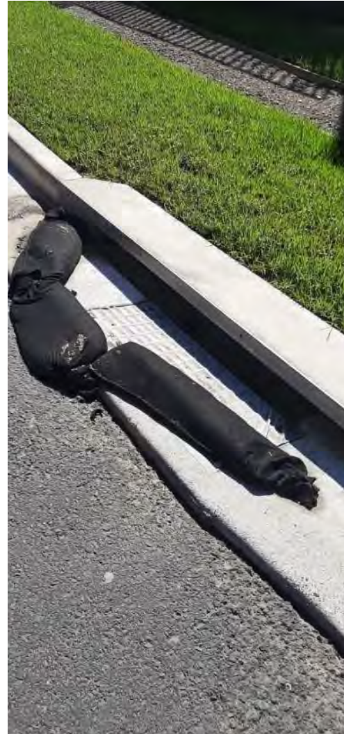
12. Stormwater drain downstream along eastern side of access road.
