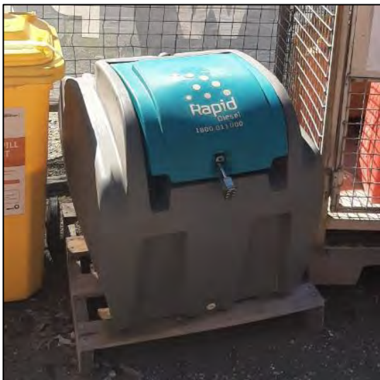
9. Secure storage for diesel.
