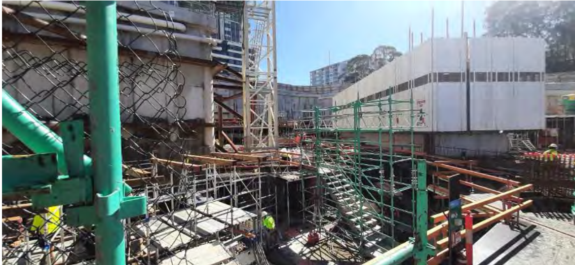
4. Worksite at A1 building
