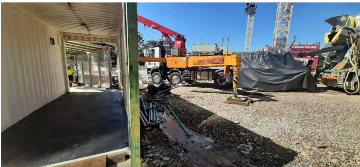
6. Concrete vehicles onsite.
