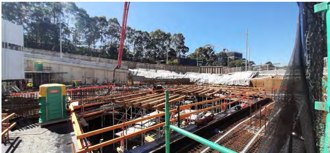
5. Construction in progress of basement levels of A1 building.
