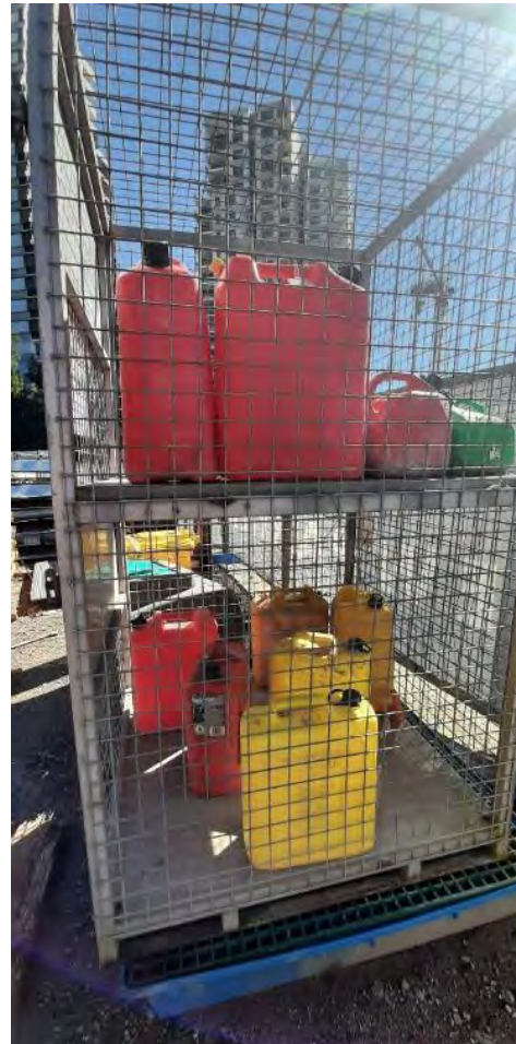
8. Flammable fuel in locked cage.
