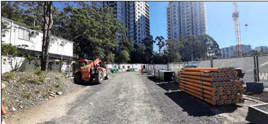
2. Site office (left) and storage of material (right).
