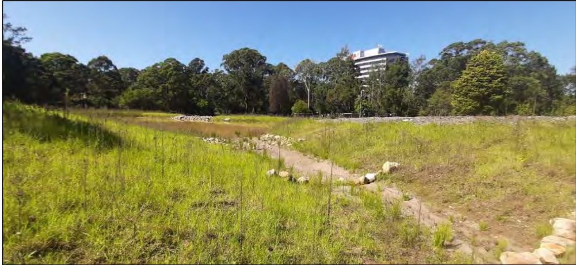
14. South western swale drain – facing south towards sedimentation basin.
