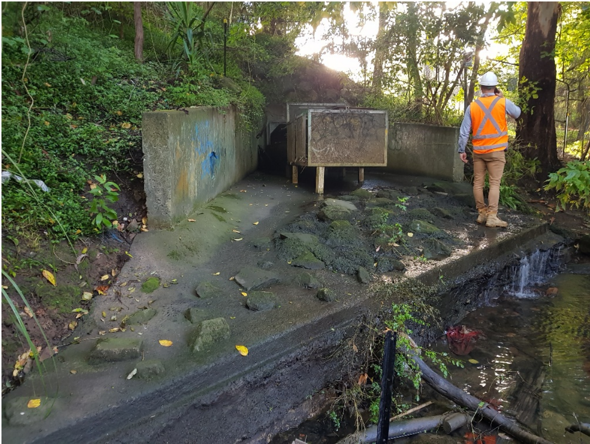
Figure 3: Existing 1200mm Headwall
