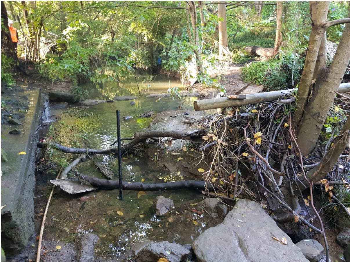
Figure 2: Debris and Obstructions in Creek Channel
