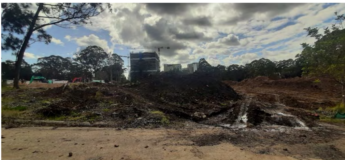
12. Mulch stockpiles in southern portion of site – facing northeast.
