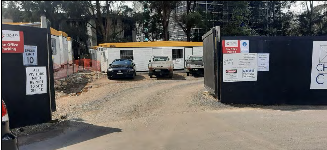
1. Entrance to Christie Civil site office – facing east from access road.
