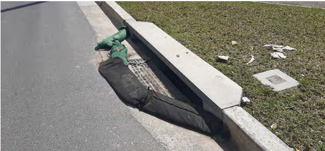
28. Silt bags and fabric filter installed around stormwater drain along Road 1.
