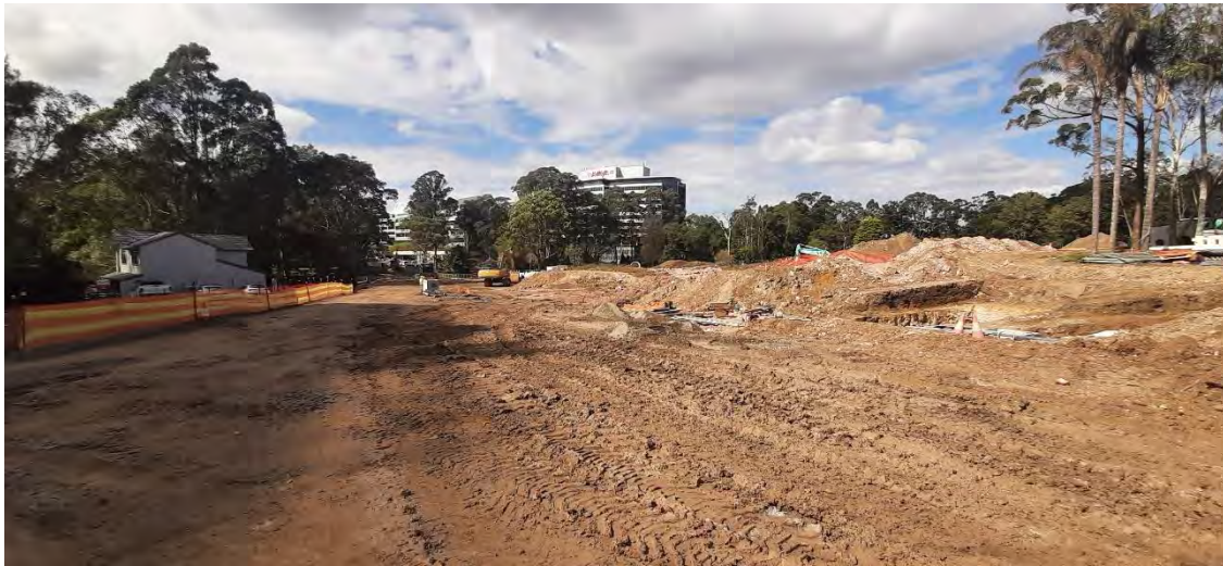
5. Earthworks in progress – facing southeast towards Shrimpton Creek.
