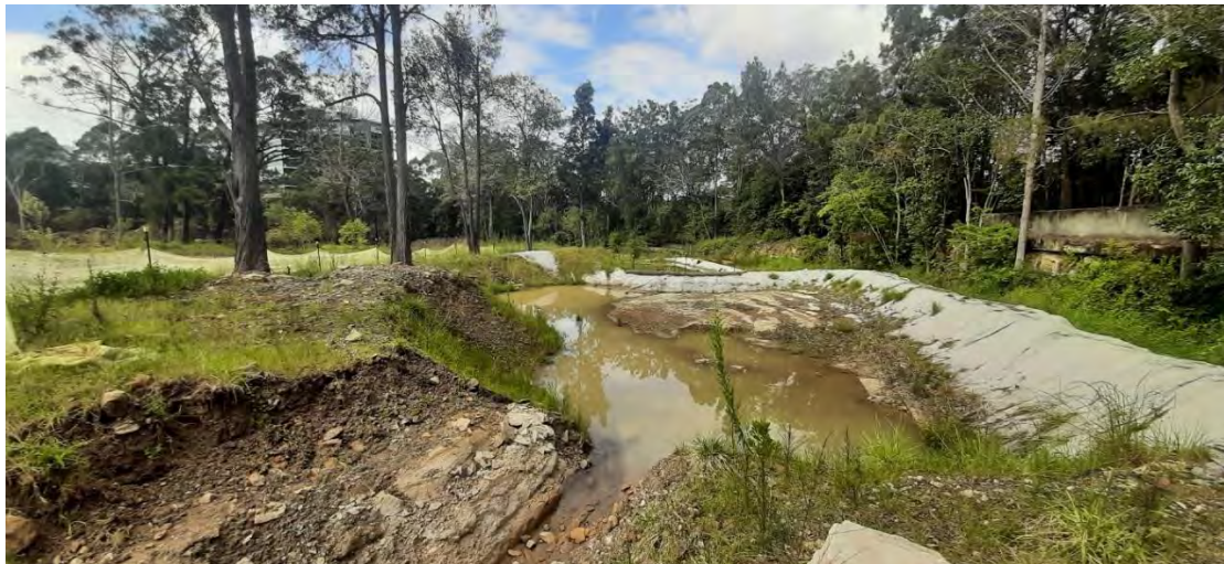
8. The initial and furthest upslope sedimentation retention basin in the southwestern portion of the site - facing south with trees lining the southwestern boundary beyond.
