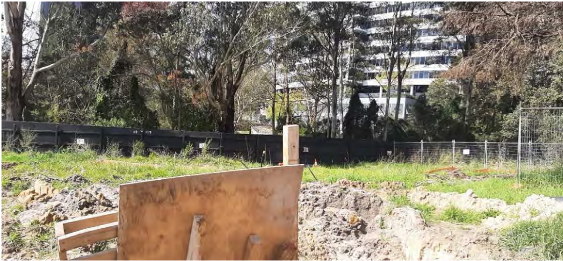
13. Class A hoarding installed around the site - facing east.
