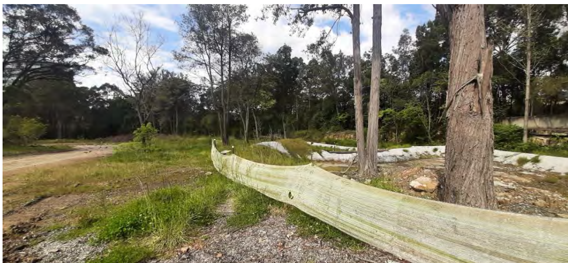
9. Silt fence present with the sedimentation retention ponds beyond (right).
