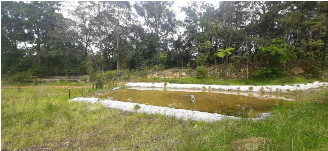
10. The second and main sedimentation retention basin. Water appeared clear with no signs of algae, visual and / or olfactory signs of contamination.
