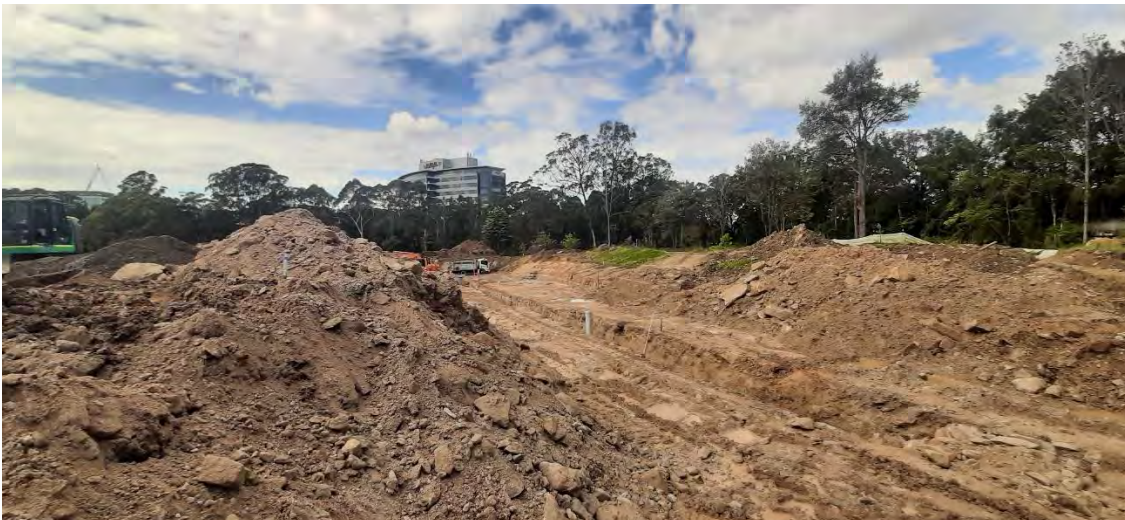
6. Excavation and installation of stormwater drainage
