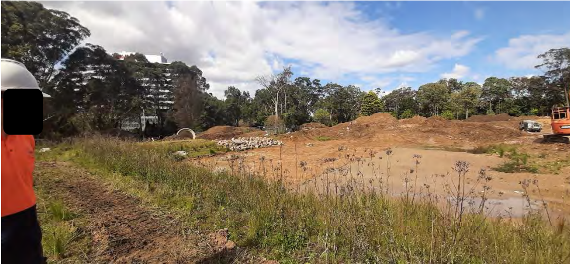
4. Sedimentation basin in central portion of site – drained and desilted.
