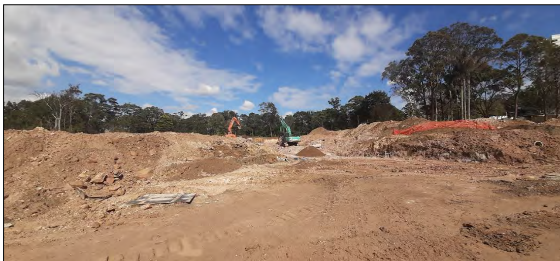
3. Earthworks in progress - facing west from eastern corner of site.
