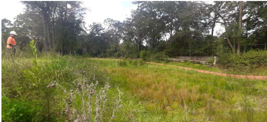
11. Overflow water from sedimentation retention basin being discharged into grassy area. Vegetation appears healthy with no signs of die-back or signs of contamination.
