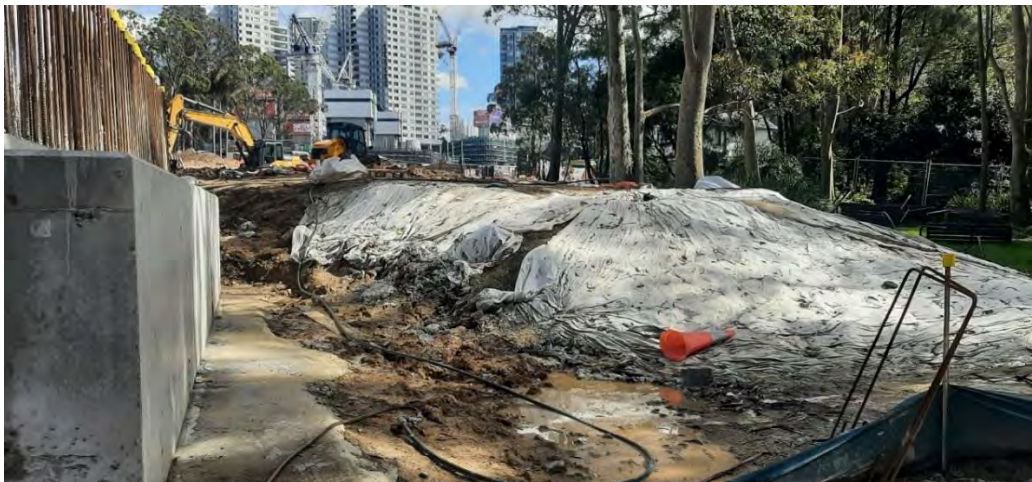
20. Covered stockpile in area southeast of Shrimpton Creek.
