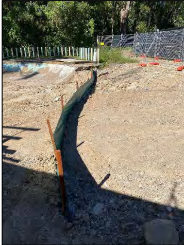
13. Additional silt fence installed upslope from Shrimptons Creek 31/03/2023.
