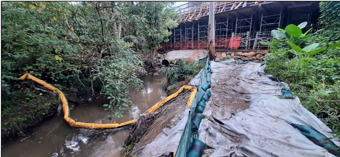
18. Siltfences re-erected along Shrimptons Creek. 29/03/2023
