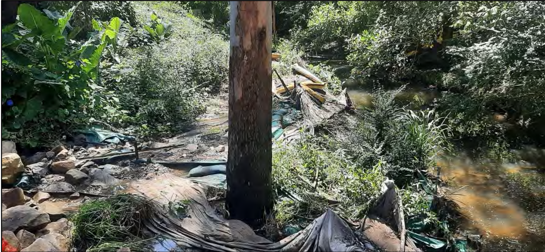
17. Collapsed siltfences noted along western bank of Shrimptons Creek – downstream from bridgeworks. 15/03/2023
