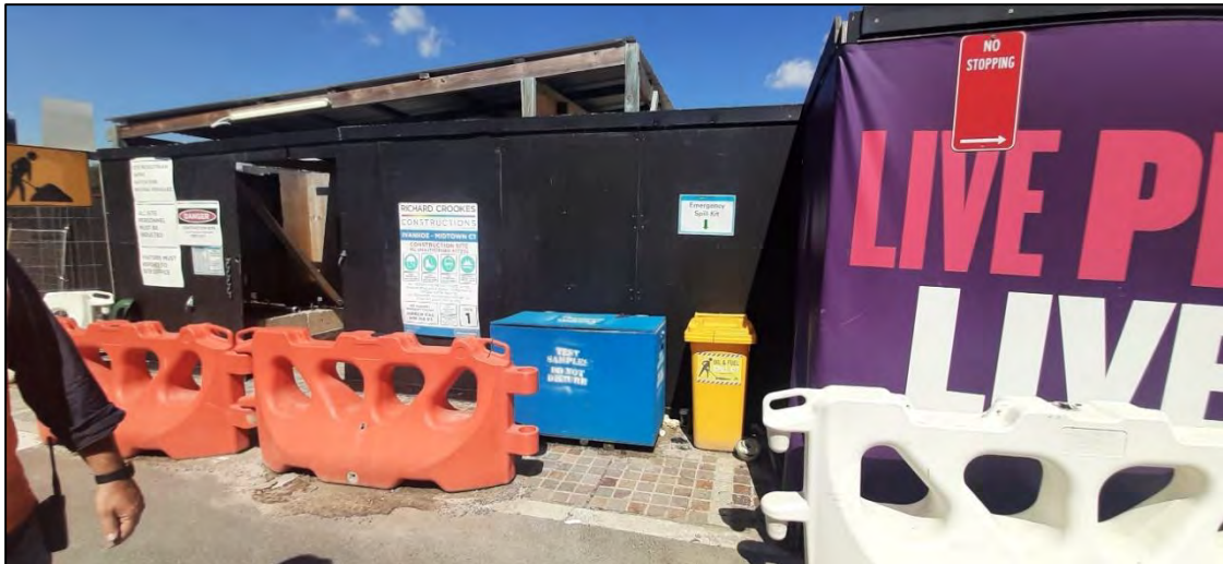
4. Personnel entrance to Richard Crookes Constructions work site on Road 1. 15/03/2023
