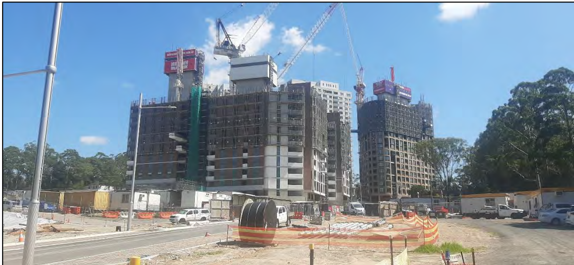
1. Building C1– facing northwest from south-eastern portion of site. 15/03/2023
