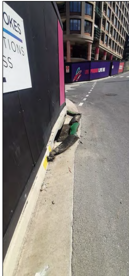
3. Silt bags and fabric filter installed around stormwater drain along Road 1. 15/03/2023
