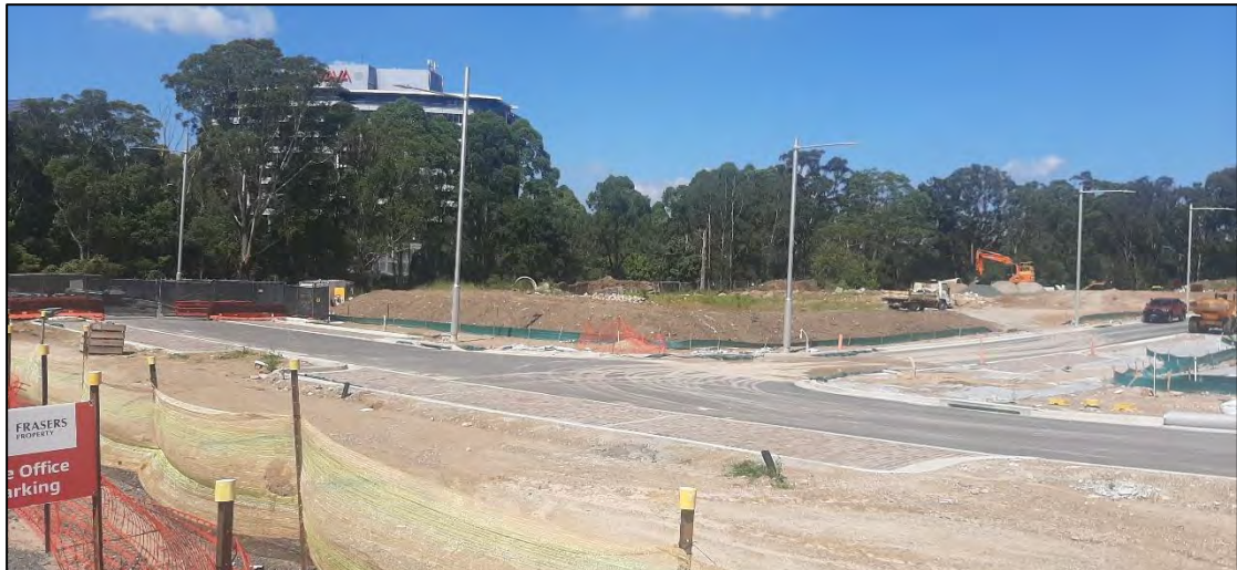
10. Facing south towards Stage 1B road construction works. 15/03/2023
