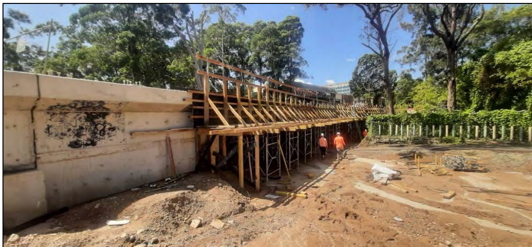
11. Bridgeworks over Shrimptons Creek - facing southeast. 15/03/2023
