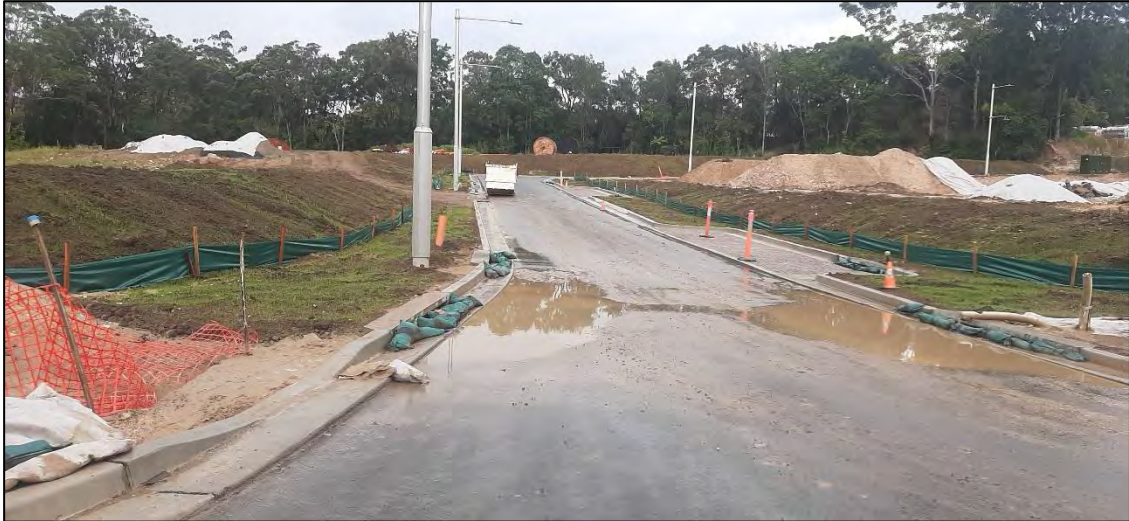
23. Newly seeded soil batters along access road 2 – facing south west. 29/03/2023
