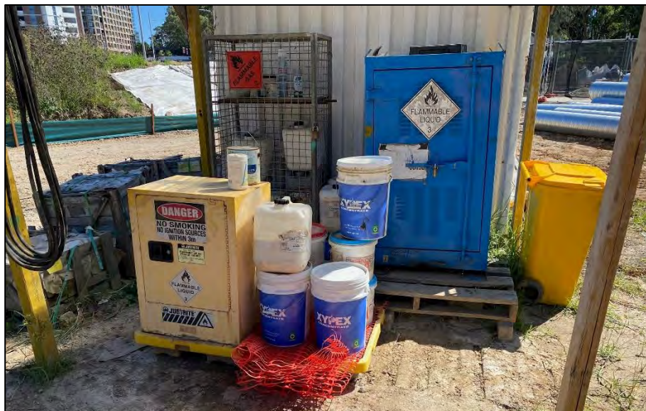
21. Hazardous storage area with locked cages and cabinets and spill kit. 31/03/2023
