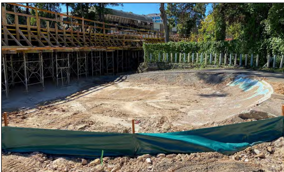
12. Additional siltfences erected upslope of bridgeworks. 31/03/2023
