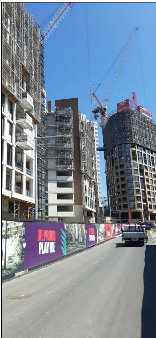
2. Class A hoarding installed along road 1 - facing northwest. 15/03/2023
