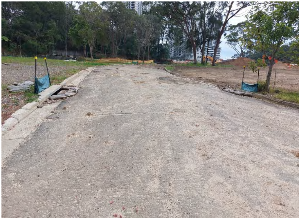
12. Erosion and sediment control – silt socks in place along Road 2.
