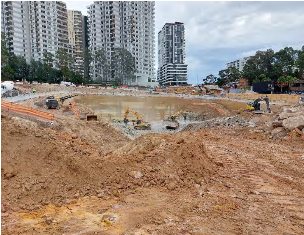
16. Site activities on the day of performance review audit inspection.
