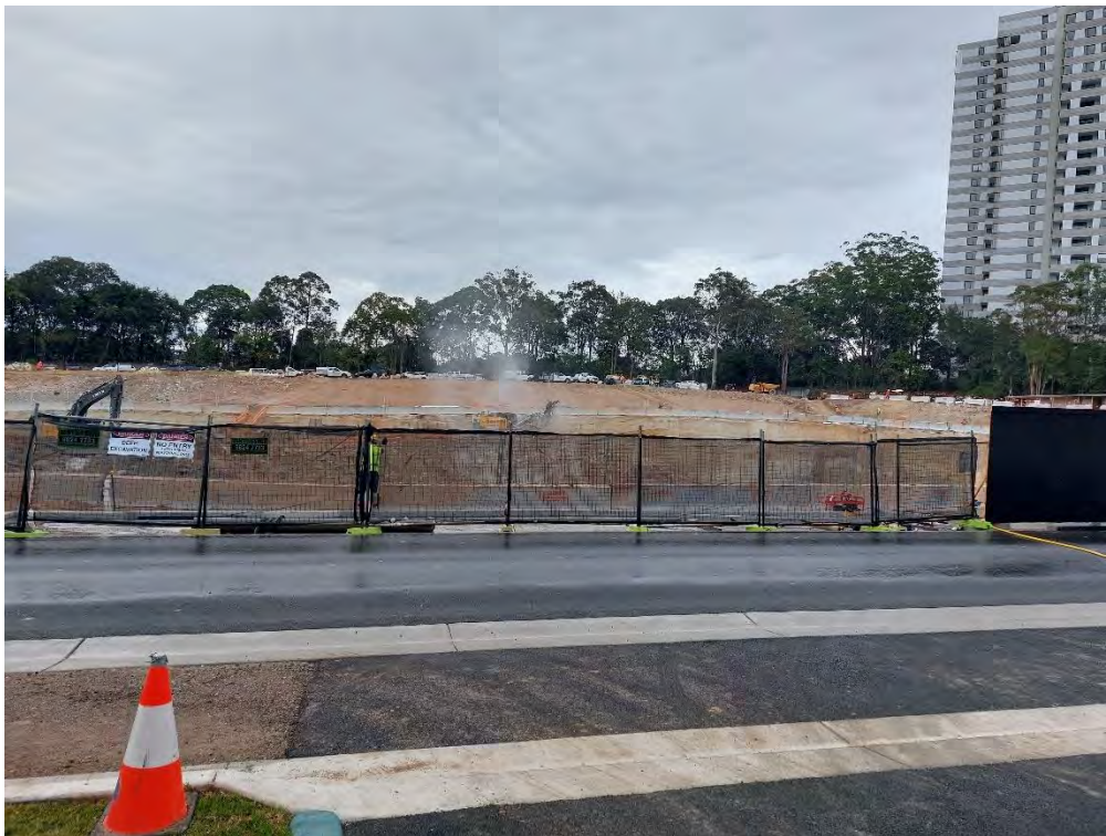
2. Application of mist water for general dust suppression.
