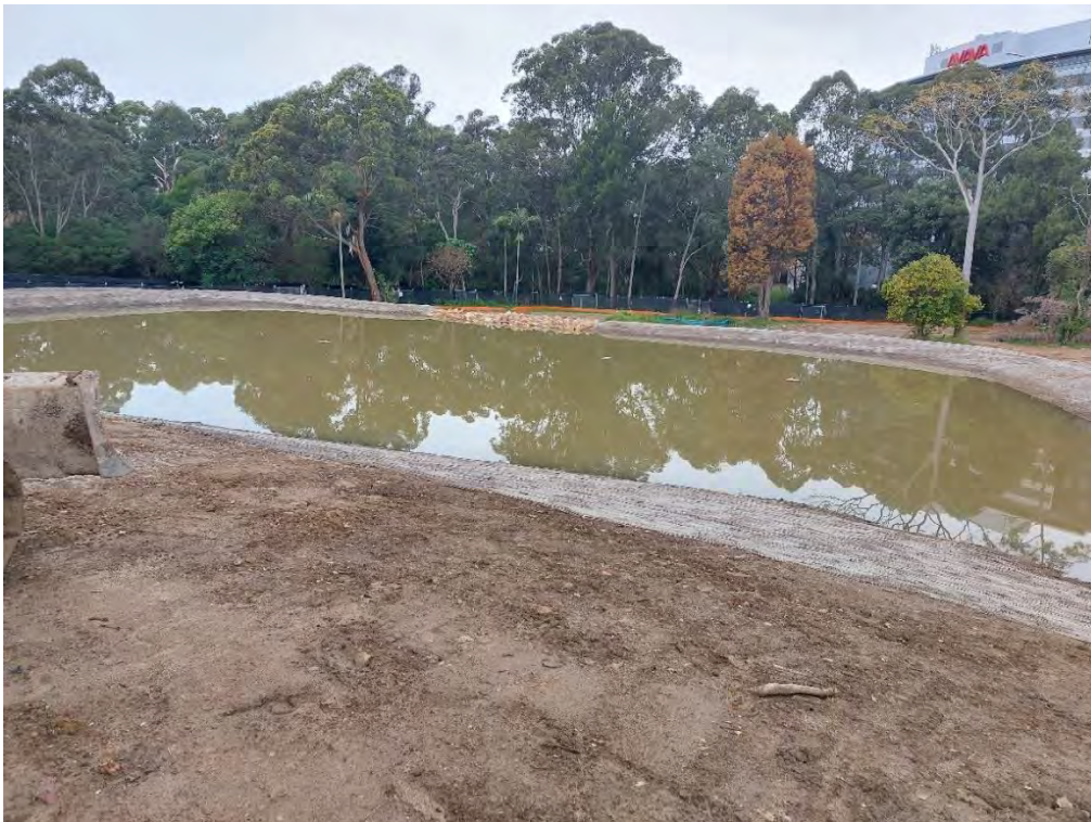
4. Sediment basin in eastern portion of the site.
