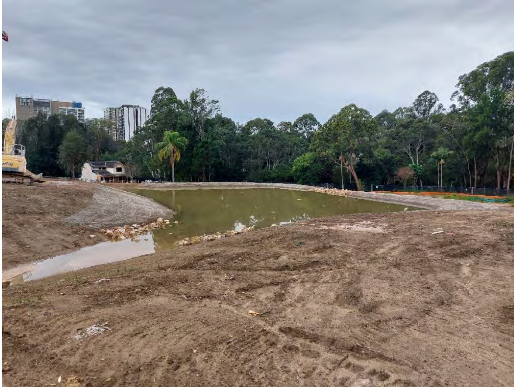
5. Sediment basin in eastern portion of the site.
