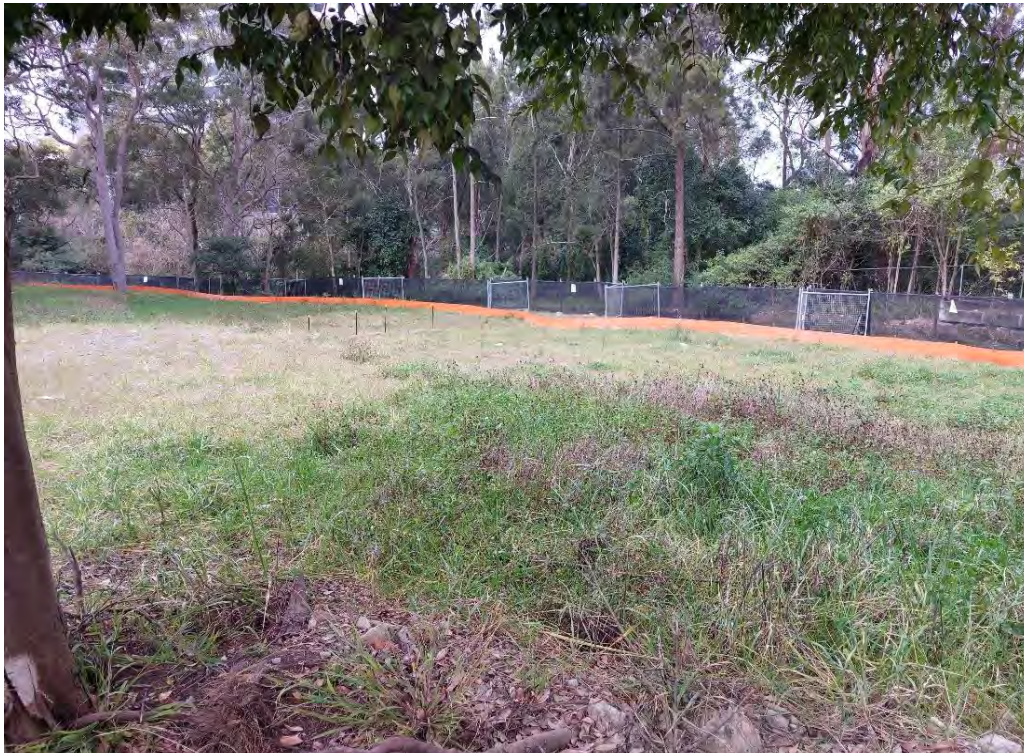
10. Erosion and sediment control – silt fencing in good condition.
