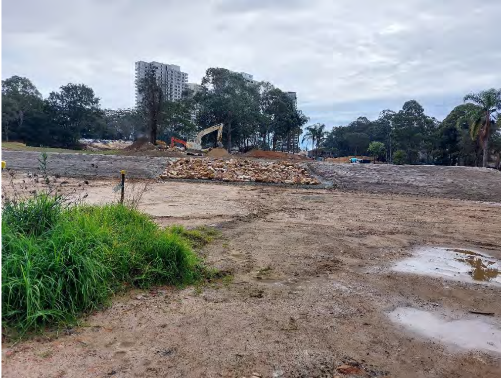
7. View of sediment basin (facing west).
