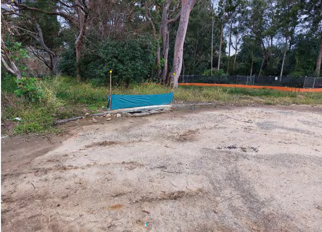
11. Erosion and sediment control – eastern portion of site (Road 2).
