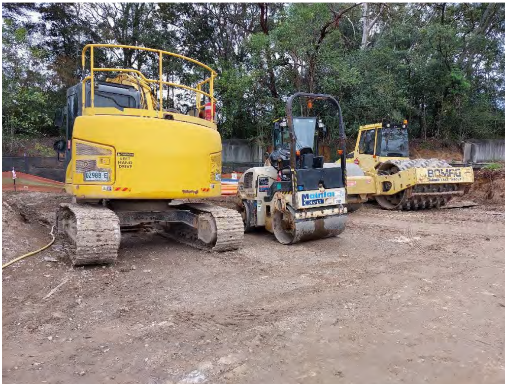
18. Good housekeeping: No staining on the ground surface.
