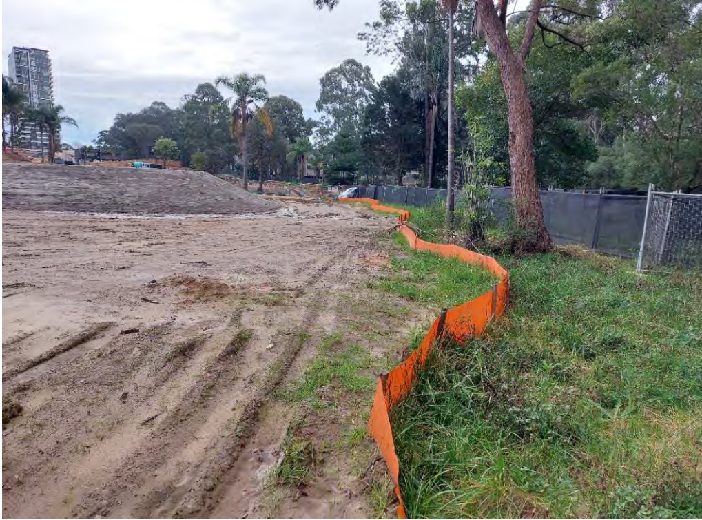
9. Erosion and sediment control – silt fencing in good condition.
