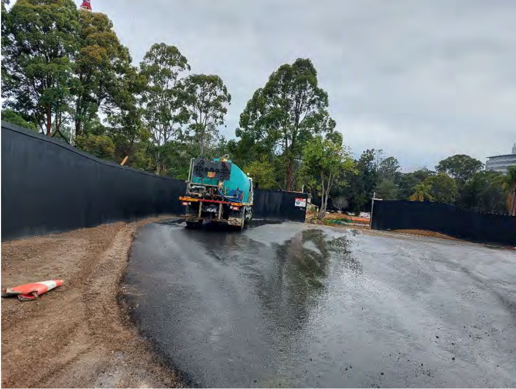
1. Water cart present onsite on day of site inspection.
