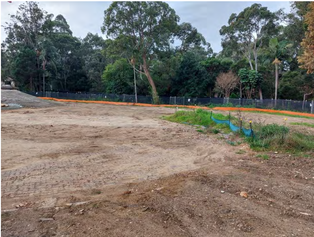
8. Erosion and sediment control east of sediment basin.
