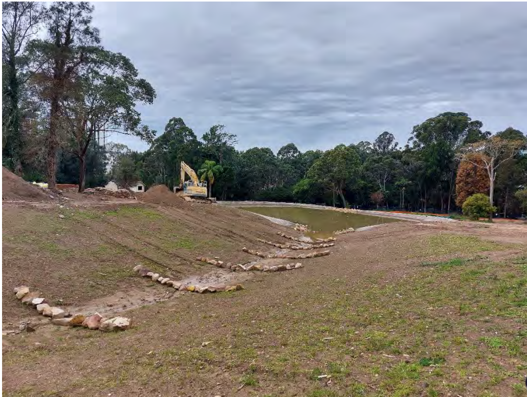
6. Swale in northern portion of site.
