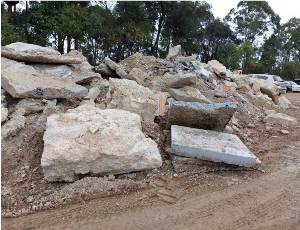
17. Recycled material stockpiled prior to removal
