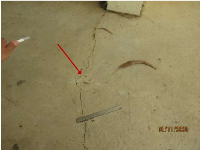
No 1-3_553_Note the cracking damage
