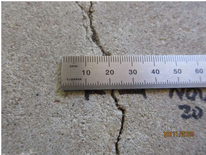
No 1-3_345_Note an estimated 1.0mm cracking width at representative location
