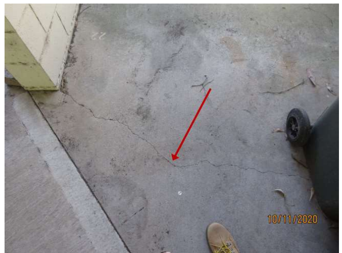
No 1-3_502_Note the cracking damage
