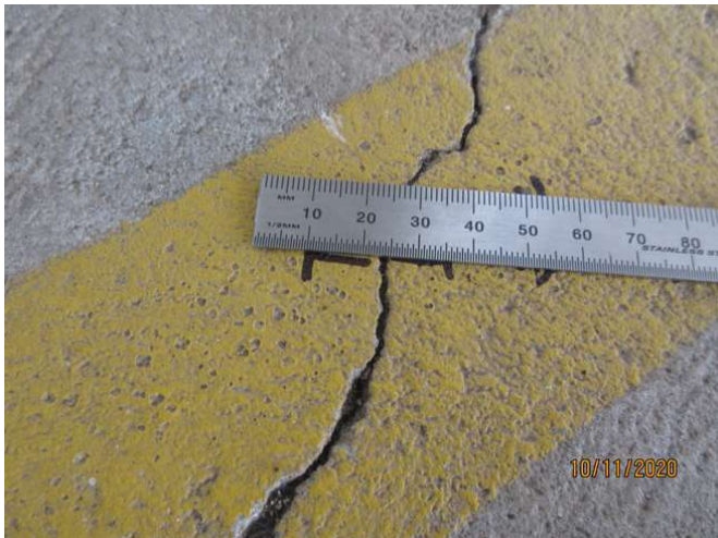
No 5_159_Note an estimated 2.0mm cracking width at representative location
