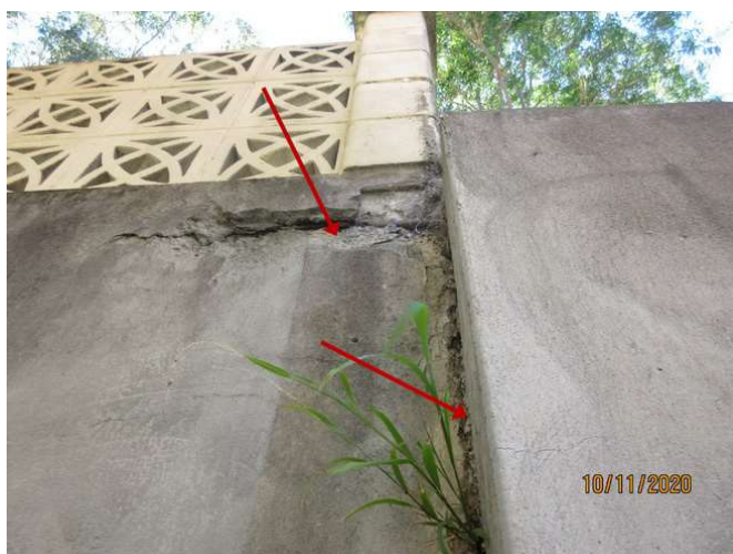
No 155_035_Spalling damage to concrete retaining wall
