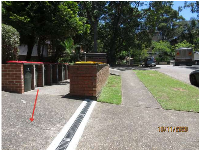
No1_003_Note evident cracking to concrete driveway
