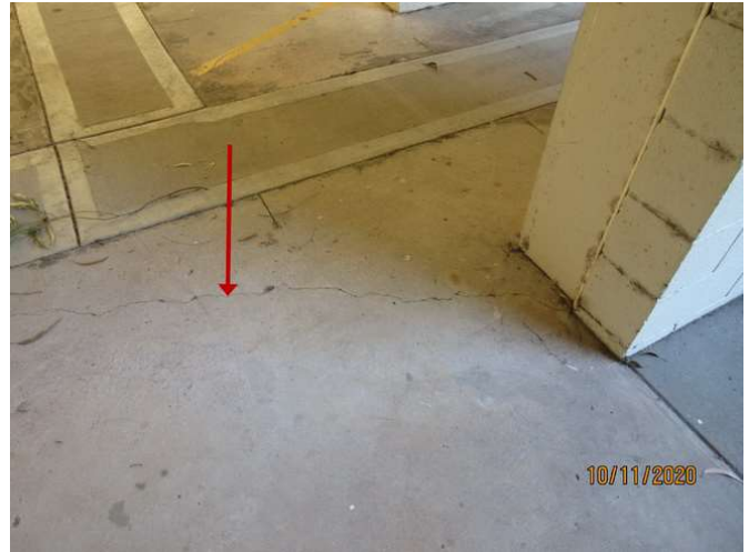
No 1-3_536_Note the cracking damage
