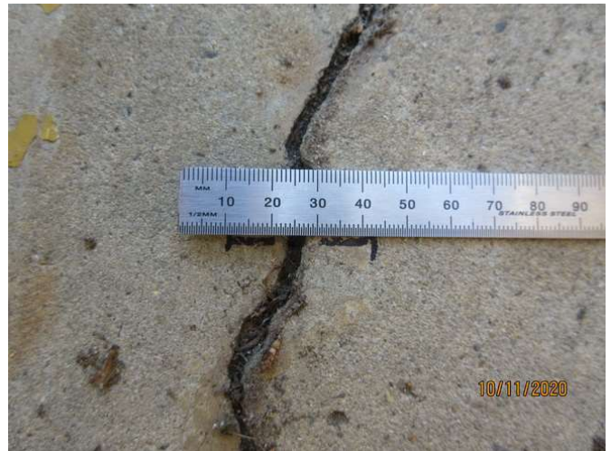
No 1-3_184_Note an estimated 3.5mm cracking width at representative location
