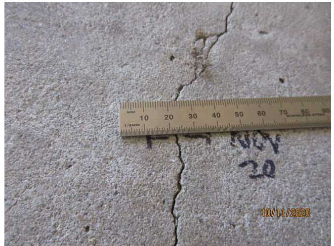
No 1-3_358_Note an estimated 1.0mm cracking width at representative location
