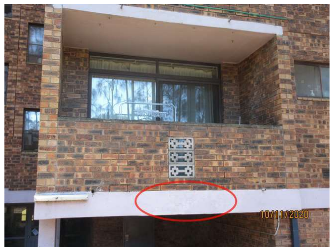
No1_072_Note slight concrete spalling
