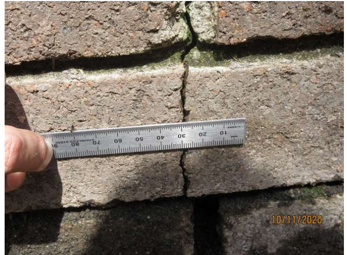
No 5_110_Note an estimated 3.0mm cracking width at representative location
