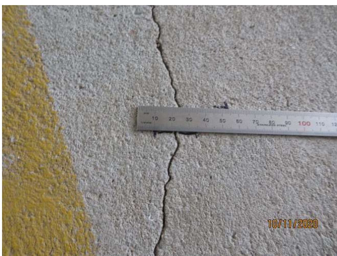
No 5_161_Note an estimated 1.5mm cracking width at representative location
