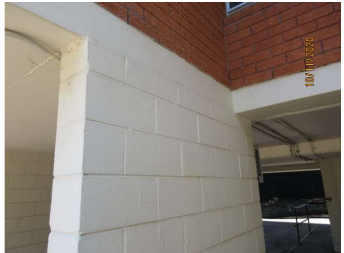
No 1-3_322_Note the cracking damage
