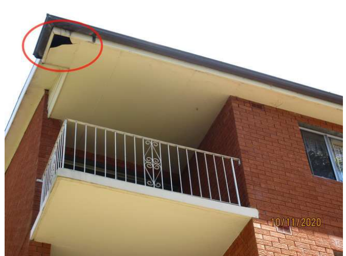
No 1-3_006_Note damaged eave line soffit board
