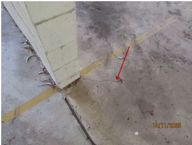
No 1-3_243_Note the cracking damage
