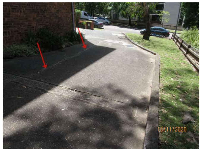
No1_048_Note evident cracking to concrete driveway
