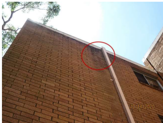
No 3_128_ Note the sign of overflow roof water
