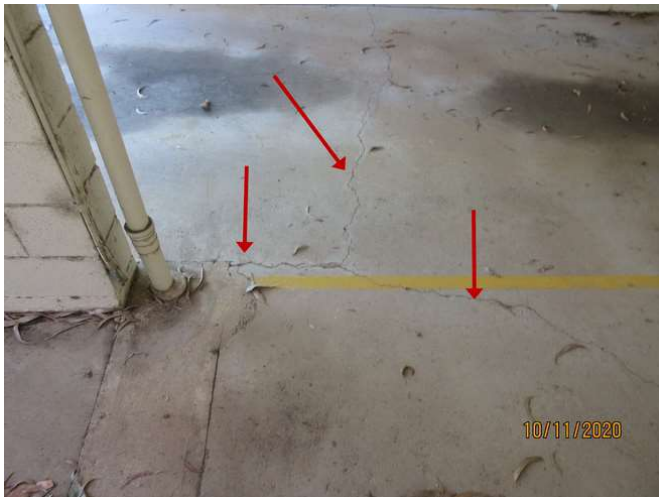
No 1-3_447_Note the cracking damage
