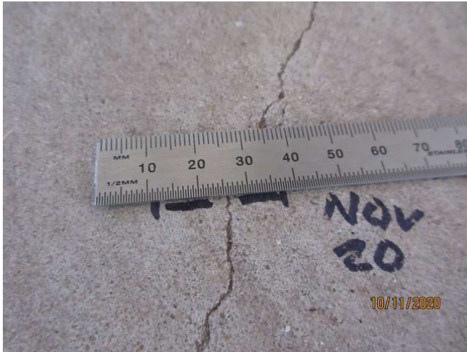
No 1-3_517_Note an estimated 0.5mm cracking width at representative location
