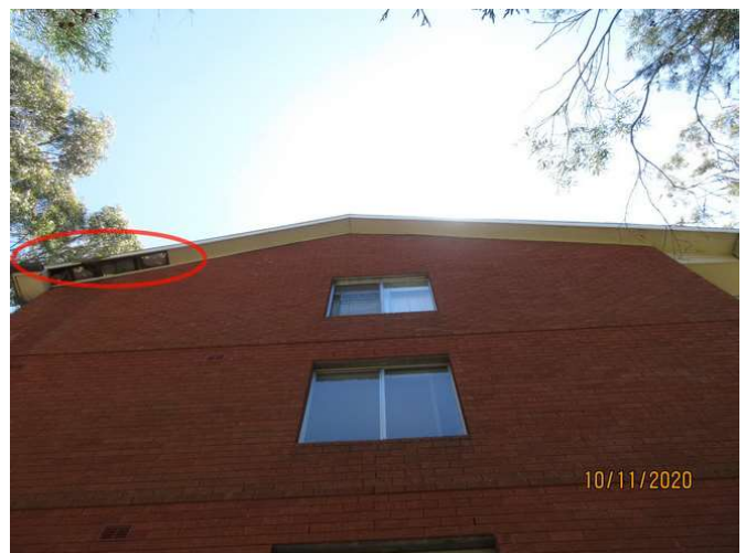
No 1-3_066_Note damaged eave line soffit board
