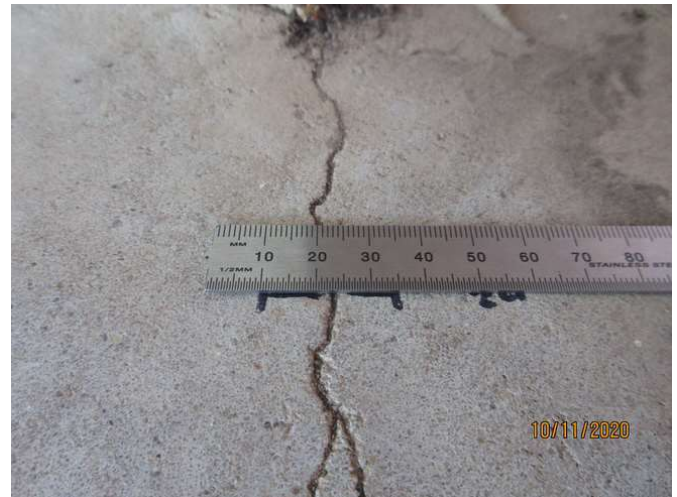
No 1-3_482_Note an estimated 1.0mm cracking width at representative location
