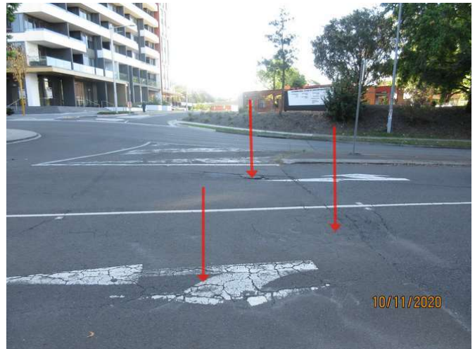
280_Note cracking damage
