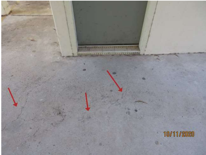
No 1-3_259_Note the cracking damage
