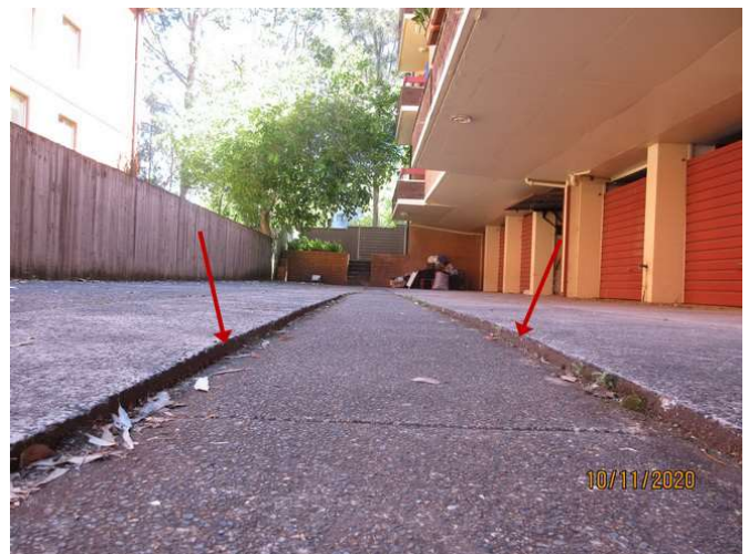
No 155_082_Subsidence along underground drain
