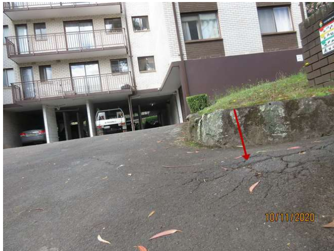
No 7_151_Note distressed road surface
