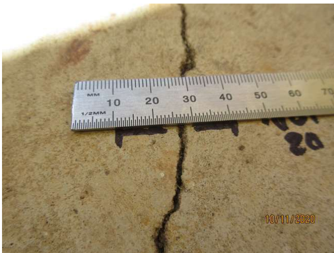
No 1-3_561_Note an estimated 2.0mm cracking width at representative location
