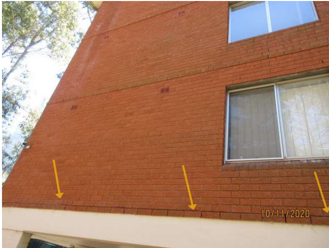
No 1-3_067_Note spalling to course joint lines
