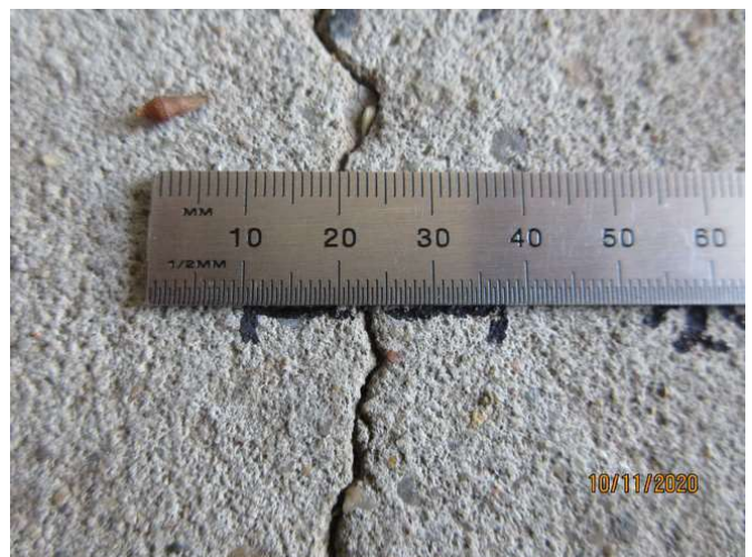
No 5_240_Note an estimated 1.5mm cracking width at representative location
