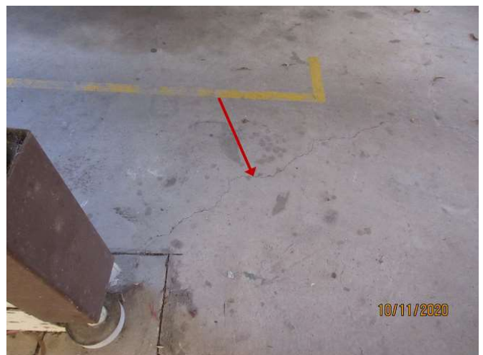
No 1-3_522_Note the cracking damage
