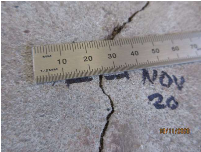
No 1-3_387_Note an estimated 1.5mm cracking width at representative location
