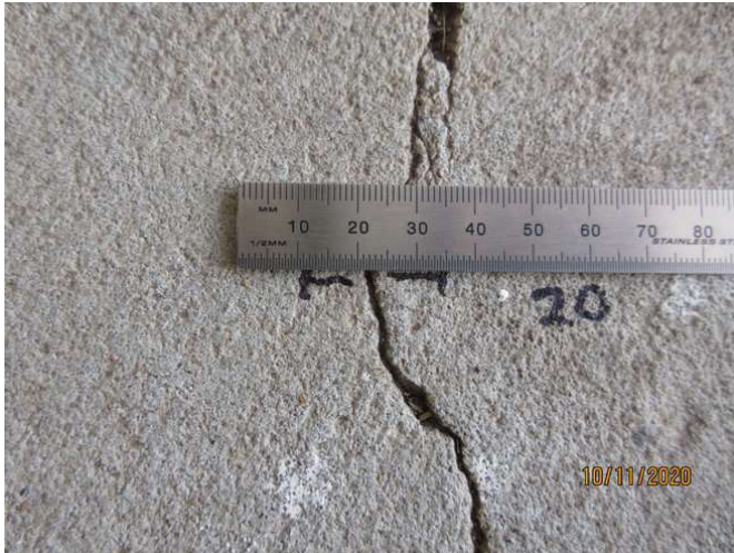
No 5_217_Note an estimated 1.5mm cracking width at representative location
