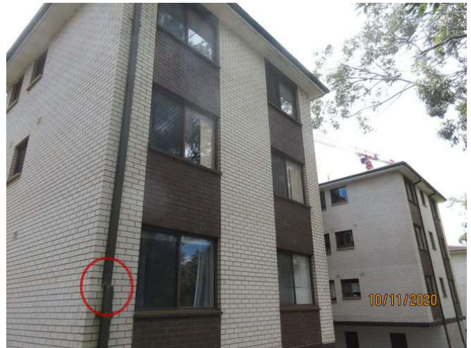
No 5_088_Note dislodged downpipe
