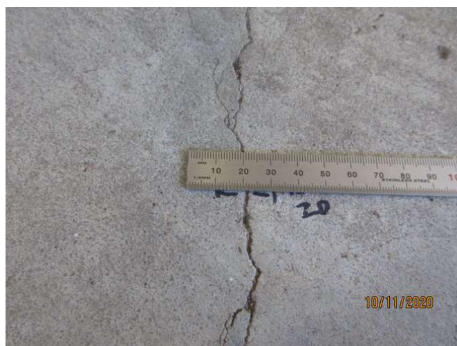
No 1-3_378_Note an estimated 1.0mm cracking width at representative location
