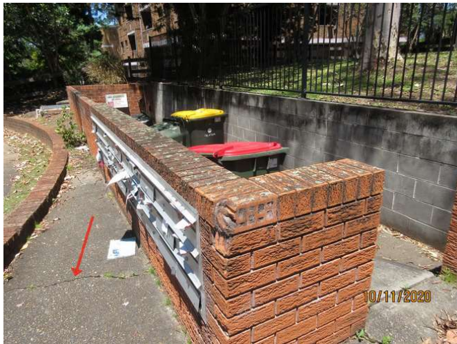
No 1-3_003_Note the cracking damage
