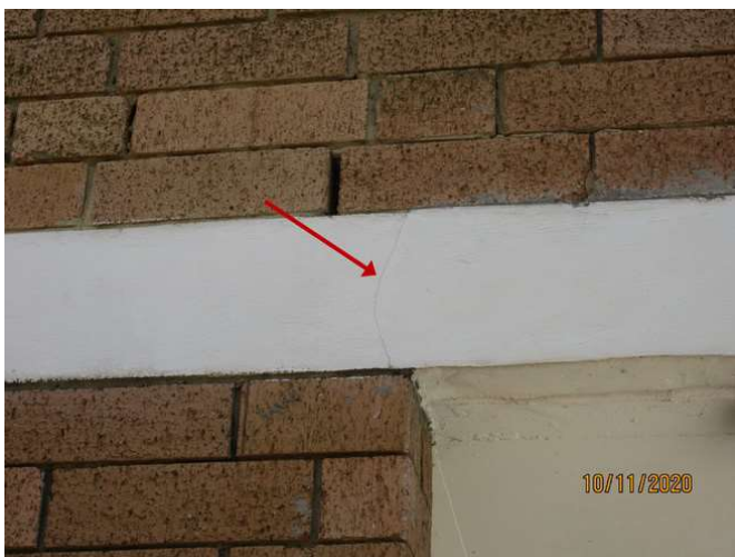
No 3_065_Note the cracking damage
