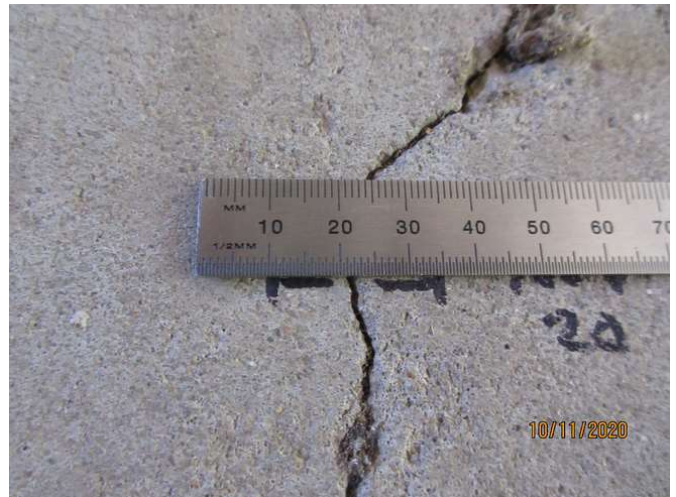
No 1-3_460_Note an estimated 1.5mm cracking width at representative location
