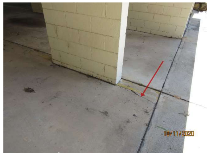
No 1-3_180_Note the cracking damage
