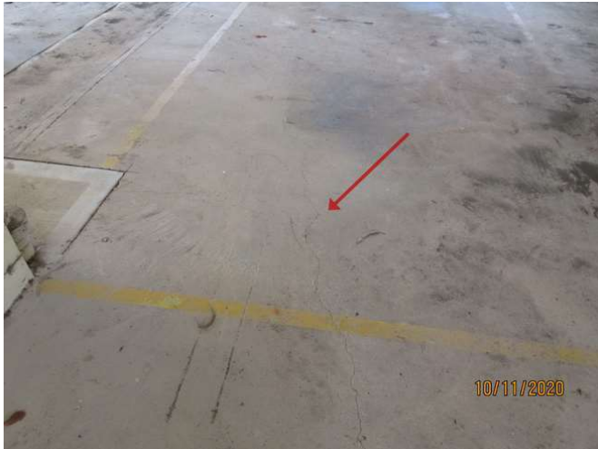
No 1-3_235_Note the cracking damage
