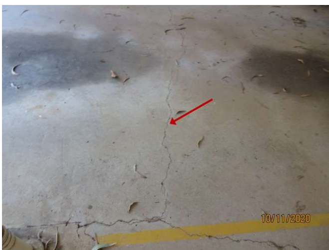
No 1-3_449_Note the cracking damage
