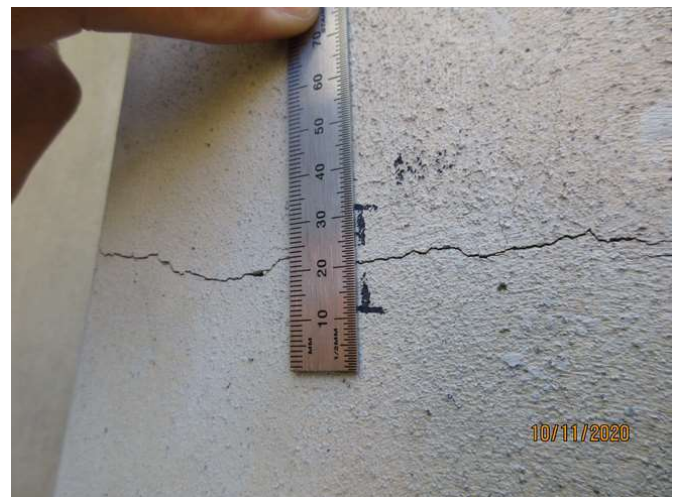
No 155_034_Note an estimated 0.5mm cracking width at representative location
