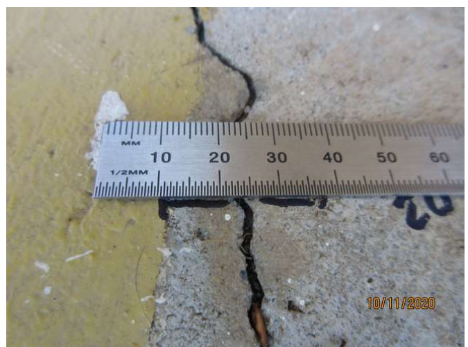
No 1-3_330_Note an estimated 1.5mm cracking width at representative location
