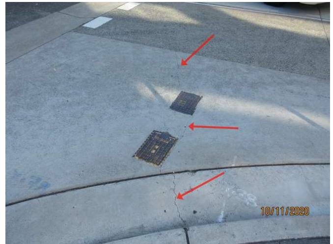
218_Note cracking damage
