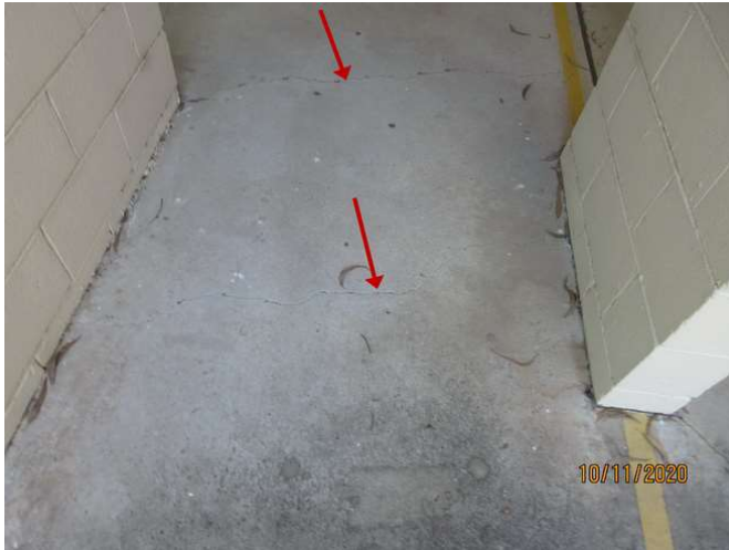
No 1-3_421_Note the cracking damage
