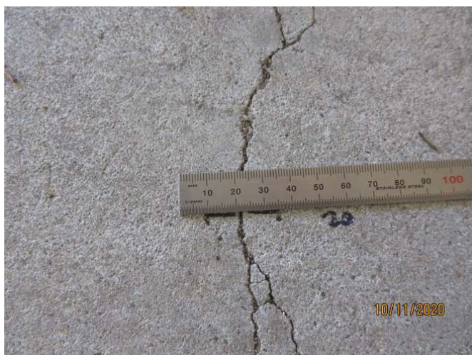
No 1-3_375_Note an estimated 1.0mm cracking width at representative location
