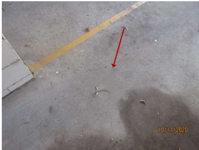
No 1-3_463_Note the cracking damage
