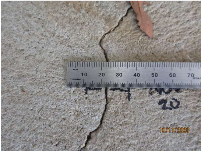
No 5_163_Note an estimated 1.0mm cracking width at representative location
