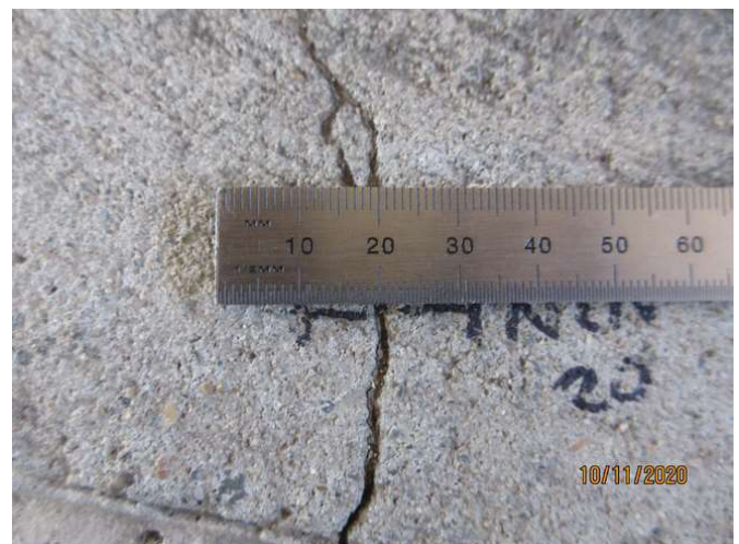
No 1-3_258_Note an estimated 1.5mm cracking width at representative location
