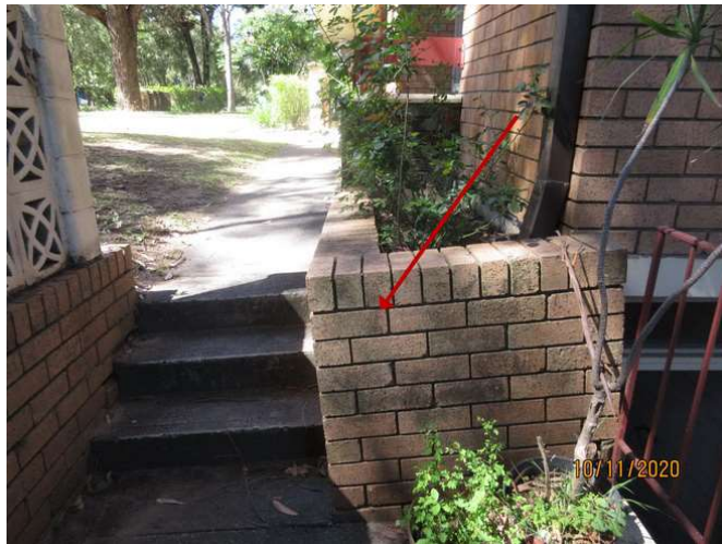
No 155_099_Distressed brick wall
