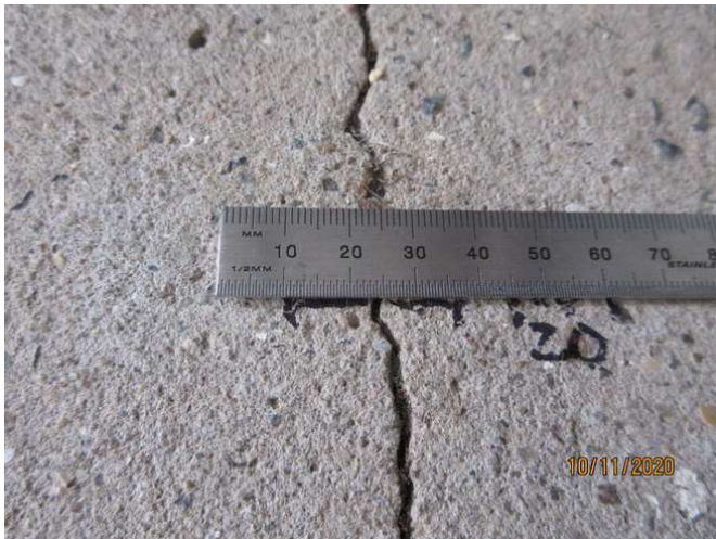
No 7_171_Note an estimated 1.5mm cracking width at representative location
