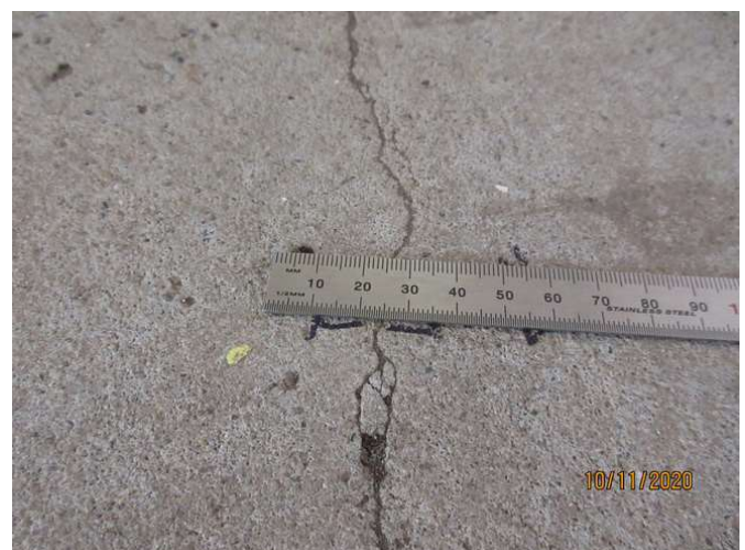
No 1-3_486_Note an estimated 1.0mm cracking width at representative location
