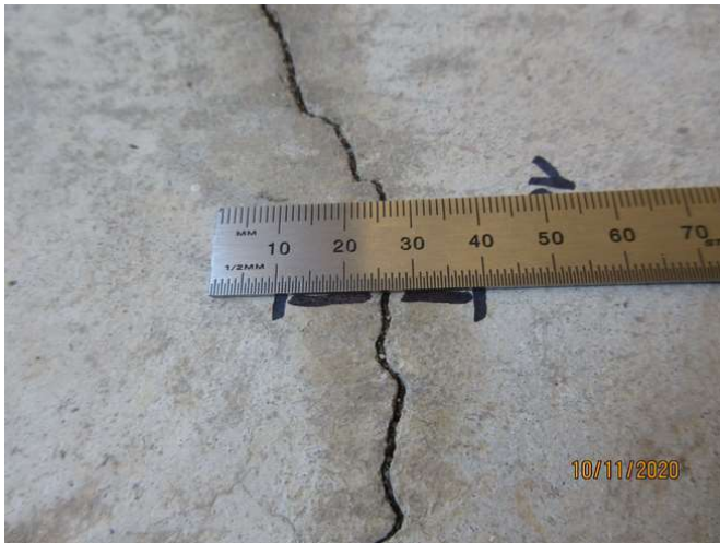
No 1-3_195_Note an estimated 1.0mm cracking width at representative location
