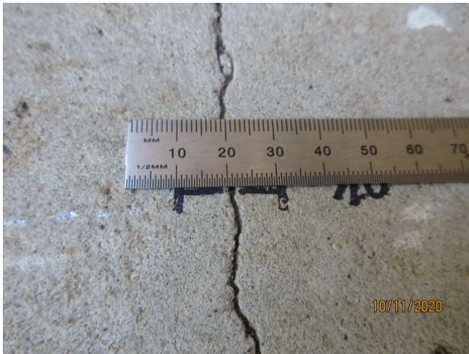
No 1-3_423_Note an estimated 1.5mm cracking width at representative location
