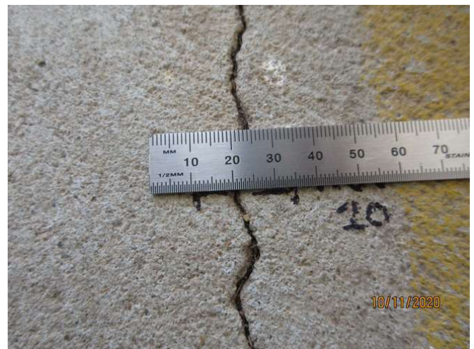
No 5_226_Note an estimated 1.0mm cracking width at representative location
