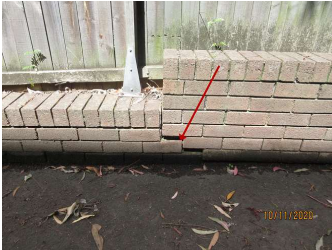
No 5_103_Note distressed retaining boundary wall
