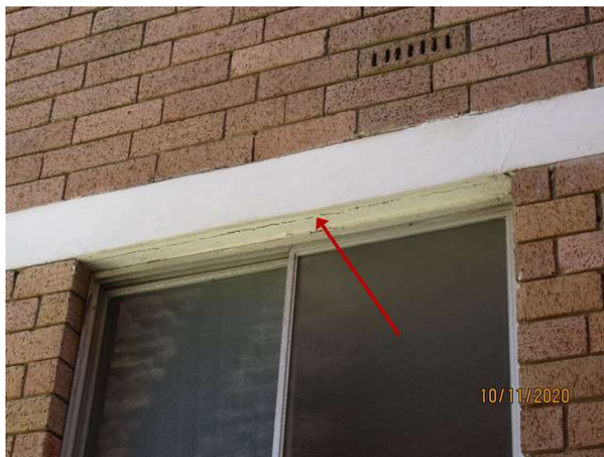
No 3_099_Note the cracking damage
