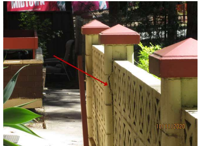
No 155_046_Note the cracking damage
