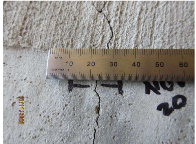
No 1-3_302_Note an estimated 0.5mm cracking width at representative location
