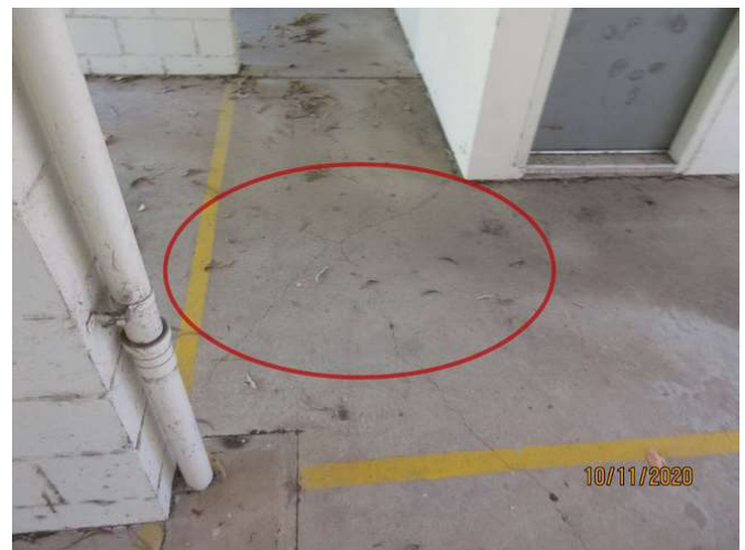
No 1-3_484_Note the cracking damage
