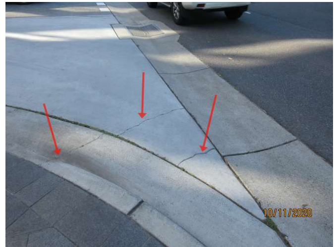
212_Note cracking damage
