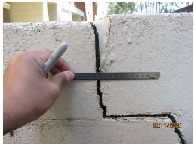
No 1-3_510_Note an estimated 5.5mm cracking width at representative location
