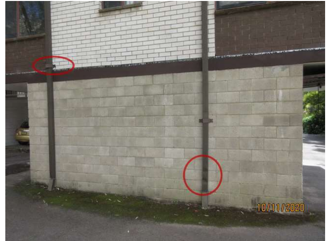
No 5_092_Note loose bracket and impact damage
