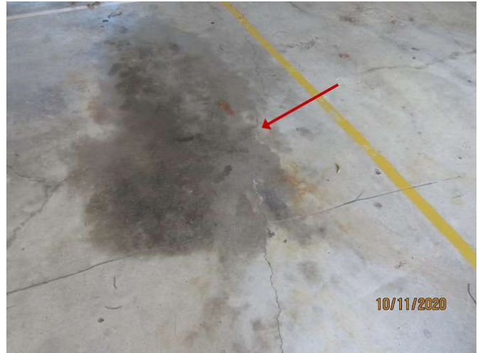
No 1-3_308_Note the cracking damage
