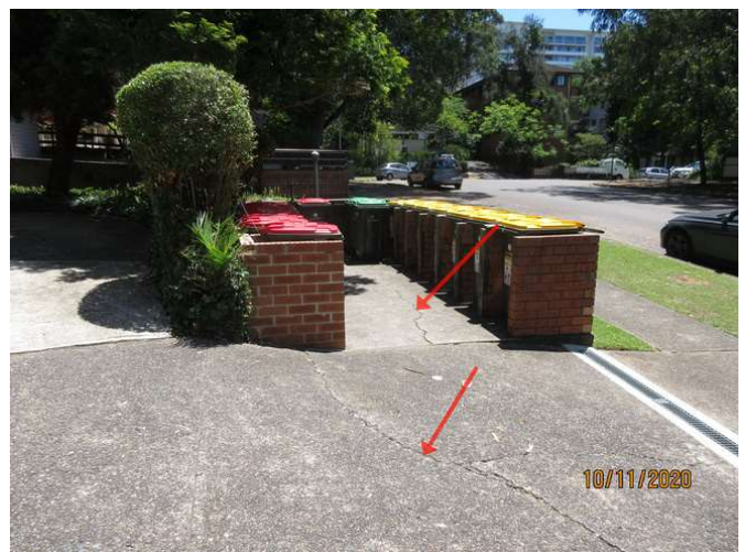
No1_006_Note evident cracking to concrete driveway
