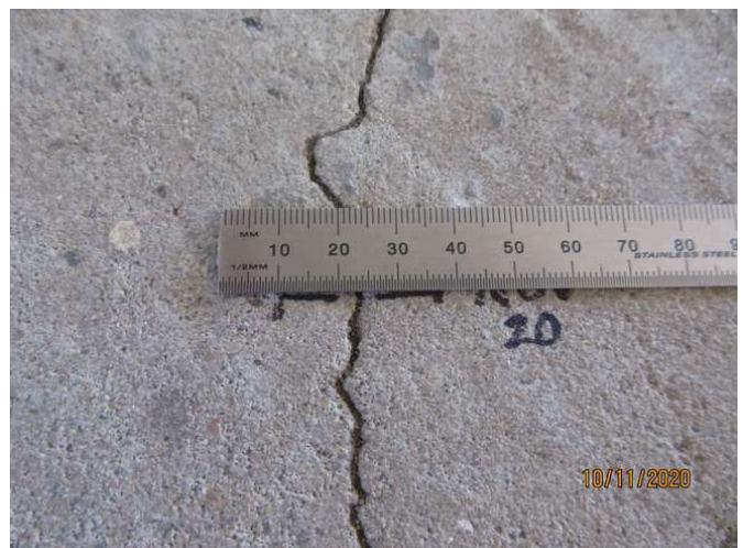
No 1-3_252_Note an estimated 1.0mm cracking width at representative location
