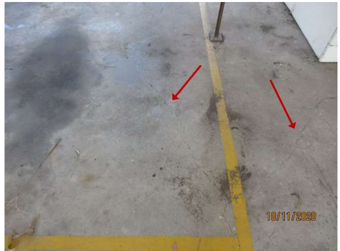
No 1-3_310_Note the cracking damage
