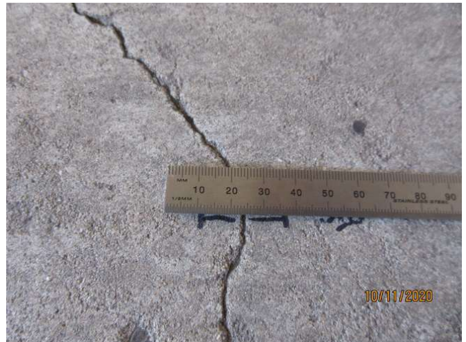
No 1-3_202_Note an estimated 1.5mm cracking width at representative location
