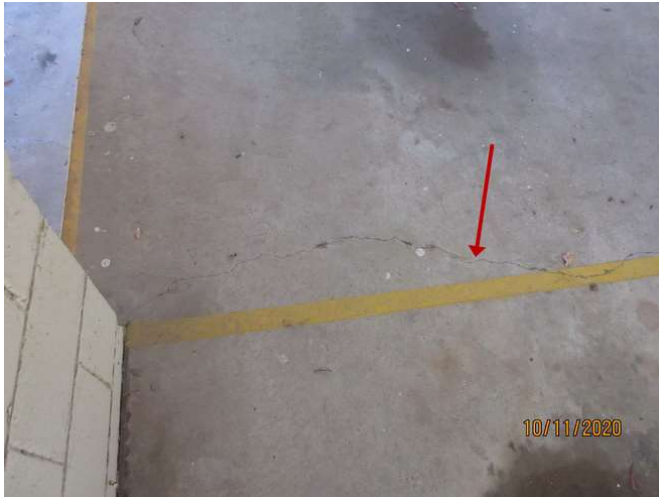
No 1-3_457_Note the cracking damage
