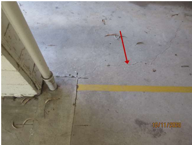
No 1-3_339_Note the cracking damage
