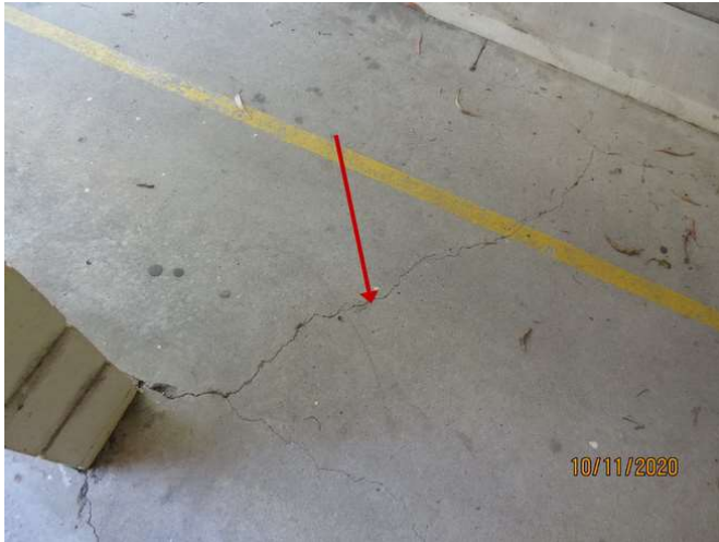
No 1-3_427_Note the cracking damage
