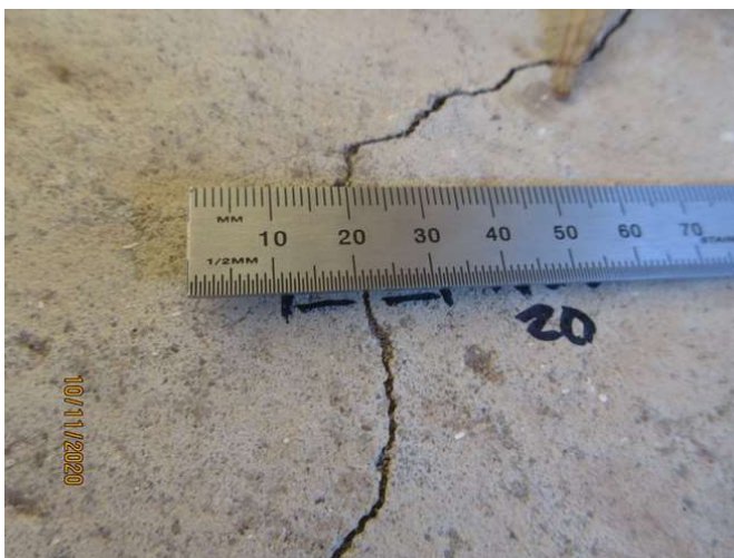
No 1-3_545_Note an estimated 0.75mm cracking width at representative location
