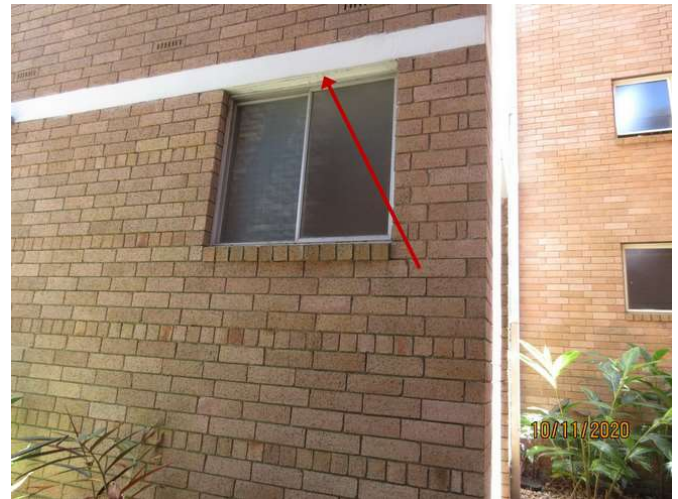
No 3_098_Note the cracking damage
