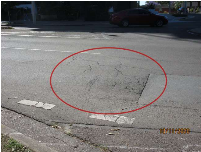
039_Note cracking damage
