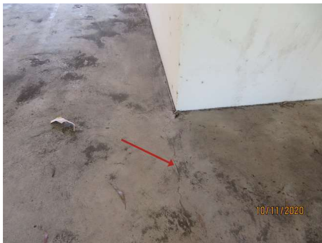
No 1-3_273_Note the cracking damage
