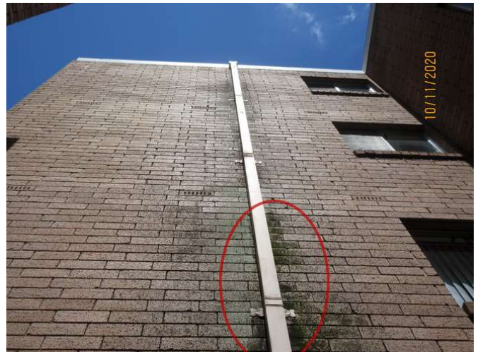
No 3_088_Note the sign of overflow roof water
