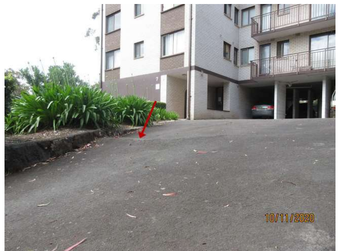
No 7_150_Note distressed road surface
