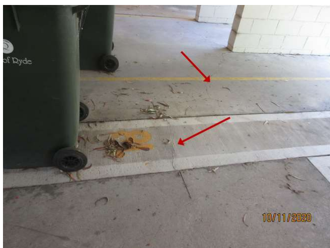
No 1-3_467_Note the cracking damage
