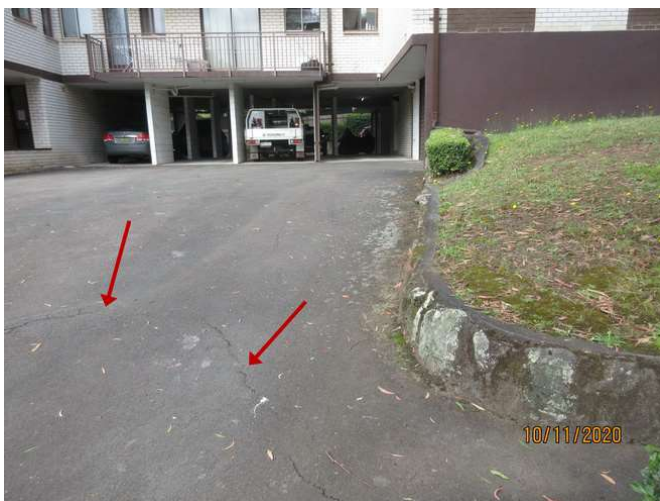
No 7_149_Note distressed road surface
