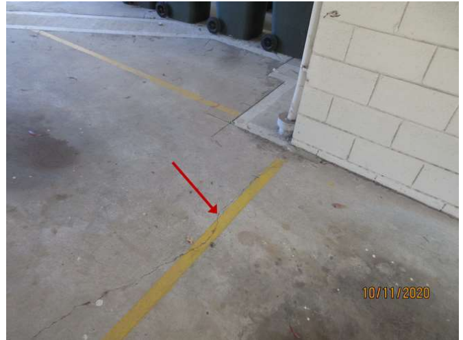
No 1-3_458_Note the cracking damage
