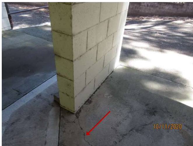
No 1-3_501_Note the cracking damage
