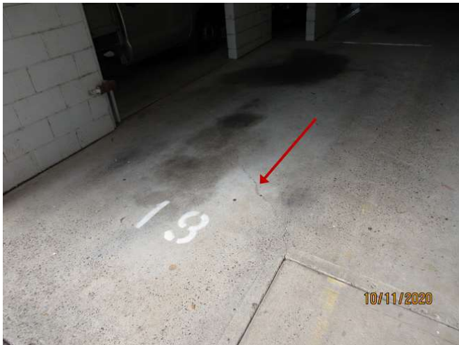
No 7_165_Cracking generally noted to concrete slab
