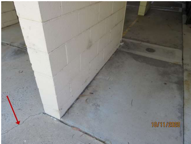
No 1-3_405_Note the cracking damage
