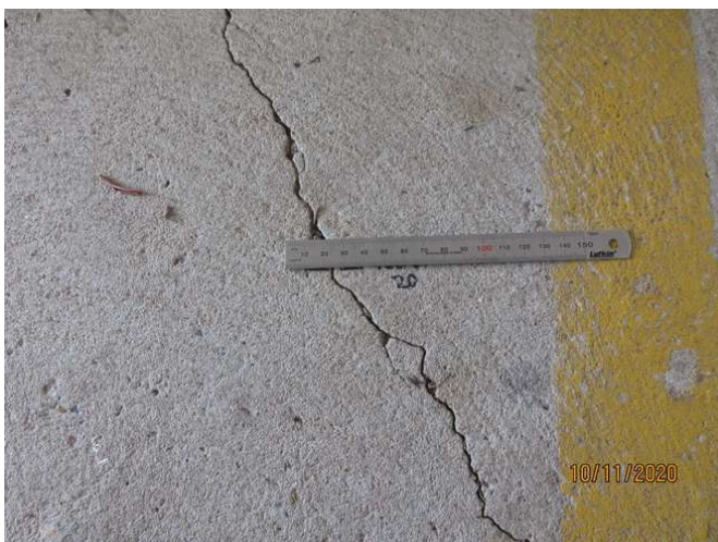
No 5_197_Note an estimated 1.5mm cracking width at representative location
