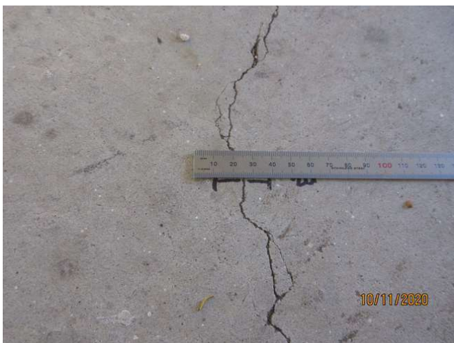
No 1-3_527_Note an estimated 1.0mm cracking width at representative location
