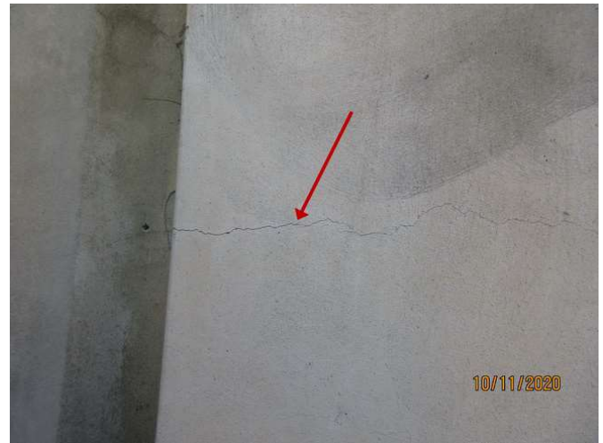
No 155_032_Note the cracking damage
