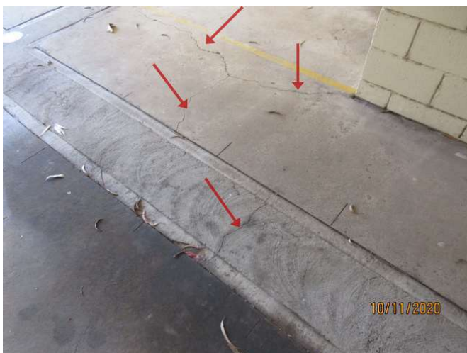
No 1-3_203_Note the cracking damage
