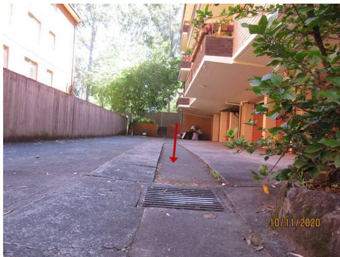
No 155_081_Subsidence along underground drain
