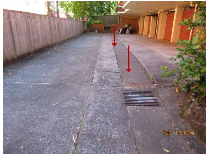
No 155_080_Subsidence along underground drain
