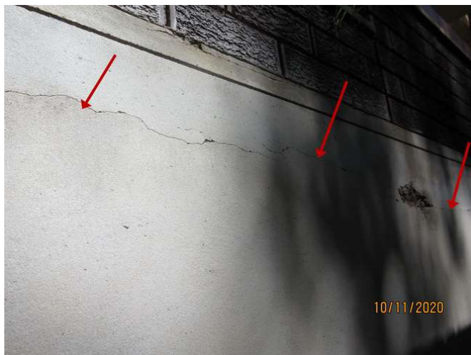
No 155_039_Note the cracking damage
