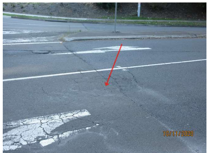
282_Note cracking damage
