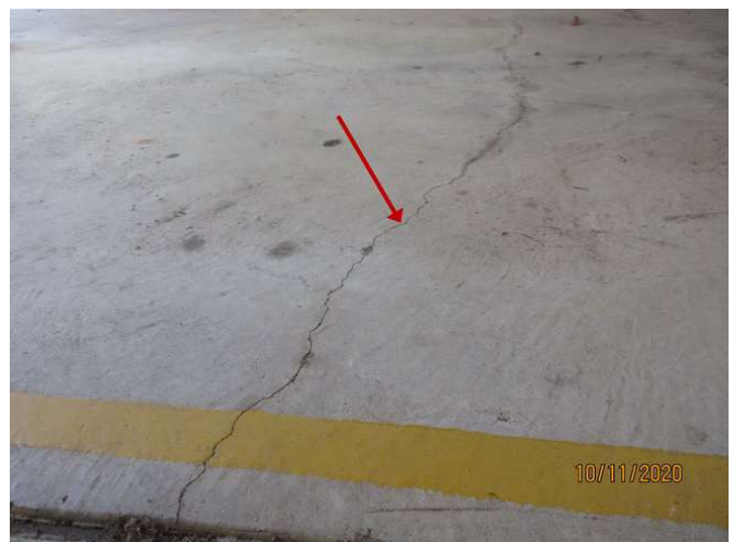
No 1-3_348_Note the cracking damage
