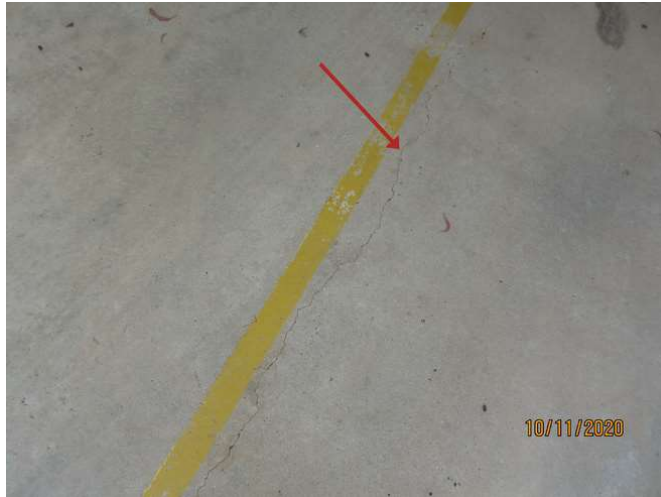
No 1-3_175_Note the cracking damage
