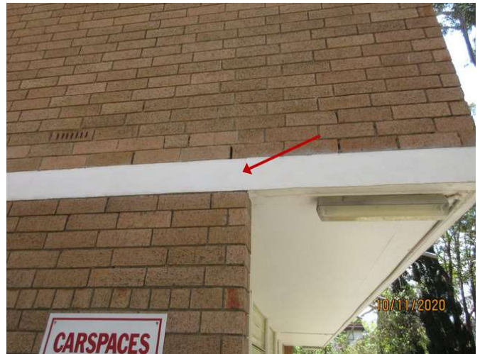
No 3_064_Note the cracking damage
