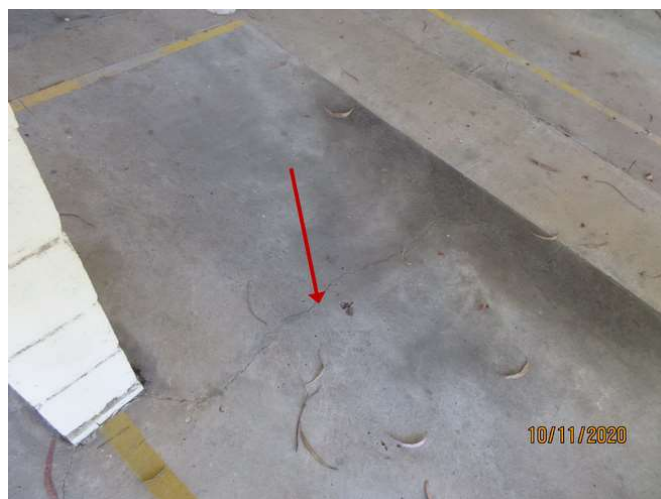
No 1-3_376_Note the cracking damage
