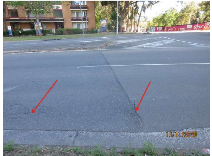
182_Note cracking damage
