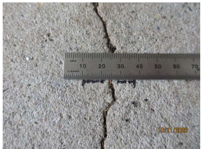
No 7_168_Note an estimated 1.5mm cracking width at representative location
