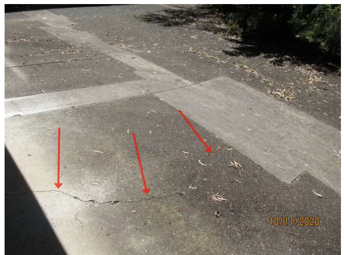
No 1-3_054_Note the cracking damage
