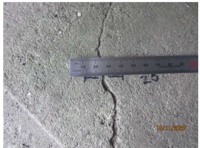
No 7_244_Note an estimated 1.0mm cracking width at representative location
