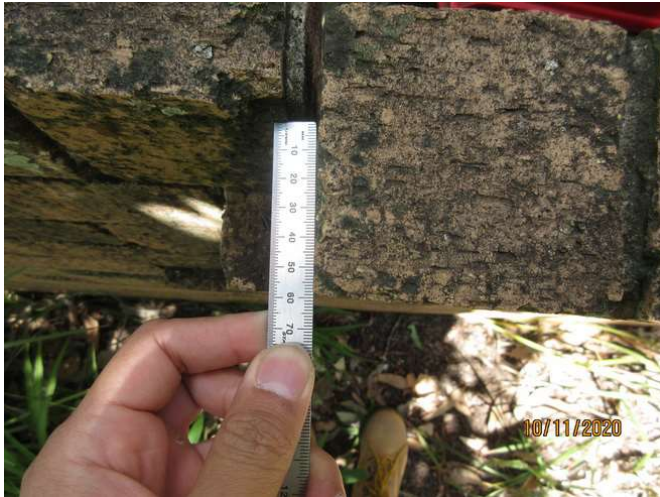
No 3_007_Note an estimated 59.0mm displacement on top
