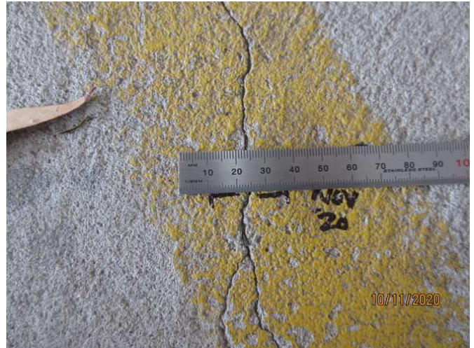
No 5_194_Note an estimated 2.0mm cracking width at representative location
