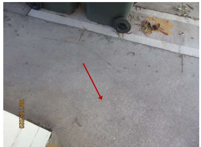
No 1-3_466_Note the cracking damage
