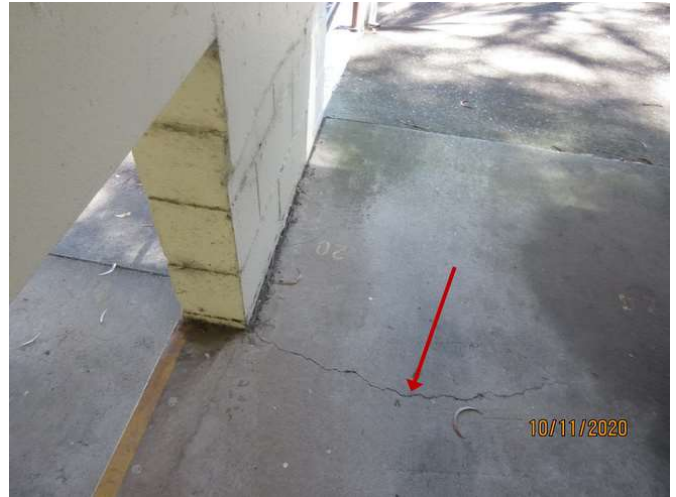
No 1-3_494_Note the cracking damage
