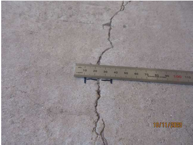
No 1-3_217_Note an estimated 3.0mm cracking width at representative location
