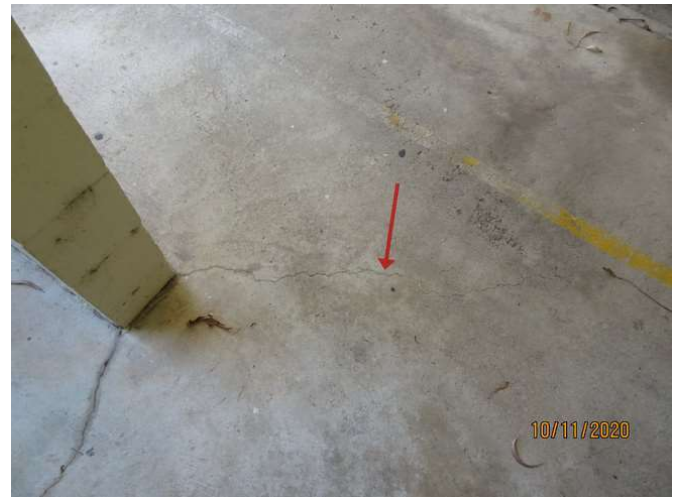
No 1-3_196_Note the cracking damage
