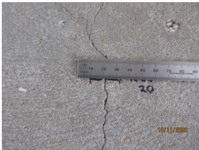
No 5_153_Note an estimated 1.0mm cracking width at representative location
