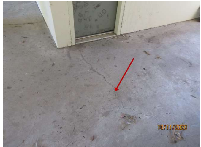
No 1-3_382_Note the cracking damage
