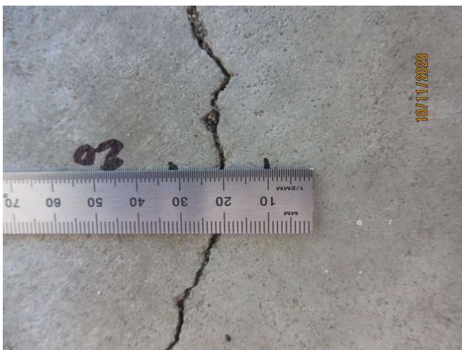
No 1-3_317_Note an estimated 2.0mm cracking width at representative location
