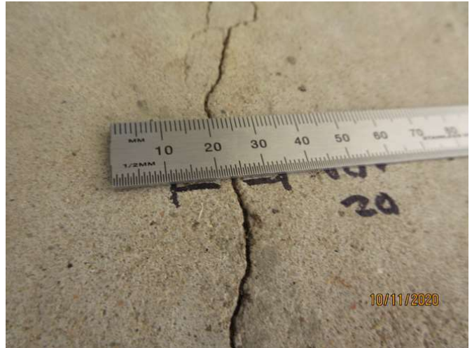
No 1-3_554_Note an estimated 1.0mm cracking width at representative location
