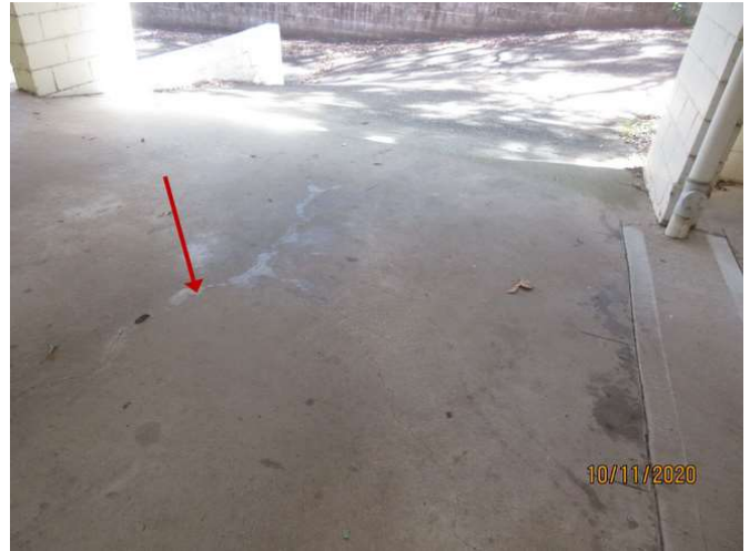
No 1-3_524_Note the cracking damage
