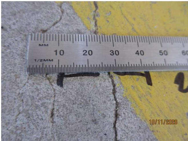
No 1-3_381_Note an estimated 1.0mm cracking width at representative location
