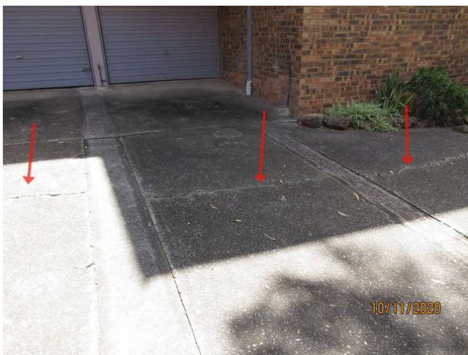
No1_047_Note evident cracking to concrete driveway
