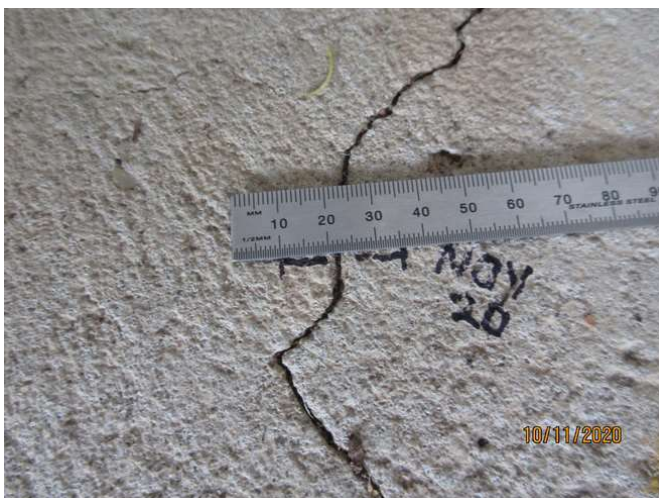
No 5_173_Note an estimated 1.0mm cracking width at representative location
