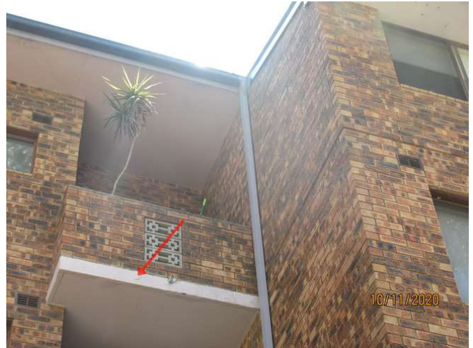
No1_038_Note slight concrete spalling
