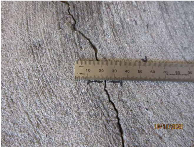
No 1-3_205_Note an estimated 1.5mm cracking width at representative location
