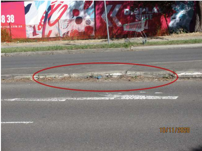
154_Note cracking to medium strip
