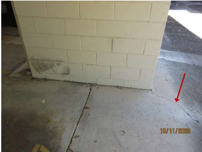
No 1-3_403_Note the cracking damage
