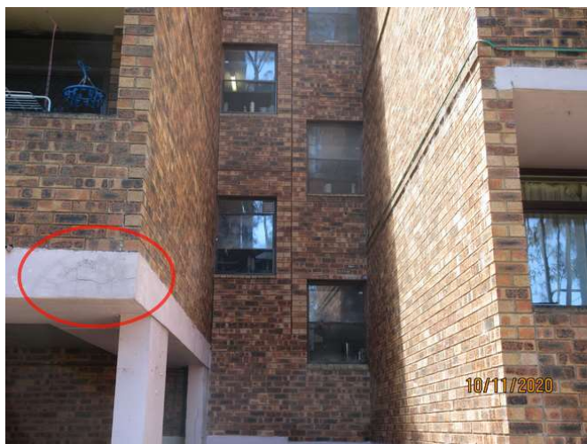
No1_065_Note slight concrete spalling
