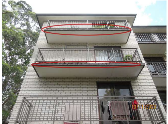
No 5_032_Note mould build up and dampness damage
