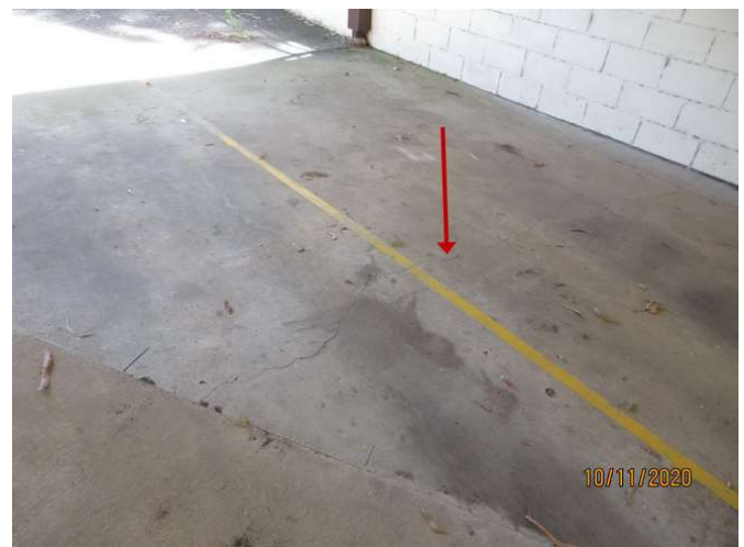
No 1-3_384_Note the cracking damage
