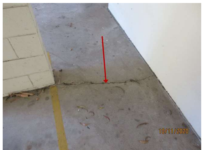
No 1-3_366_Note the cracking damage
