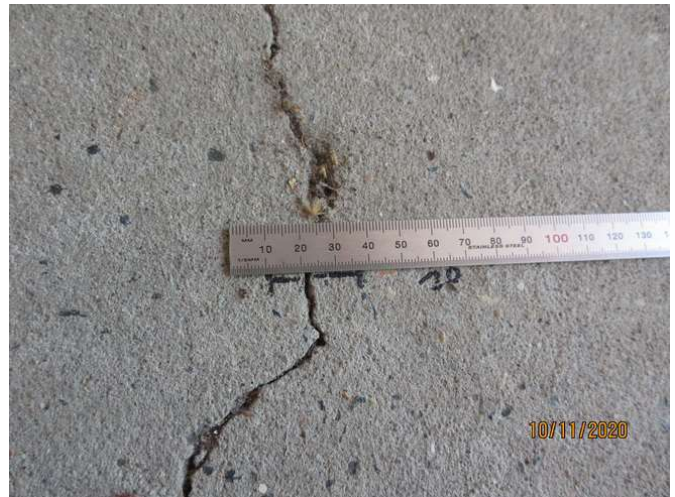
No 1-3_430_Note an estimated 2.0mm cracking width at representative location
