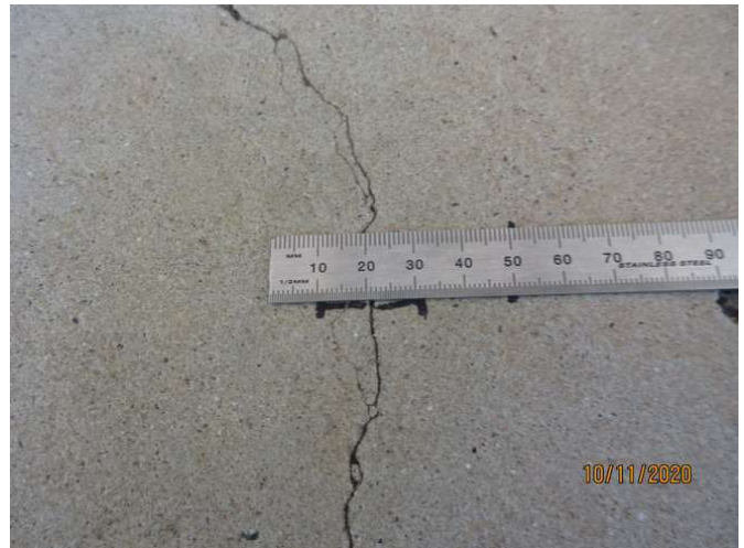
No 1-3_172_Note 1.0mm cracking width at representative location
