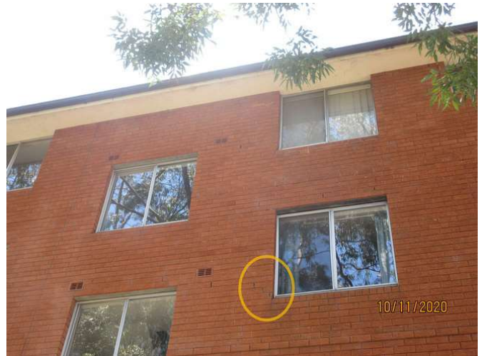
No 1-3_086_Note the cracking damage
