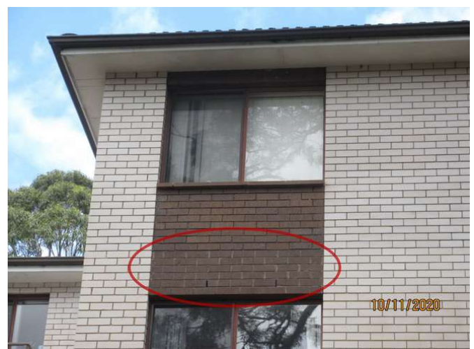
No 5_024_Note re-addressing to course joints
