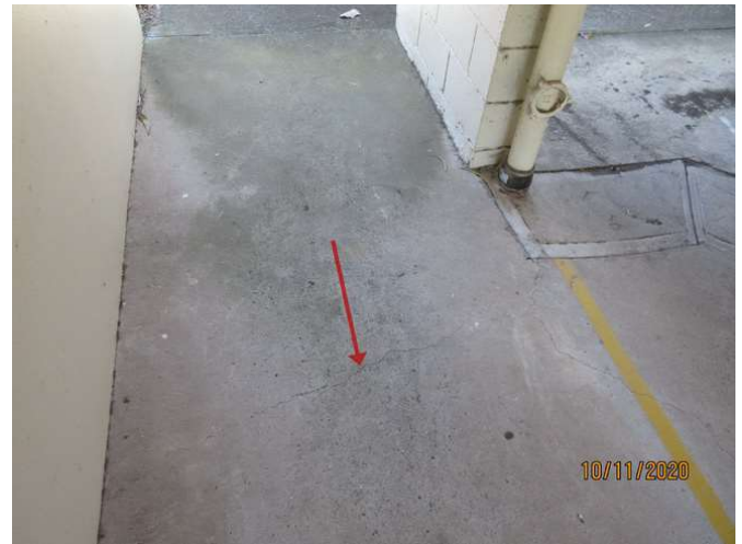
No 1-3_262_Note the cracking damage
