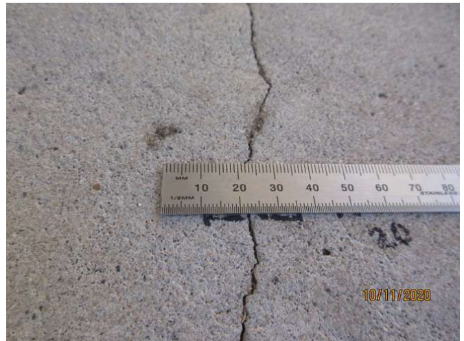
No 1-3_592_Note an estimated 0.5mm cracking width at representative location
