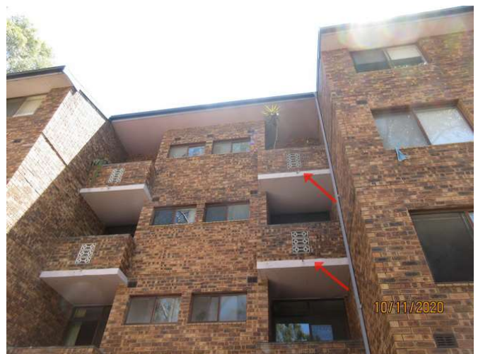
No1_024_Note slight concrete spalling
