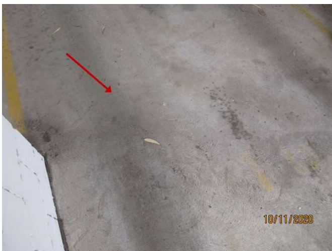
No 5_119_Note cracking generally noted to concrete slab
