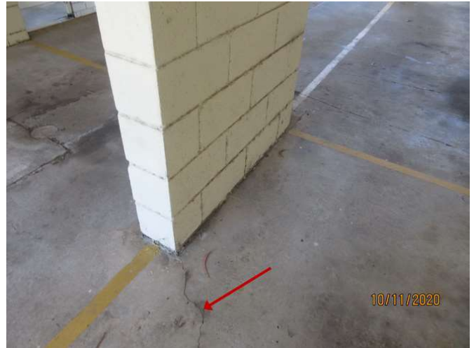
No 1-3_356_Note the cracking damage
