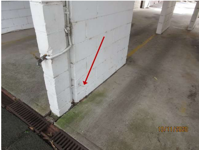
No 5_115_Note the cracking damage
