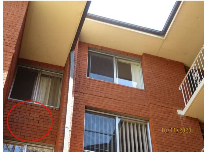
No 1-3_032_Note spalling to course joint lines
