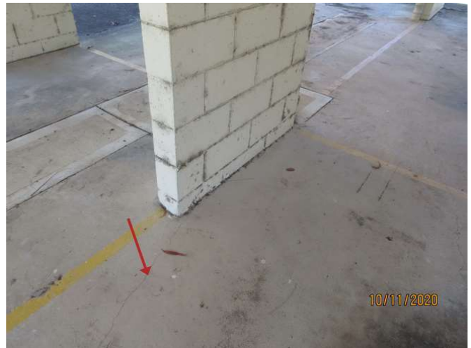
No 1-3_232_Note the cracking damage
