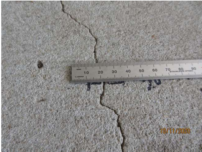
No 5_205_Note an estimated 1.5mm cracking width at representative location
