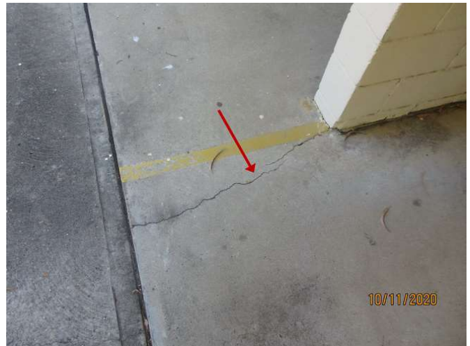
No 1-3_328_Note the cracking damage
