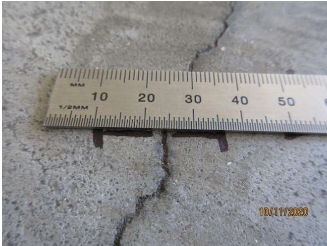
No 1-3_361_Note an estimated 1.0mm cracking width at representative location
