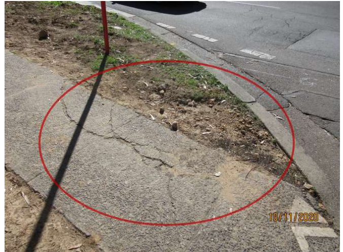
038_Note cracking damage to footpath
