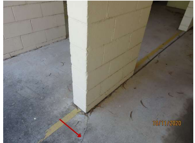
No 1-3_434_Note the cracking damage
