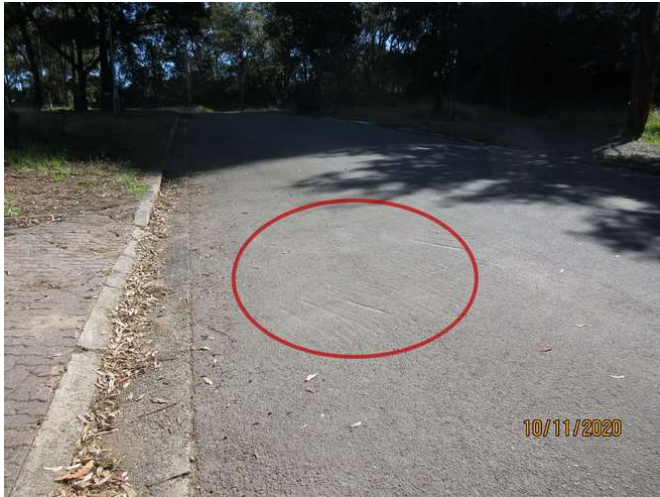
007_Note slight surface cracking and scratch damage
