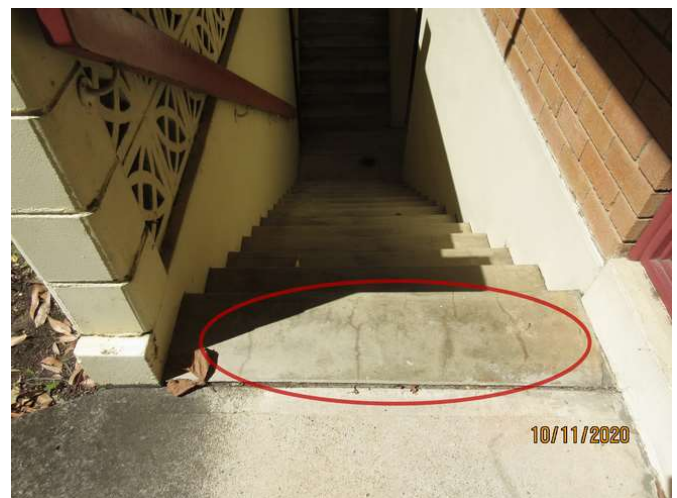
No 155_048_Note the cracking damage
