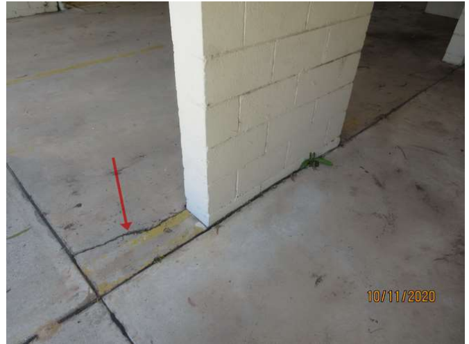
No 1-3_182_Note the cracking damage
