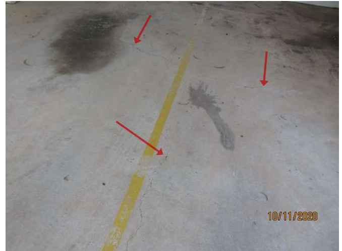
No 1-3_176_Note the cracking damage
