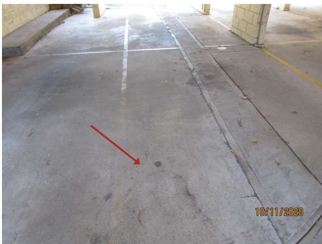
No 1-3_269_Note the cracking damage
