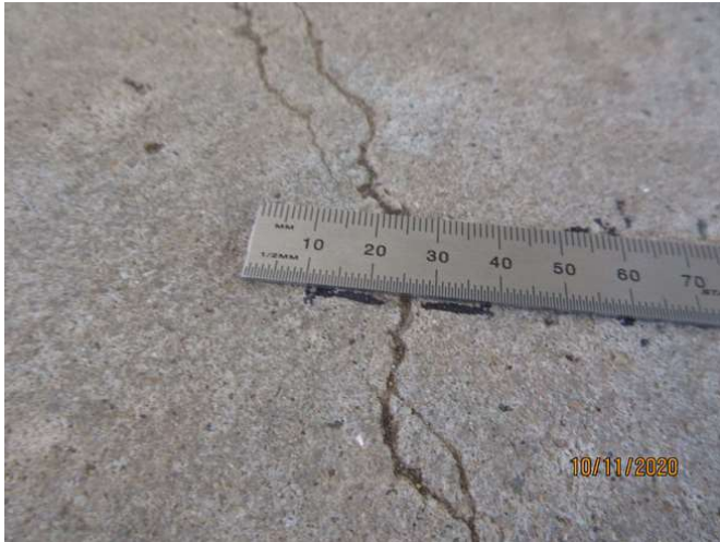
No 1-3_493_Note an estimated 1.5mm cracking width at representative location
