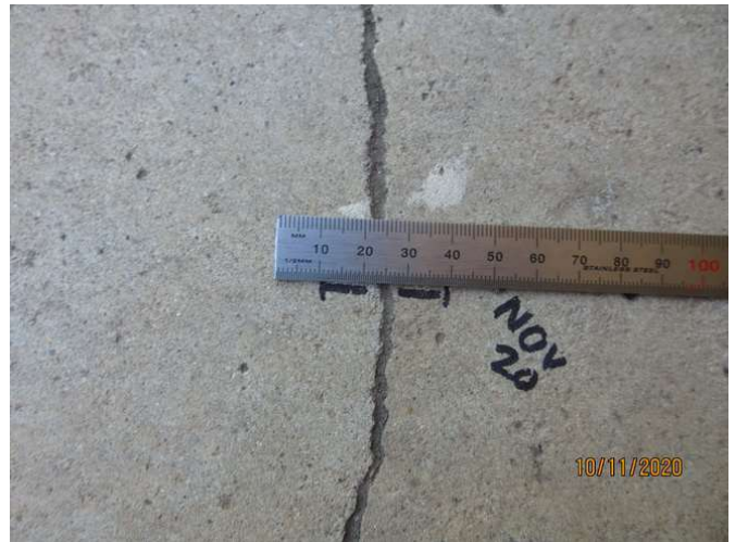
No 1-3_418_Note an estimated 3.5mm cracking width at representative location
