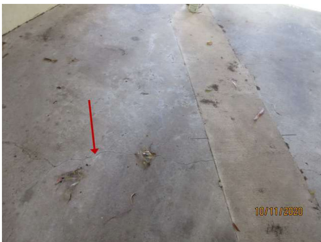
No 1-3_383_Note the cracking damage
