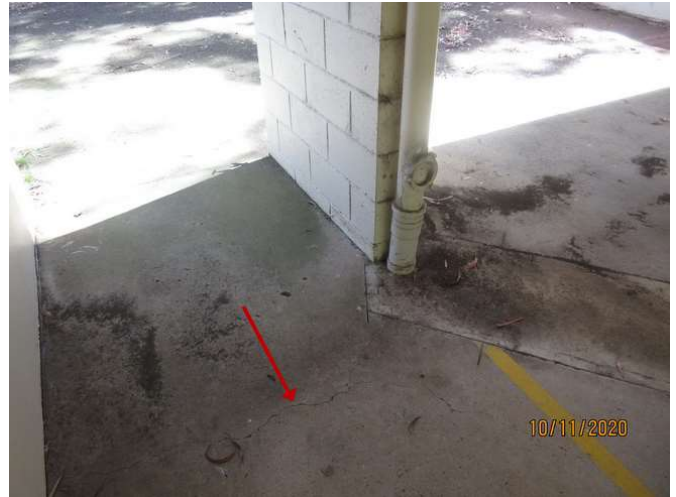
No 1-3_488_Note the cracking damage
