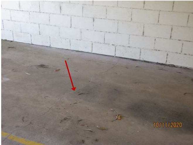
No 1-3_385_Note the cracking damage
