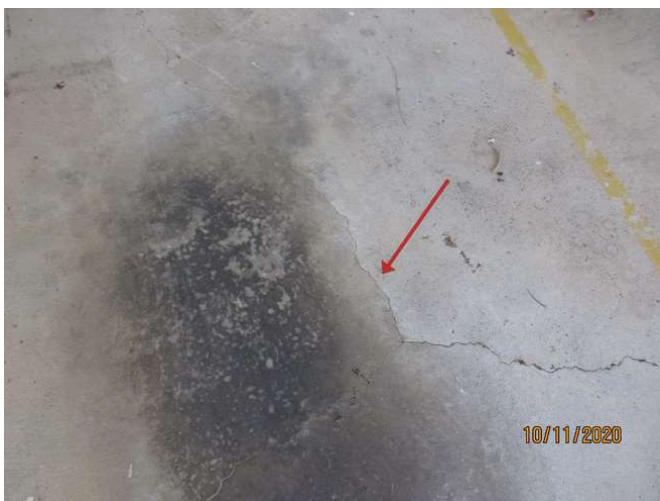
No 1-3_233_Note the cracking damage
