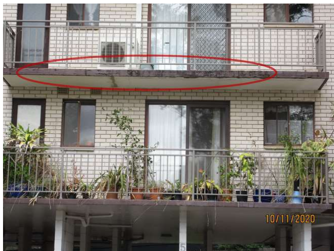
No 5_021_Note mould build up and dampness damage
