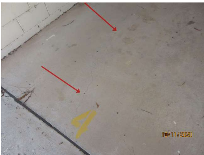
No 1-3_167_Note the cracking damage
