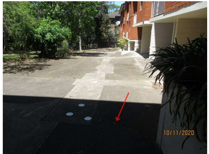
No 1-3_052_Note the cracking damage
