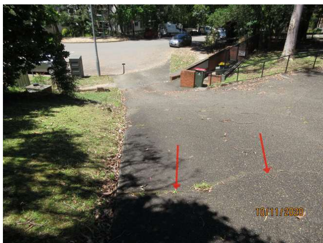
No 1-3_057_Note the cracking damage
