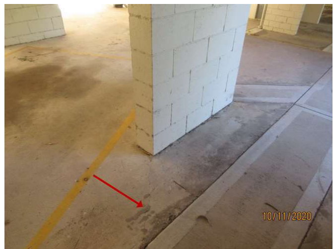
No 1-3_540_Note the cracking damage
