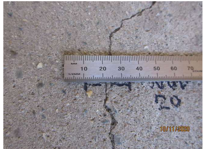
No 1-3_272_Note an estimated 1.0mm cracking width at representative location
