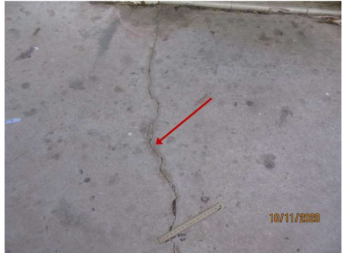
No 1-3_386_Note the cracking damage
