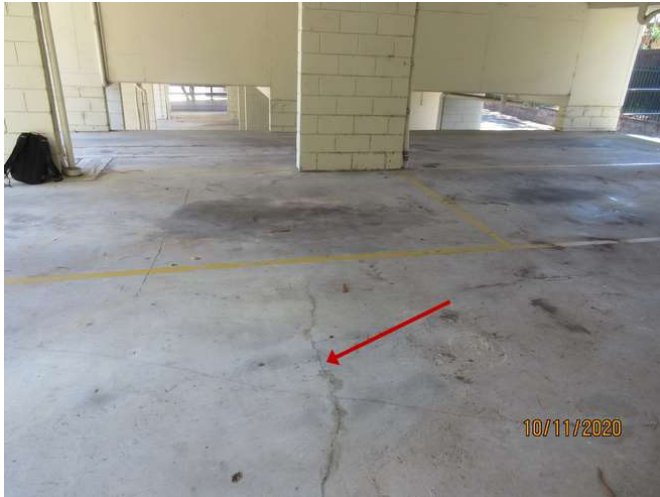
No 1-3_343_Note the cracking damage
