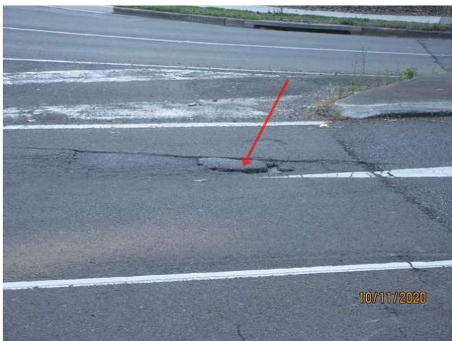
281_Note pothole next to roundabout
