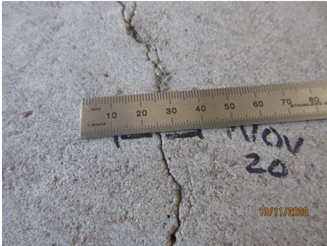
No 1-3_475_Note an estimated 1.0mm cracking width at representative location
