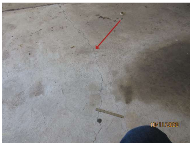
No 1-3_213_Note the cracking damage
