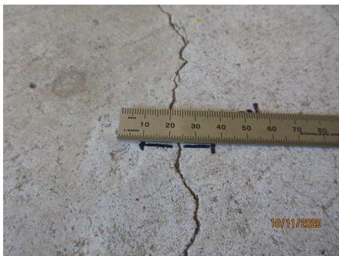
No 1-3_214_Note an estimated 1.0mm cracking width at representative location
