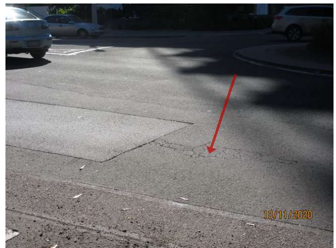
034_Note cracking damage
