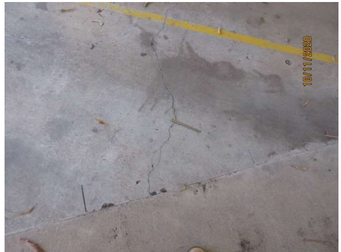
No 1-3_388_Note the cracking damage
