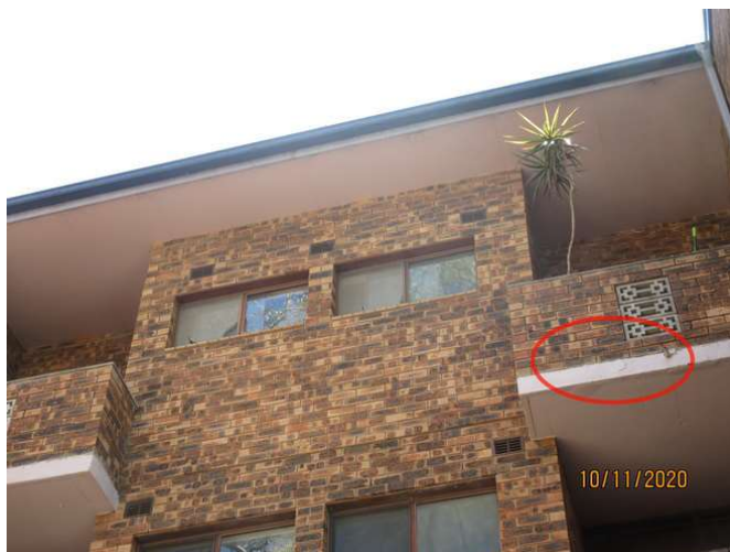
No1_035_Note slight concrete spalling
