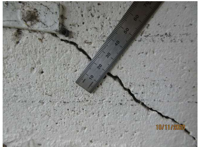
No 5_118_Note an estimated 2.0mm cracking width at representative location
