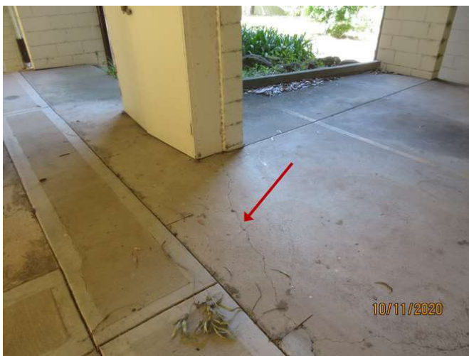
No 1-3_533_Note the cracking damage
