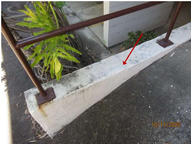
No 1-3_399_Note the cracking damage
