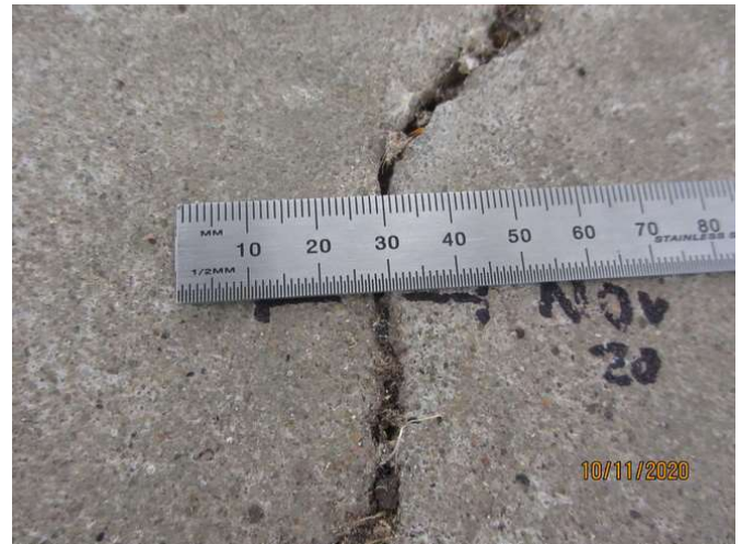
No 1-3_368_Note an estimated 2.0mm cracking width at representative location
