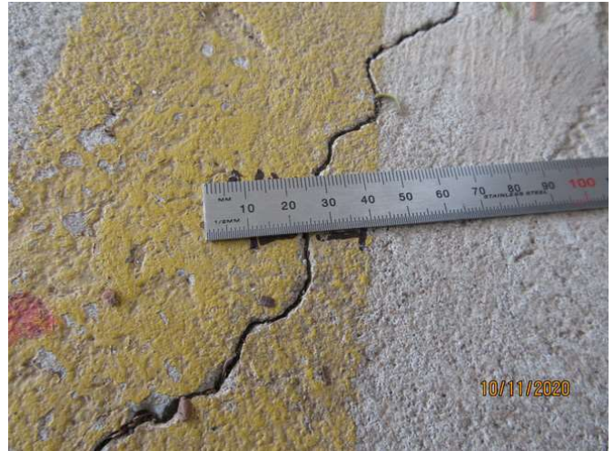
No 5_182_Note an estimated 1.5mm cracking width at representative location
