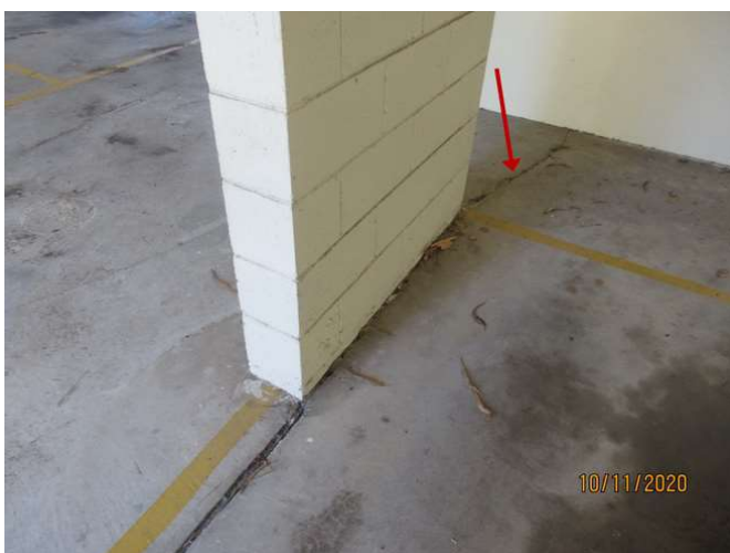
No 1-3_365_Note the cracking damage
