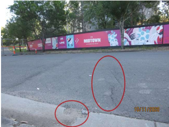
055_Note slight surface cracking and scratch damage
