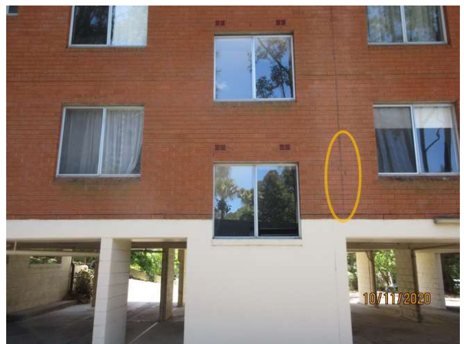
No 1-3_084_Note the cracking damage
