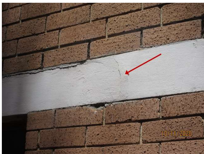
No 3_123_Note the cracking damage
