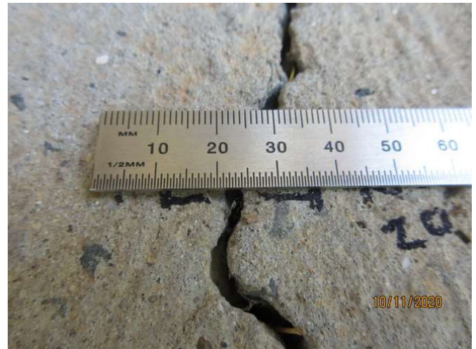
No 1-3_410_Note an estimated 3.0mm cracking width at representative location
