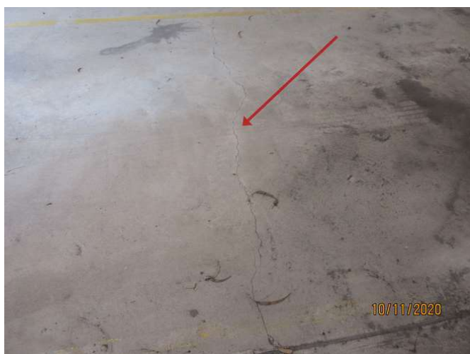
No 1-3_215_Note the cracking damage
