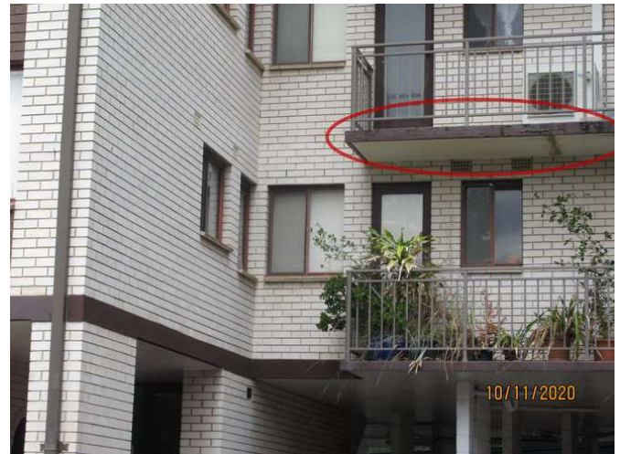
No 5_020_Note mould build up and dampness damage
