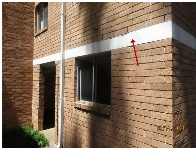
No 3_122_Note the cracking damage
