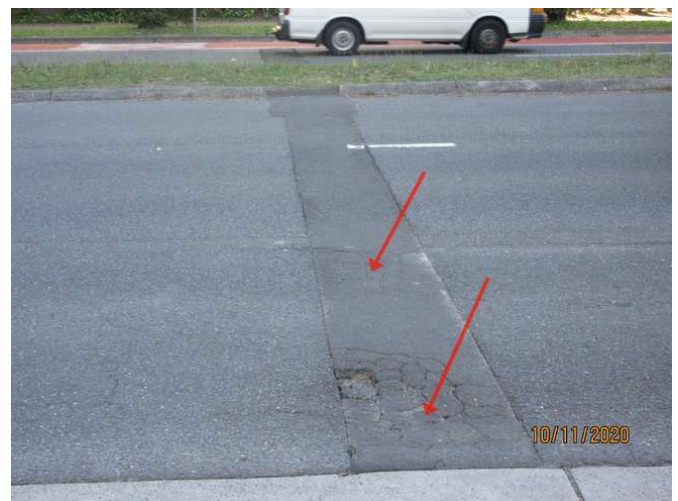
216_Note cracking damage
