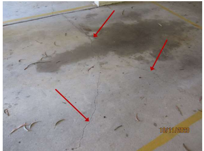
No 1-3_340_Note the cracking damage
