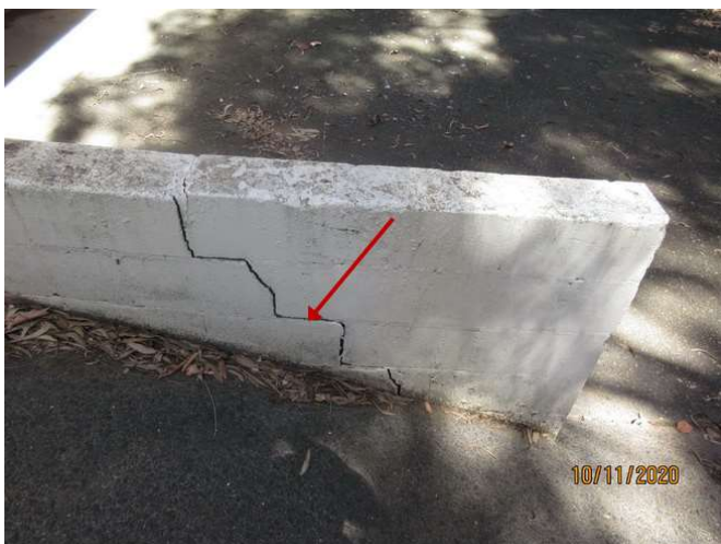
No 1-3_509_Note structual distress to block wall
