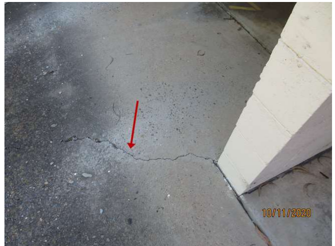
No 1-3_406_Note the cracking damage
