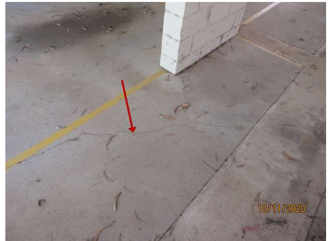
No 1-3_448_Note the cracking damage
