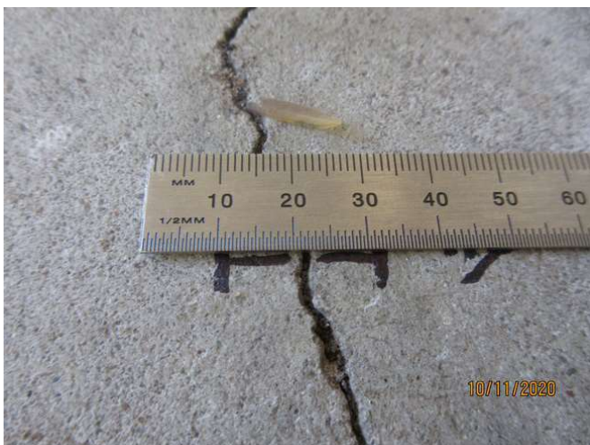
No 1-3_347_Note an estimated 1.0mm cracking width at representative location
