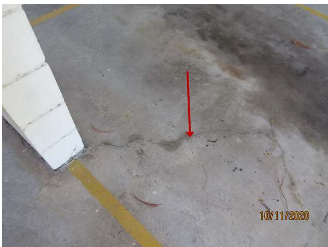
No 1-3_359_Note the cracking damage
