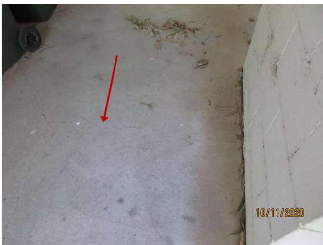
No 1-3_473_Note the cracking damage
