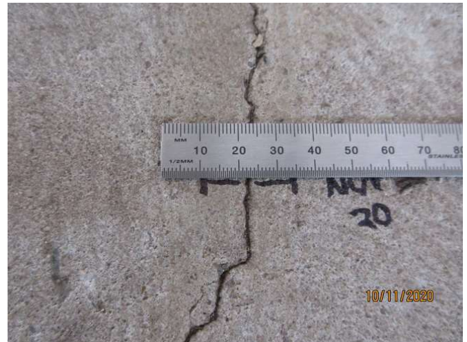
No 5_190_Note an estimated 1.0mm cracking width at representative location
