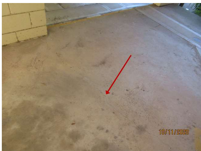
No 1-3_569_Note the cracking damage
