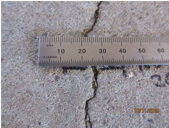
No 1-3_255_Note an estimated 2.0mm cracking width at representative location
