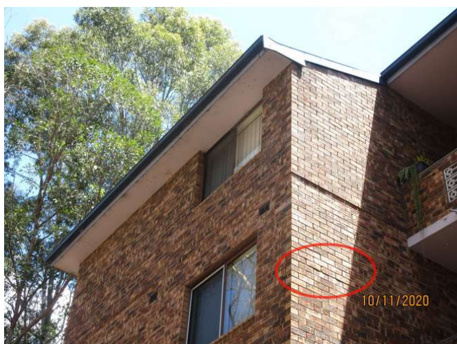
No1_029_Note protruding wall bricks
