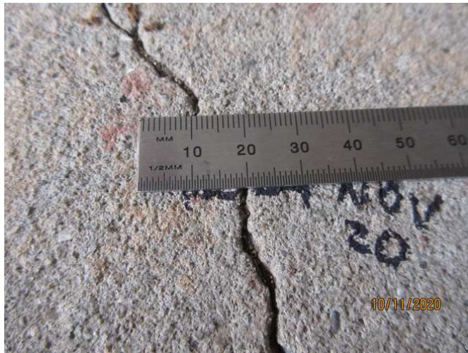
No 7_205_Note an estimated 2.0mm cracking width at representative location
