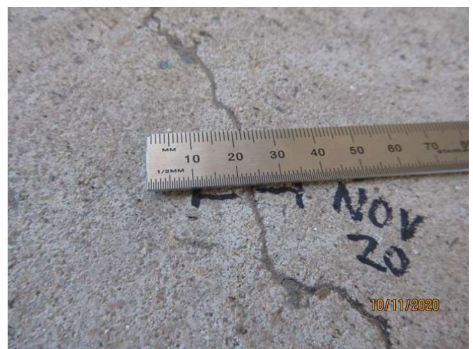
No 1-3_264_Note an estimated 1.5mm cracking width at representative location
