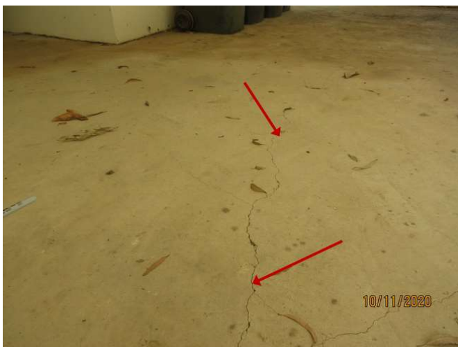
No 1-3_557_Note the cracking damage
