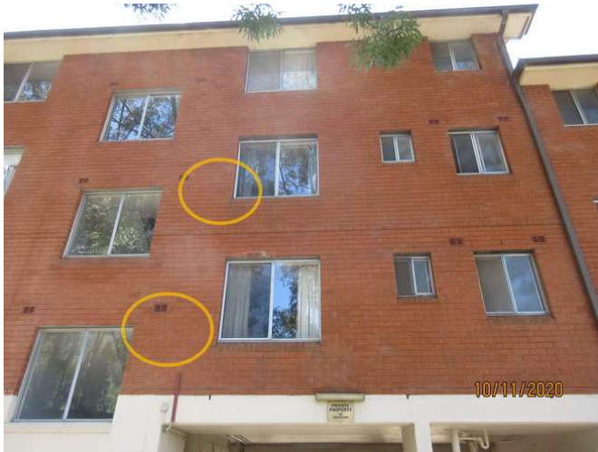
No 1-3_085_Note the cracking damage
