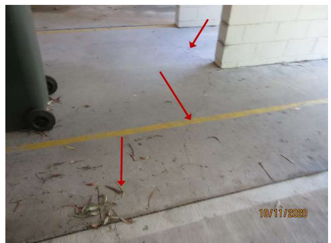
No 1-3_468_Note the cracking damage
