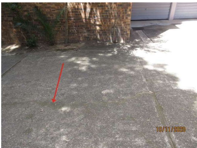
No1_095_Note evident cracking to concrete driveway
