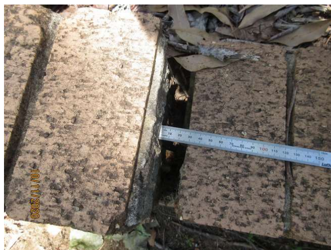
No 3_020_Note an estimated 28.0mm width of opening
