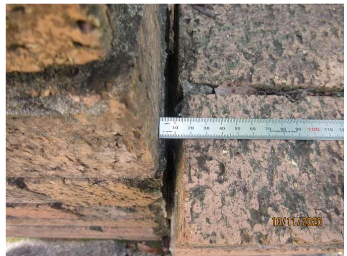
No 3_016_Note an estimated 15mm width of opening
