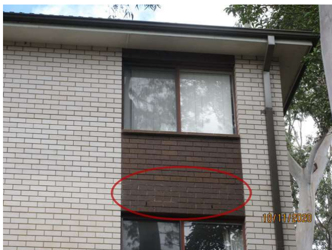
No 5_025_Note re-addressing to course joints
