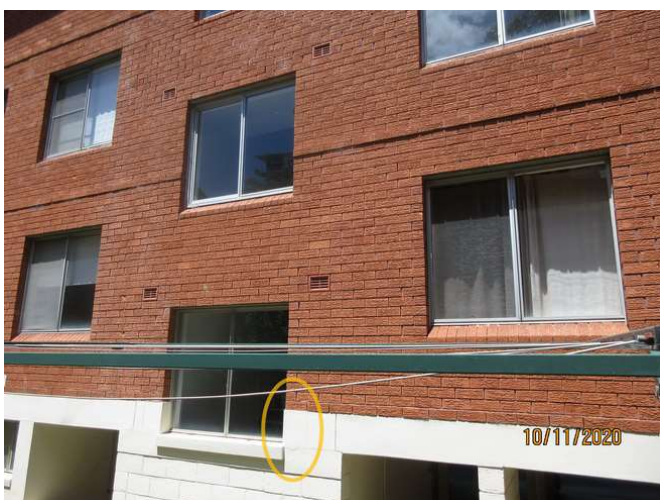
No 1-3_143_Note the cracking damage
