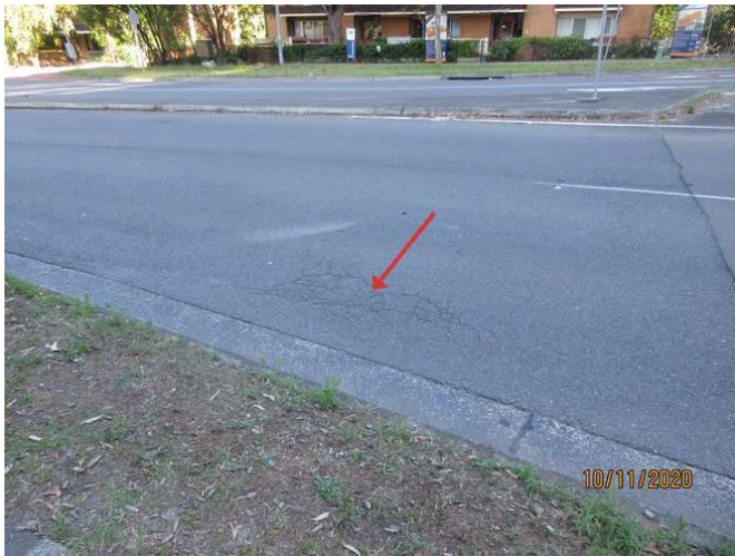
183_Note cracking damage
