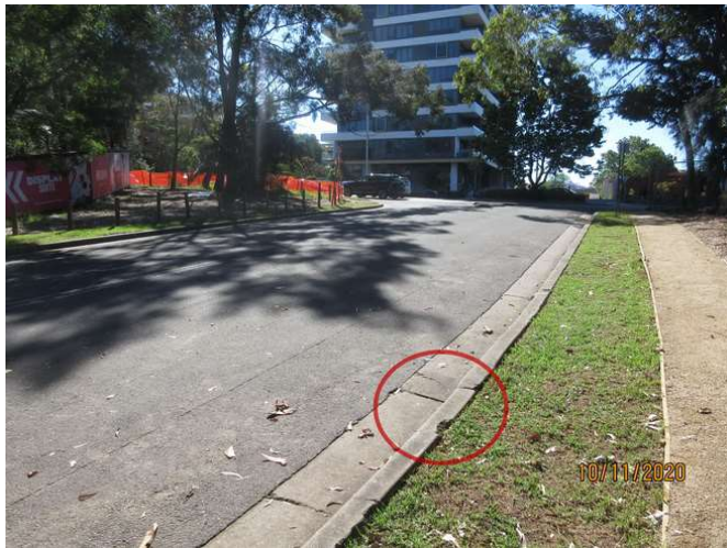
003_Note cracking damage
