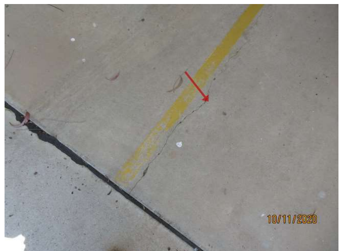
No 1-3_174_Note the cracking damage
