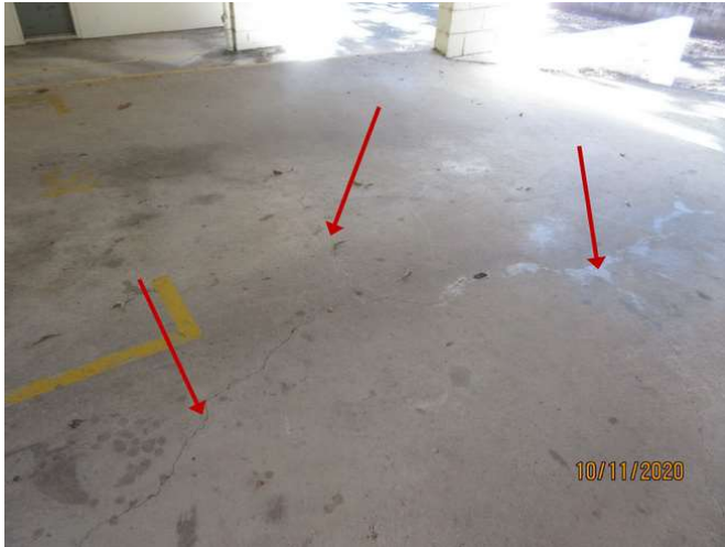
No 1-3_523_Note the cracking damage
