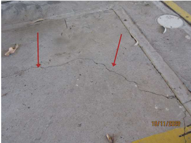
No 1-3_253_Note the cracking damage
