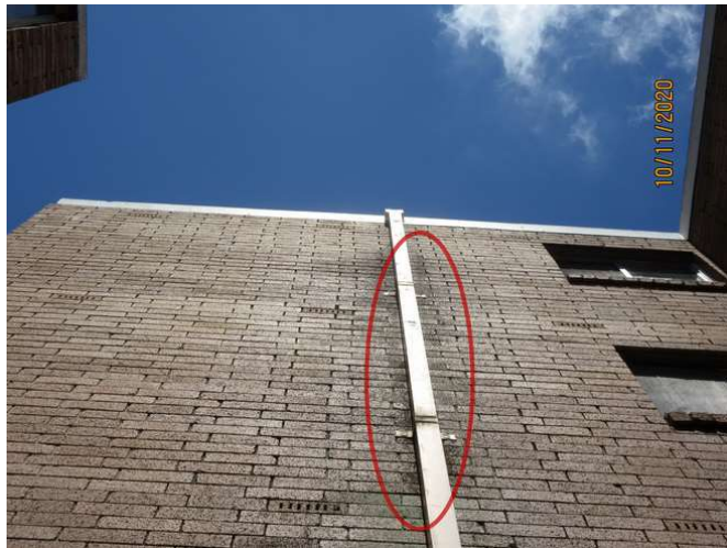
No 3_087_Note the sign of overflow roof water
