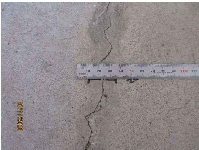
No 1-3_305_Note an estimated 0.5mm cracking width at representative location
