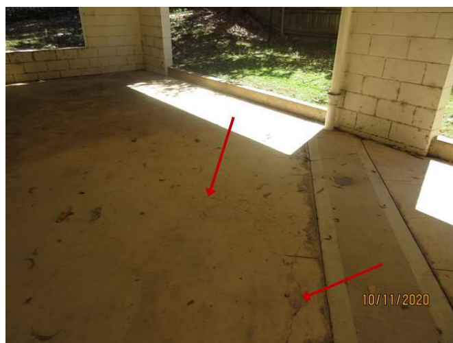
No 1-3_552_Note the cracking damage
