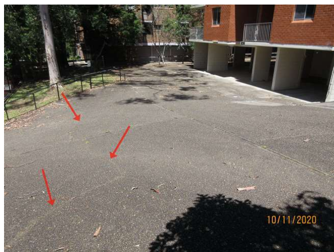
No 1-3_058_Note the cracking damage
