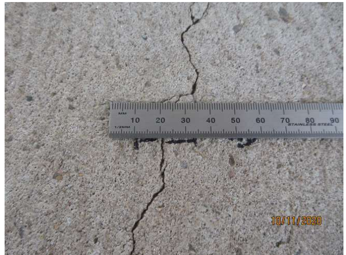
No 5_124_Note an estimated 1.0mm cracking width at representative location
