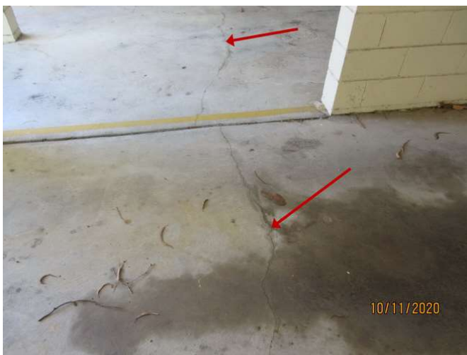
No 1-3_341_Note the cracking damage
