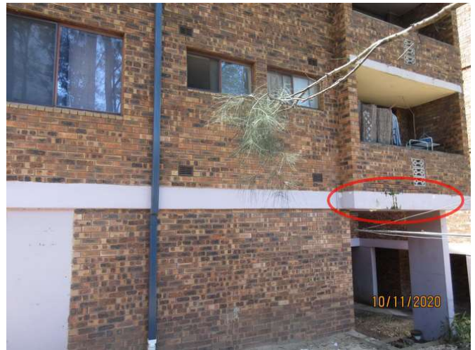
No1_052_Note slight concrete spalling
