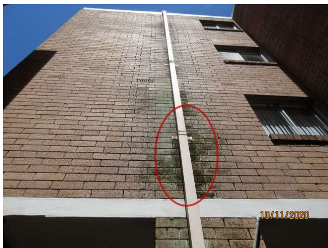
No 3_089_Note the sign of overflow roof water
