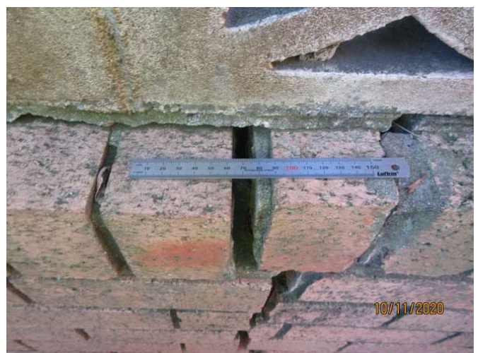
No 155_096_Note an estimated 28.0mm opening on top
