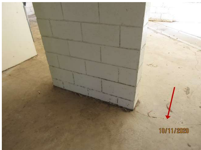
No 1-3_547_Note the cracking damage
