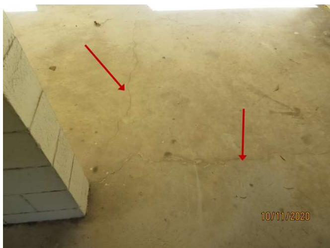
No 1-3_567_Note the cracking damage
