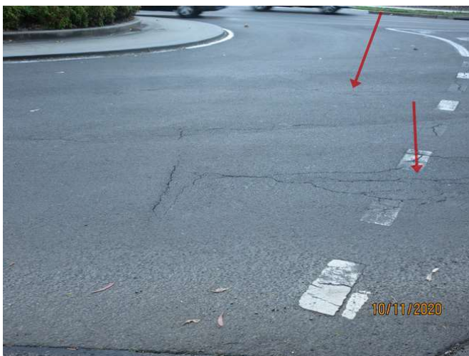
029_Note cracking damage
