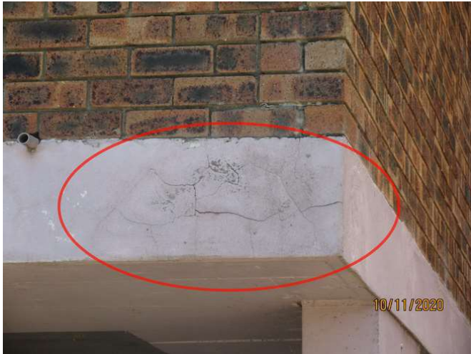
No1_067_Note slight concrete spalling
