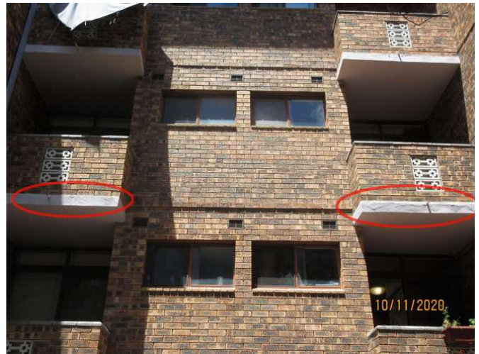
No1_088_Note slight concrete spalling
