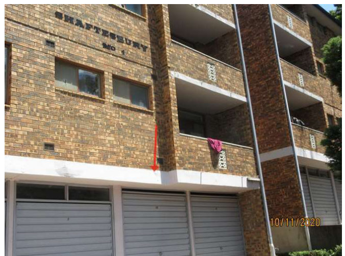
No1_012_Note slight concrete spalling
