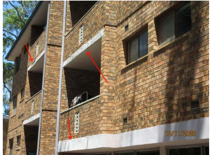
No1_020_Note slight concrete spalling
