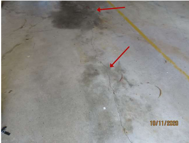
No 1-3_307_Note the cracking damage
