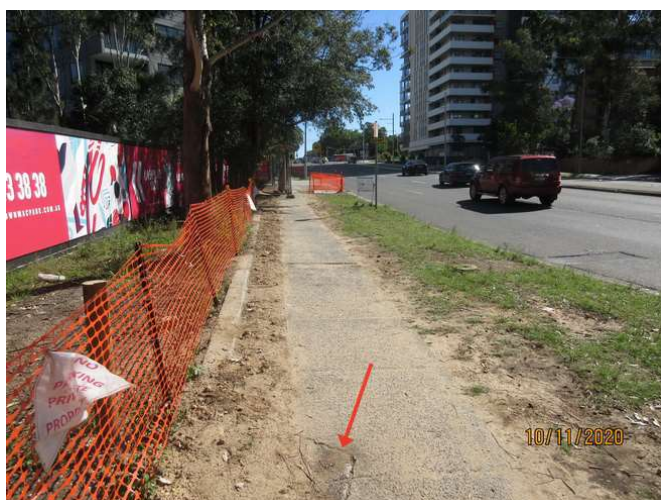
047_Note cracking damage_Note exposed soil ground along footpath
