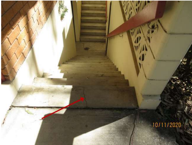
No 155_043_Note the cracking damage
