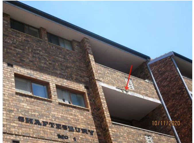
No1_008_Note slight concrete spalling
