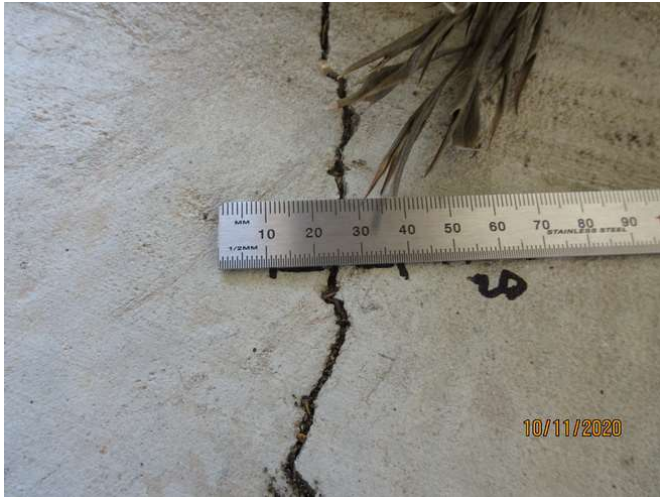
No 1-3_223_Note an estimated 2.0mm cracking width at representative location
