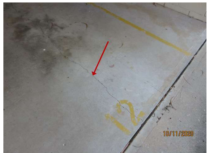
No 1-3_306_Note the cracking damage
