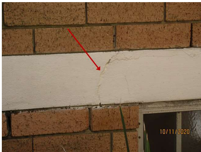
No 3_135_Note the cracking damage
