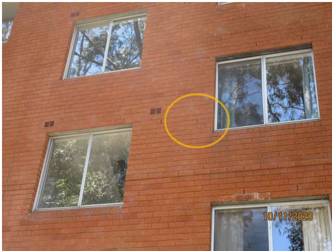
No 1-3_087_Note the cracking damage
