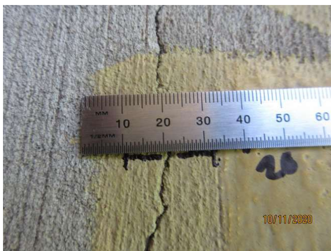
No 1-3_413_Note an estimated 0.5mm cracking width at representative location
