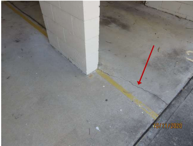
No 1-3_325_Note the cracking damage
