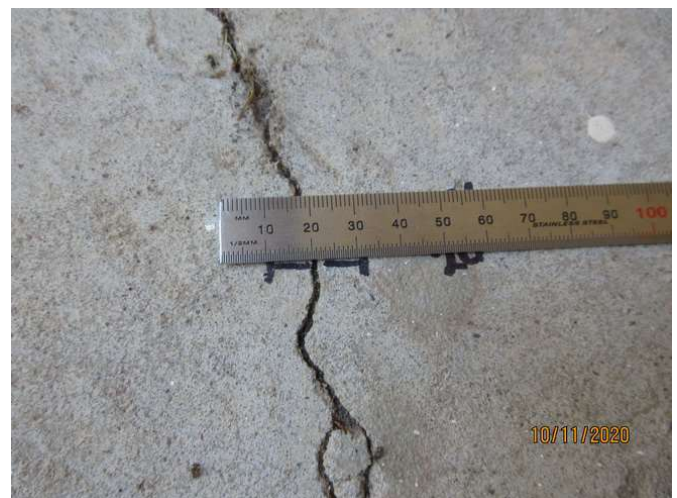
No 1-3_426_Note an estimated 1.0mm cracking width at representative location
