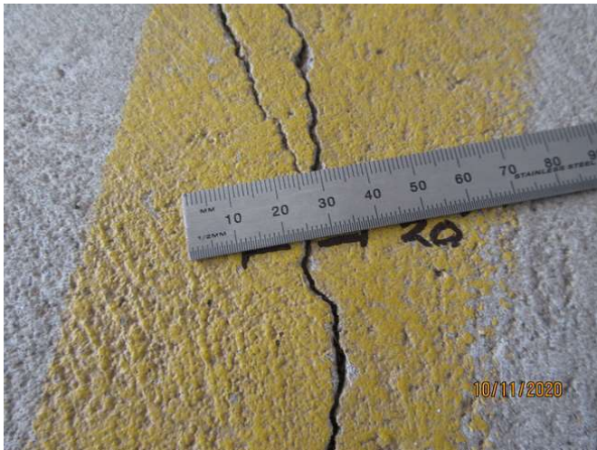
No 5_165_Note an estimated 1.0mm cracking width at representative location
