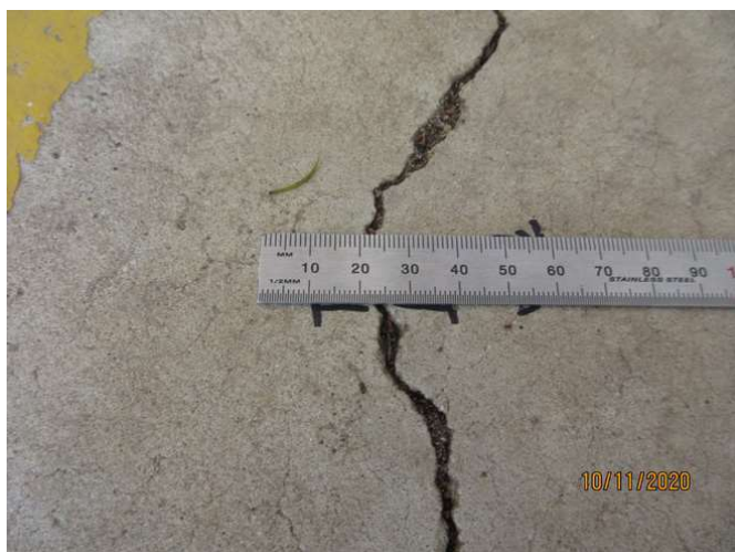
No 1-3_211_Note an estimated 2.0mm cracking width at representative location
