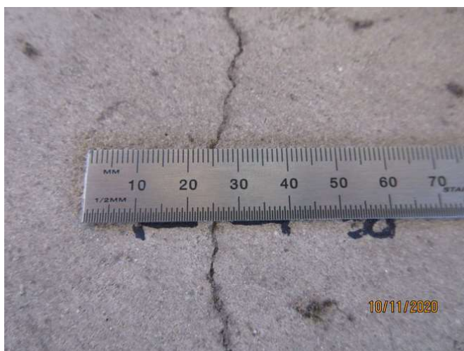
No 1-3_275_Note an estimated 0.5mm cracking width at representative location
