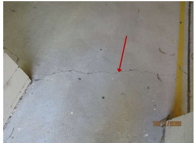
No 1-3_424_Note the cracking damage
