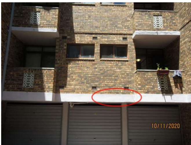
No1_089_Note slight concrete spalling
