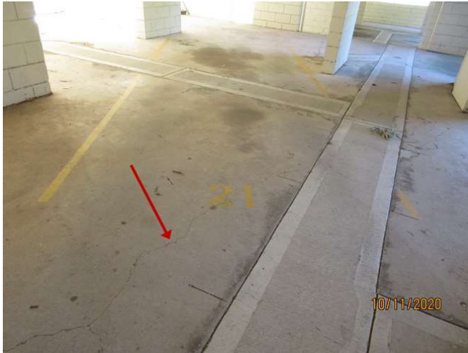
No 1-3_529_Note the cracking damage
