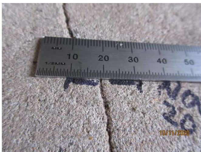
No 7_221_Note an estimated 0.5mm cracking width at representative location
