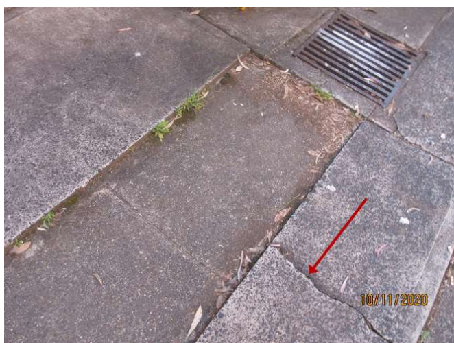
No 155_083_Note cracking damage
