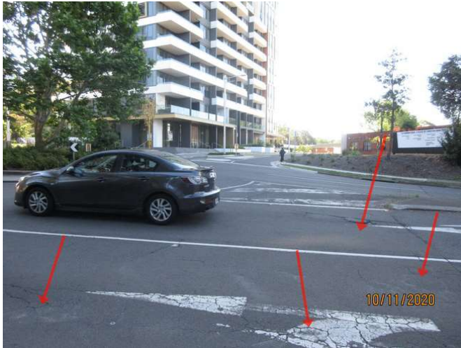
277_Note cracking damage
