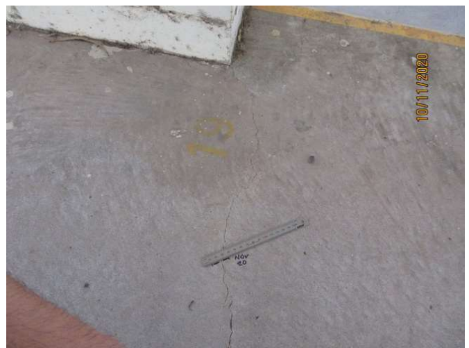
No 1-3_516_Note the cracking damage
