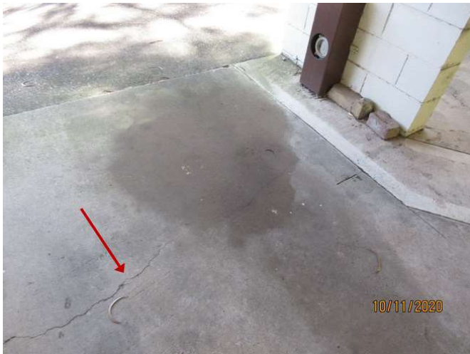
No 1-3_495_Note the cracking damage
