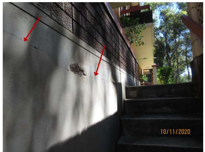
No 155_040_Note the cracking damage
