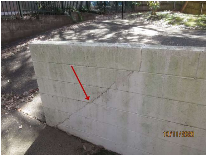
No 1-3_507_Note structual distress to block wall
