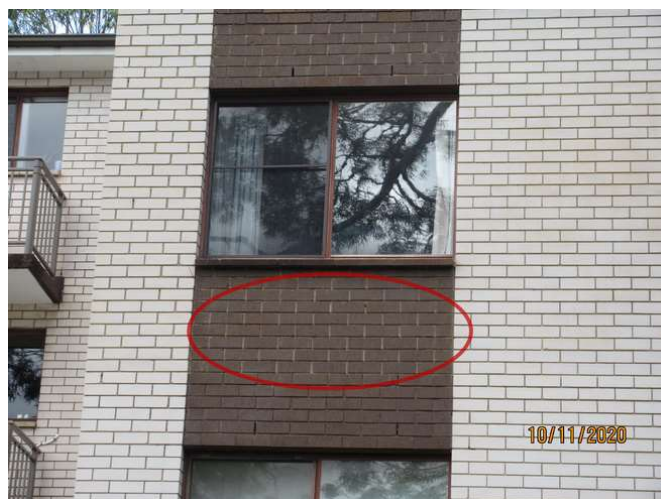
No 5_026_Note re-addressing to course joints
