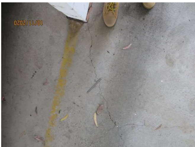
No 5_125_Note cracking generally noted to concrete slab
