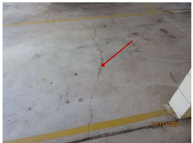
No 1-3_342_Note the cracking damage
