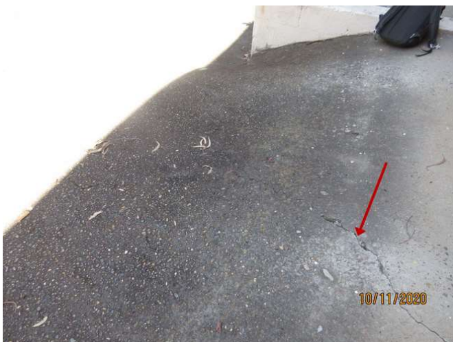
No 1-3_407_Note the cracking damage
