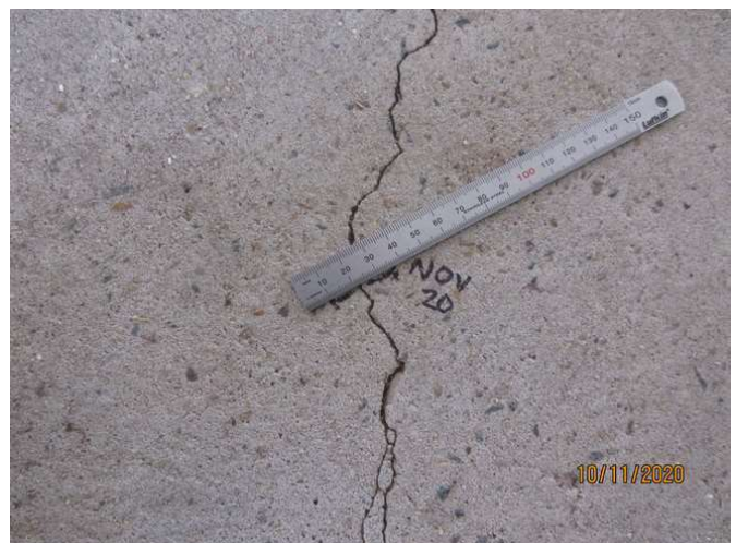
No 5_126_Note an estimated 2.0mm cracking width at representative location
