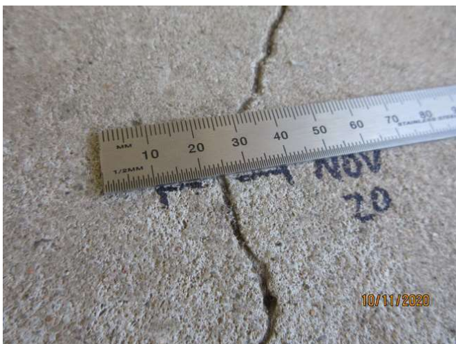
No 1-3_497_Note an estimated 2.0mm cracking width at representative location
