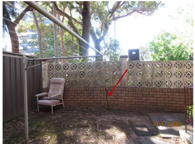
No 155_092_Distressed brick wall
