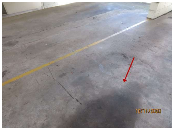
No 1-3_312_Note the cracking damage
