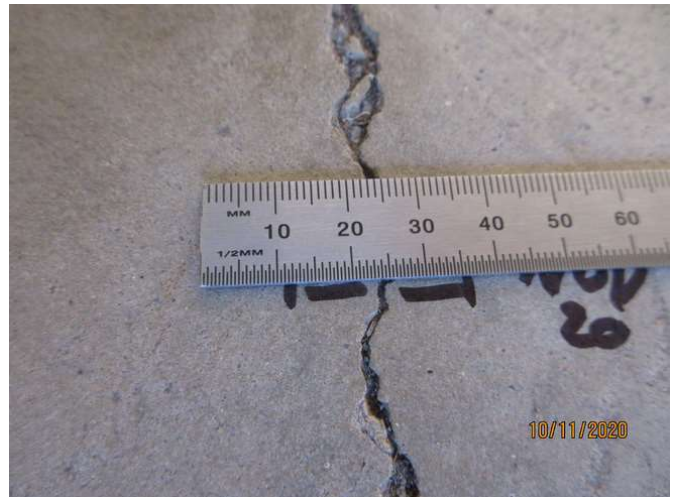
No 1-3_574_Note an estimated 1.0mm cracking width at representative location
