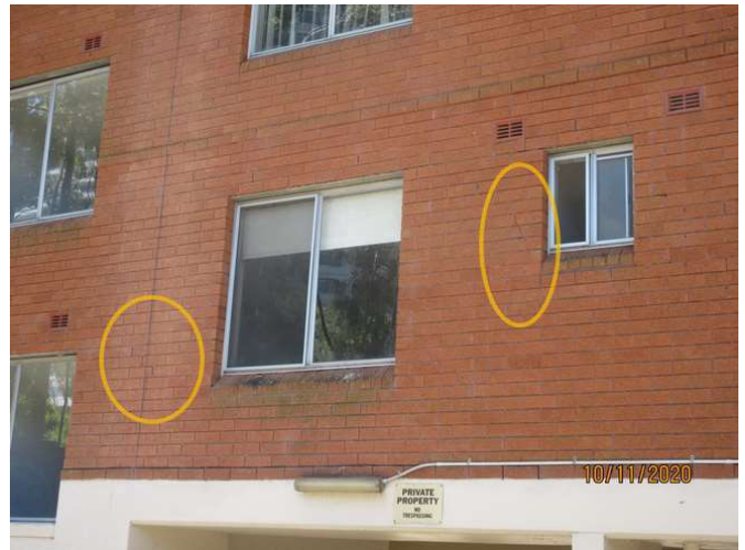
No 1-3_076_Note the cracking damage
