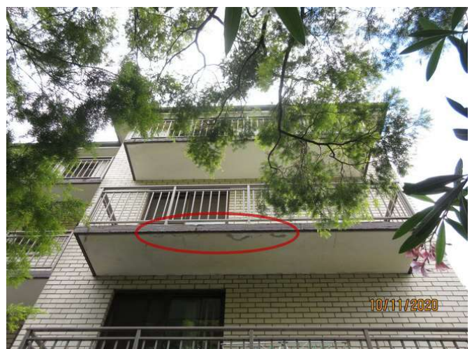
No 5_048_Note water damage
