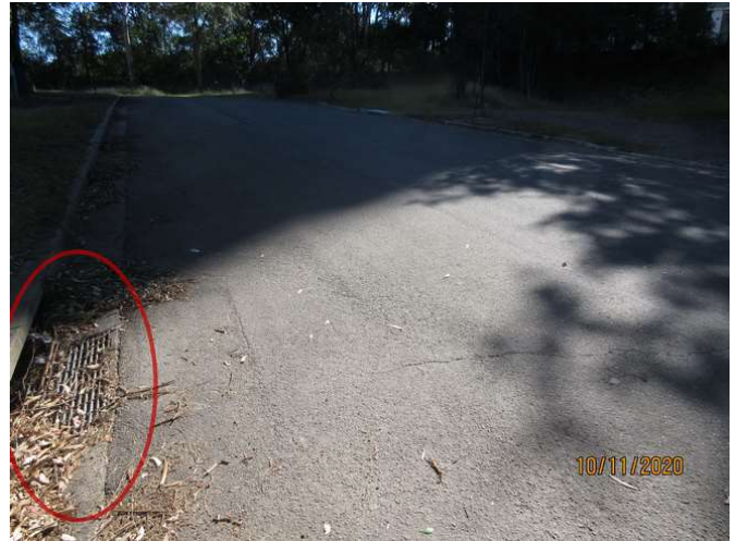
008_Road drains generally noted with leave blockage
