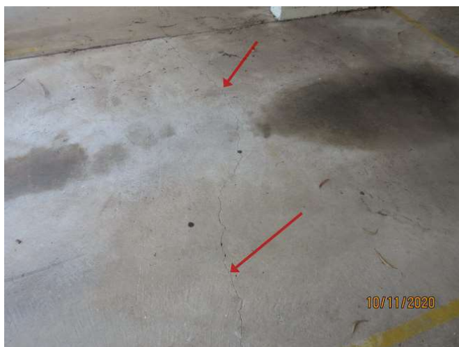
No 1-3_212_Note the cracking damage
