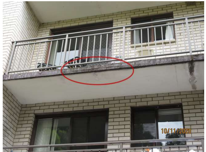
No 5_044_Note water damage
