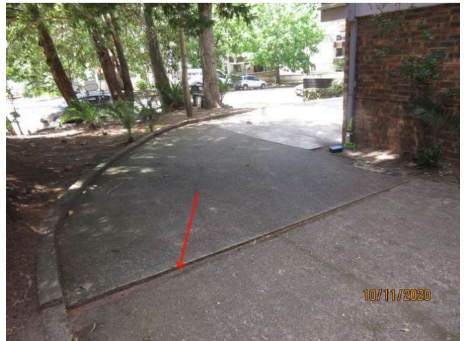
No1_094_Note dropping in levelling to the eastern driveway
