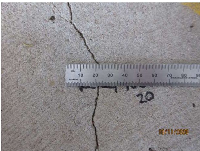
No 5_167_Note an estimated 1.5mm cracking width at representative location
