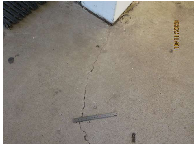
No 1-3_530_Note the cracking damage
