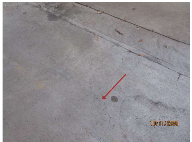
No 1-3_270_Note the cracking damage
