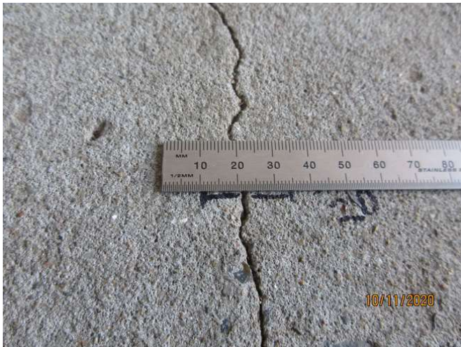
No 5_231_Note an estimated 1.5mm cracking width at representative location
