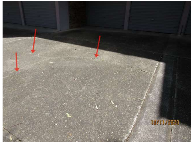
No1_046_Note evident cracking to concrete driveway
