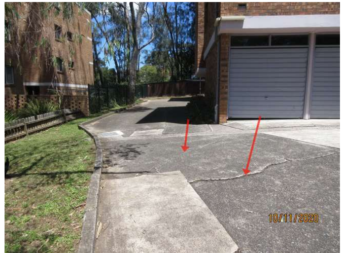
No1_004_Note evident cracking to concrete driveway
