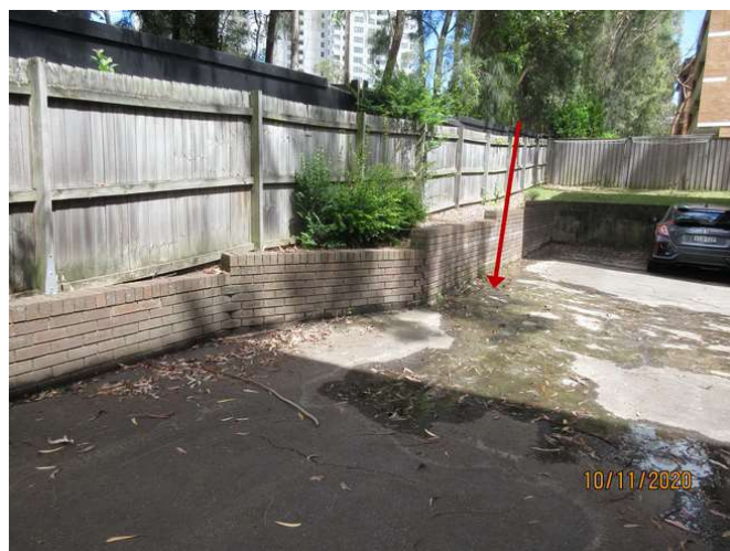
No 5_098_Note groud n water leakage
