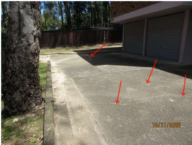
No1_045_Note evident cracking to concrete driveway
