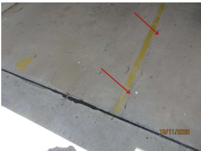
No 1-3_173_Note the cracking damage
