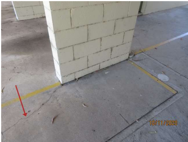
No 1-3_249_Note the cracking damage
