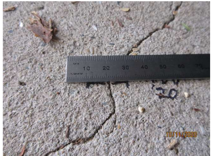
No 7_208_Note an estimated 1.5mm cracking width at representative location
