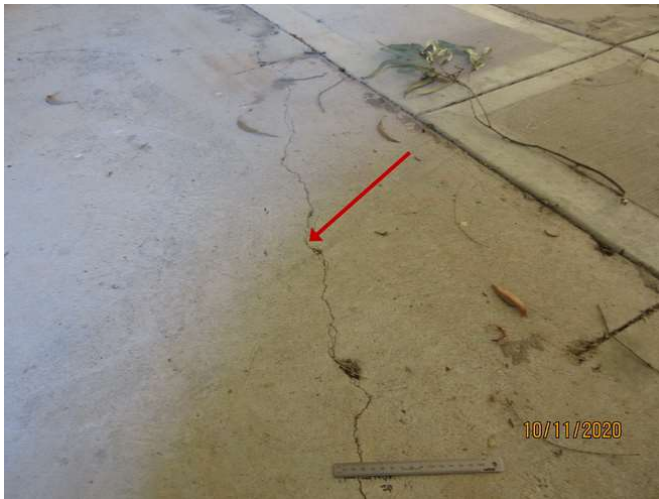
No 1-3_537_Note the cracking damage
