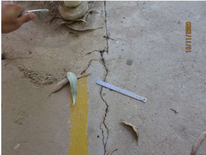
No 1-3_451_Note the cracking damage
