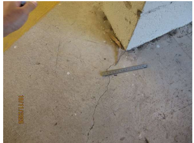
No 1-3_544_Note the cracking damage
