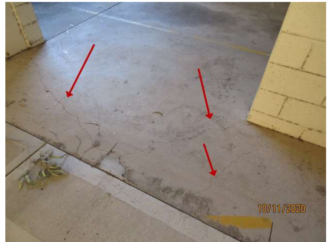
No 1-3_532_Note the cracking damage
