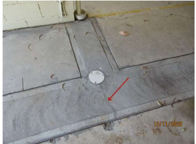
No 1-3_206_Note the cracking damage
