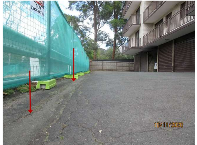
No 7_056_Note elevation dropping next to deep excavation
