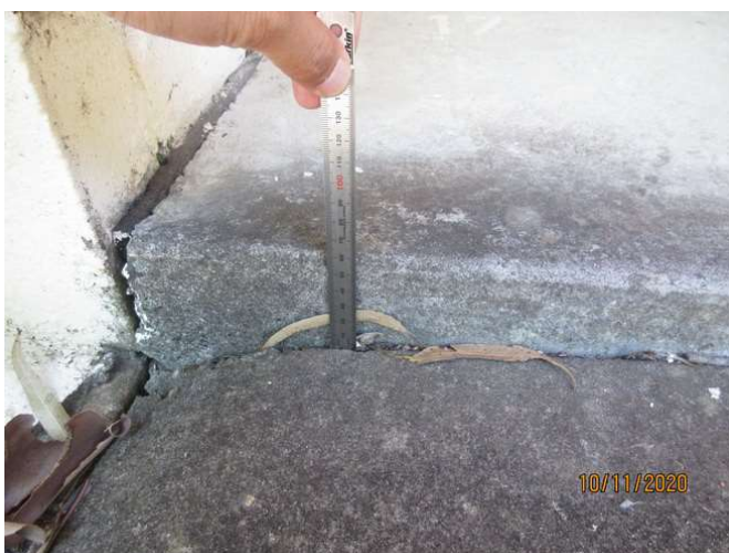
No 1-3_401_60mm dropping in level
