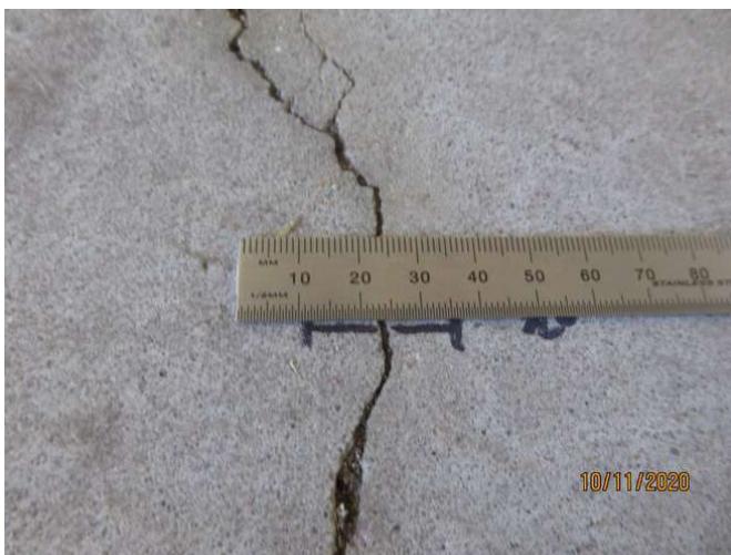
No 1-3_389_Note an estimated 1.5mm cracking width at representative location
