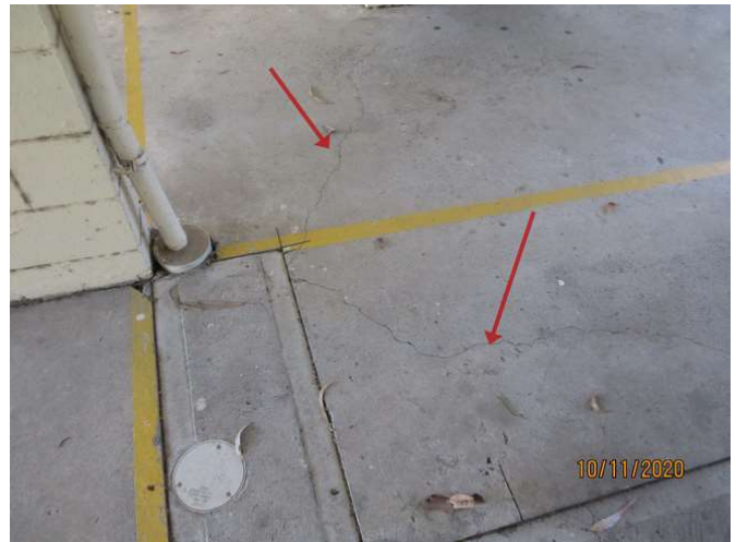
No 1-3_250_Note the cracking damage
