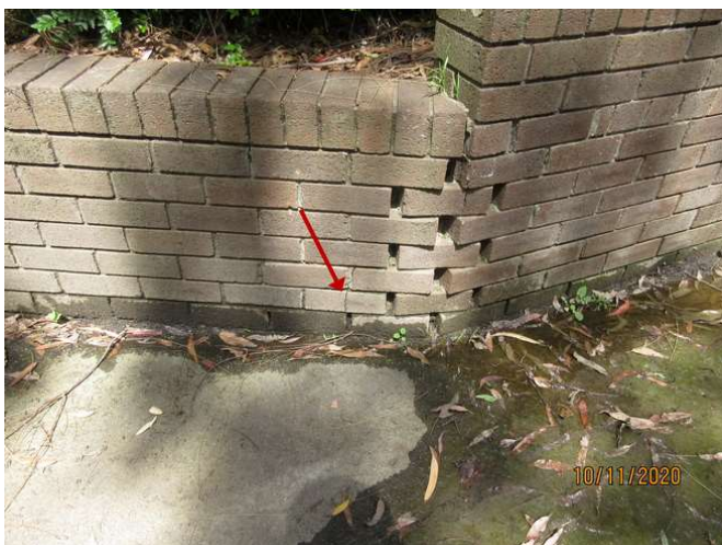
No 5_107_Note the cracking damage
