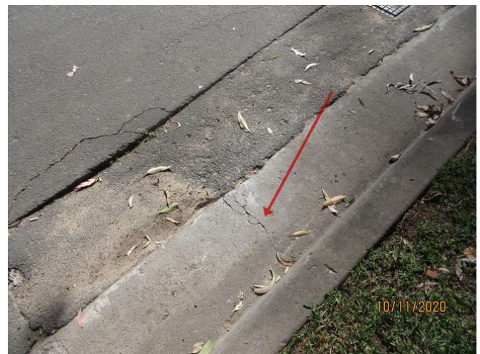
022_Note cracking damage
