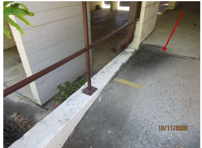
No 1-3_400_Note the dropping in level
