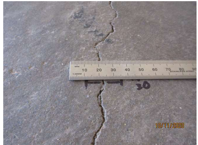
No 1-3_220_Note an estimated 1.0mm cracking width at representative location
