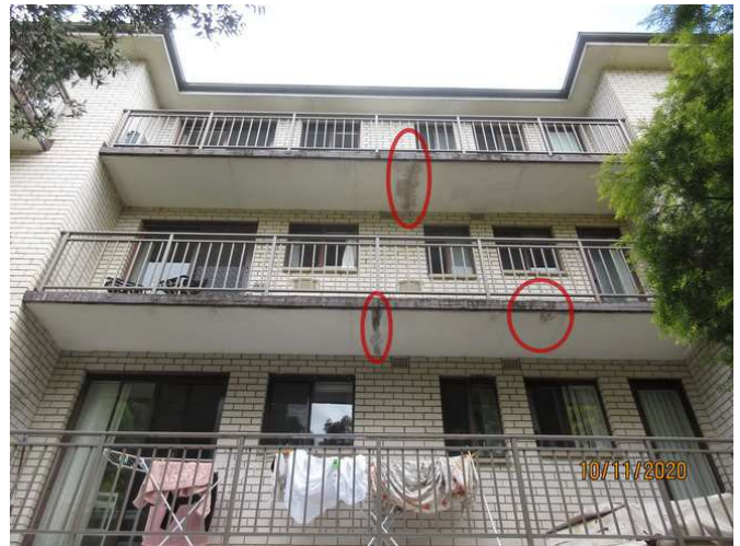
No 5_040_Note water damage
