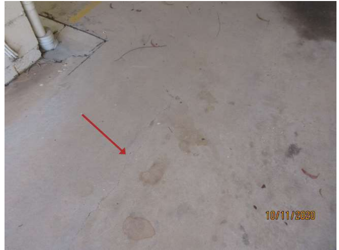
No 1-3_170_Note the cracking damage
