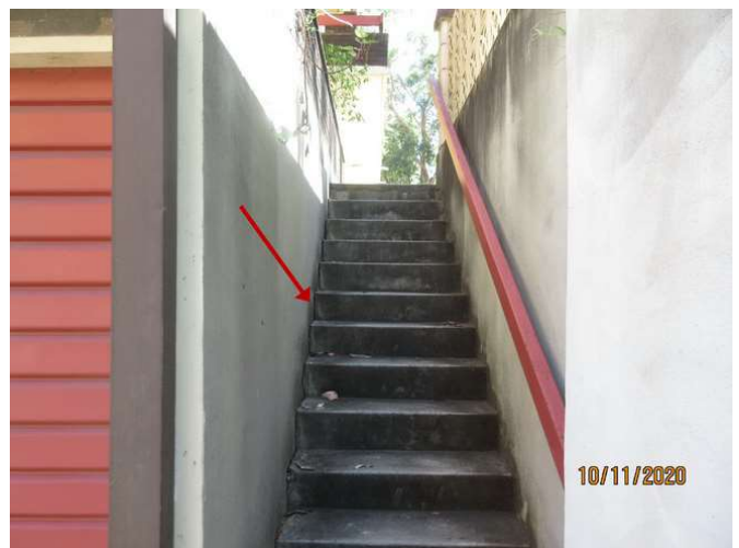
No 155_030_Note the opening to staircase edge
