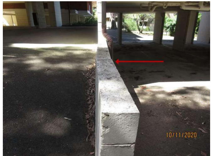
No 1-3_508_Note CAT-3 structual distress to block wall
