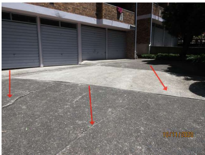
No1_005_Note evident cracking to concrete driveway
