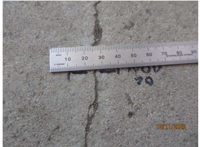
No 1-3_338_Note an estimated 2.0mm cracking width at representative location
