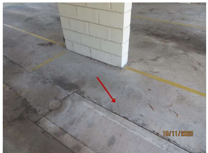
No 1-3_354_Note the cracking damage
