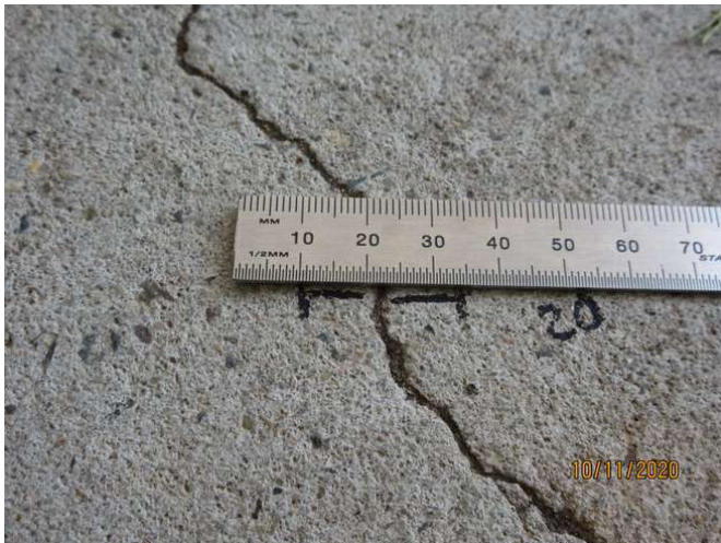
No 5_213_Note an estimated 2.0mm cracking width at representative location
