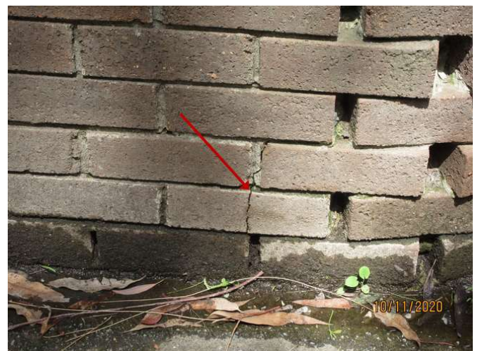
No 5_108_Note the cracking damage
