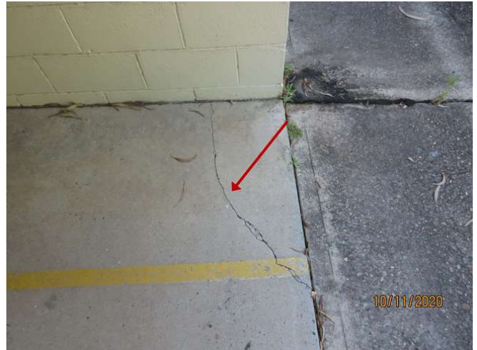
No 1-3_416_Note the cracking damage
