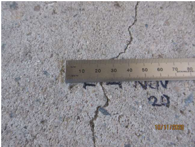
No 1-3_261_Note an estimated 1.5mm cracking width at representative location
