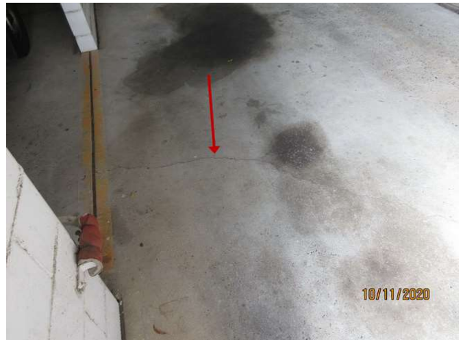
No 7_166_Cracking generally noted to concrete slab
