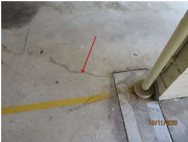
No 1-3_303_Note the cracking damage
