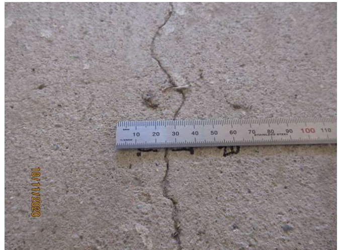
No 1-3_238_Note an estimated 1.0mm cracking width at representative location
