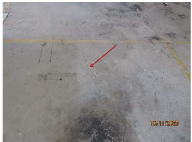
No 1-3_234_Note the cracking damage
