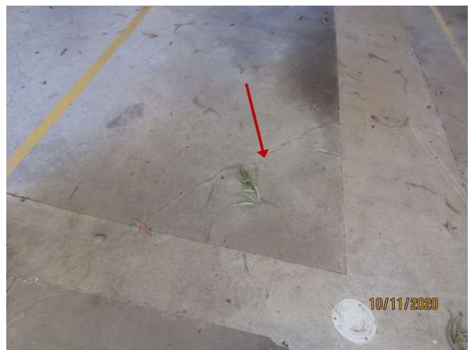
No 1-3_336_Note the cracking damage
