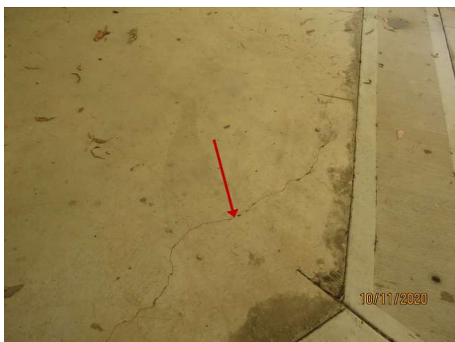
No 1-3_551_Note the cracking damage
