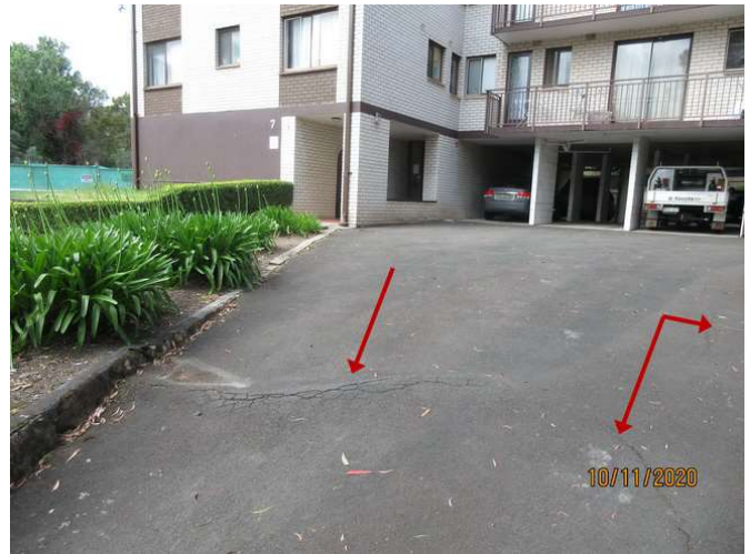
No 7_148_Note distressed road surface
