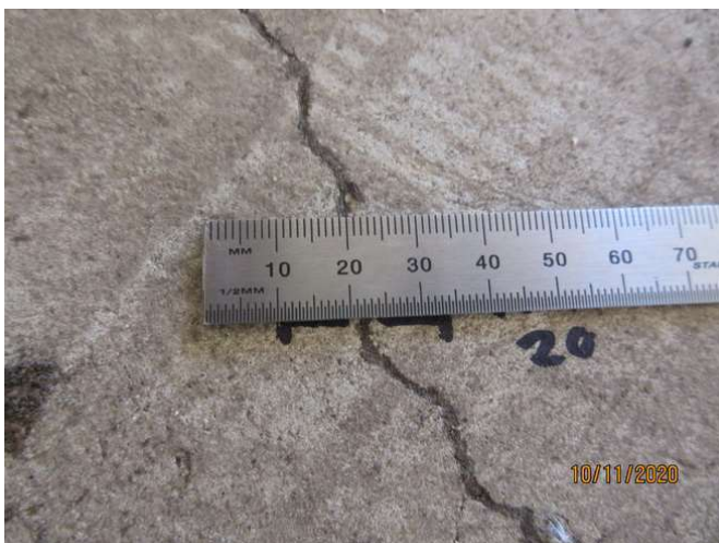
No 1-3_245_Note an estimated 2.0mm cracking width at representative location
