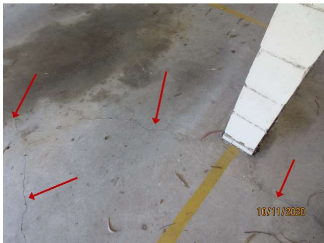
No 1-3_373_Note the cracking damage
