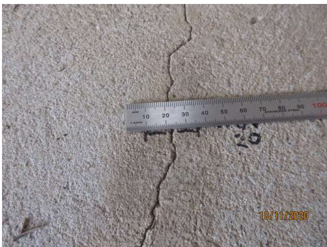
No 5_203_Note an estimated 2.0mm cracking width at representative location
