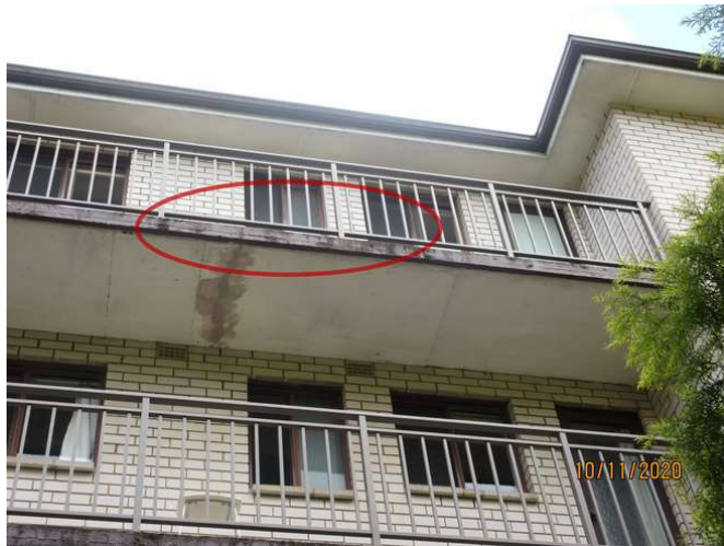
No 5_043_Note water damage
