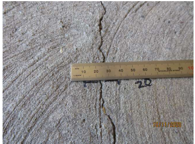
No 1-3_208_Note an estimated 1.5mm cracking width at representative location
