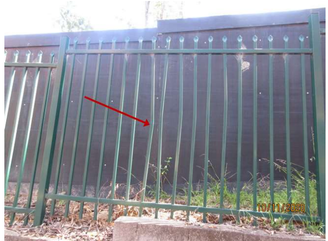
No 1-3_608_Note impact to metal railing fence
