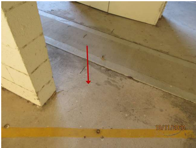
No 1-3_543_Note the cracking damage
