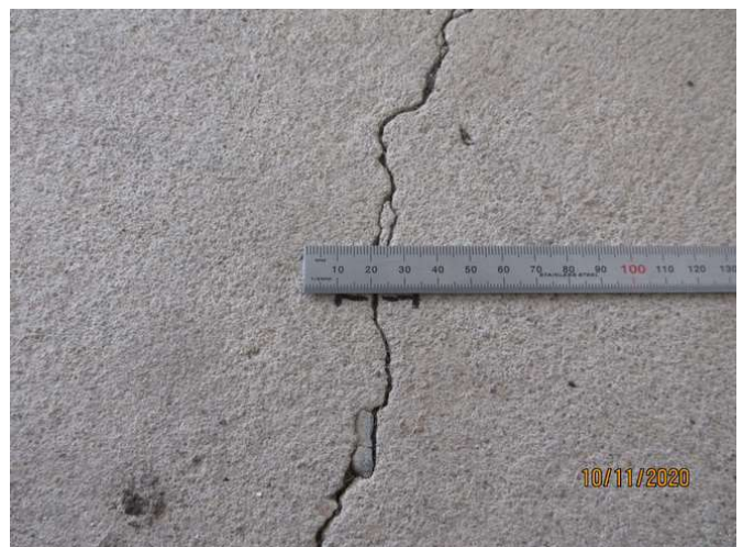
No 5_144_Note an estimated 2.0mm cracking width at representative location
