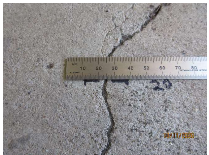
No 1-3_504_Note an estimated 1.5mm cracking width at representative location
