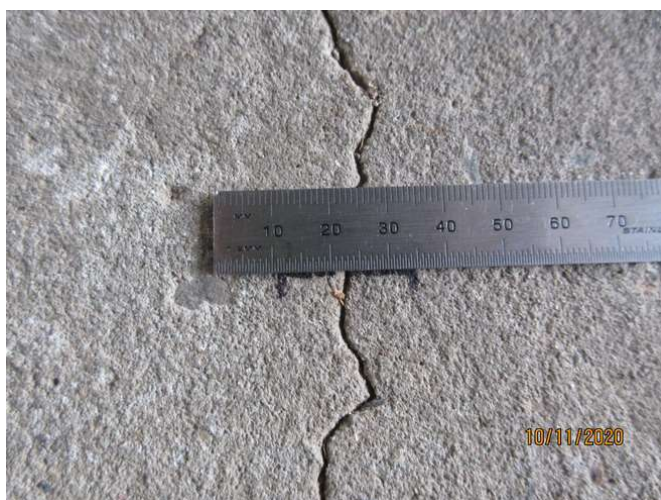
No 7_233_Note an estimated 1.0mm cracking width at representative location
