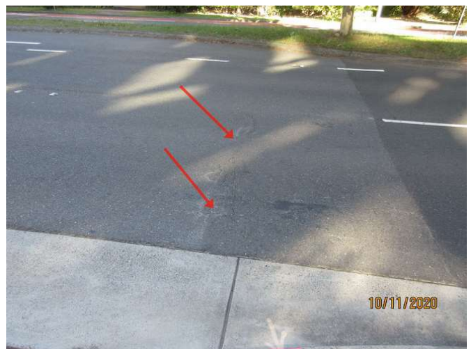
210_Note cracking damage
