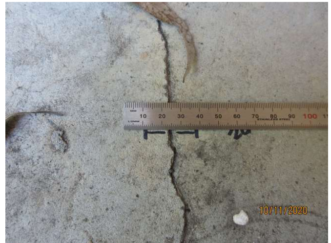
No 1-3_436_Note an estimated 1.5mm cracking width at representative location
