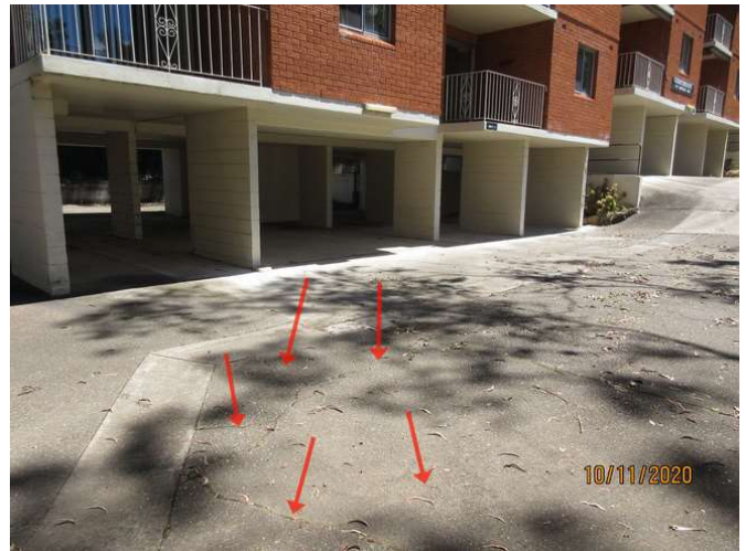
No 1-3_064_Note the cracking damage
