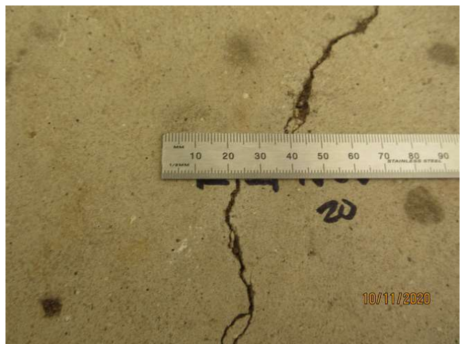
No 1-3_558_Note an estimated 1.0mm cracking width at representative location
