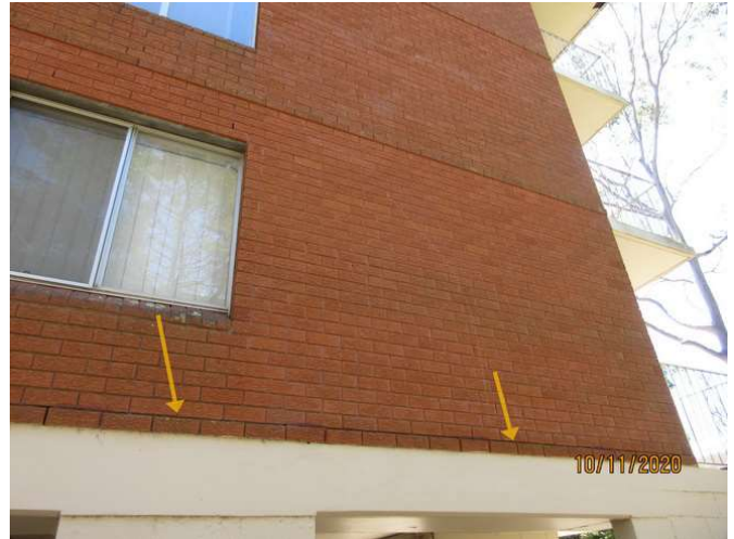
No 1-3_068_Note spalling to course joint lines
