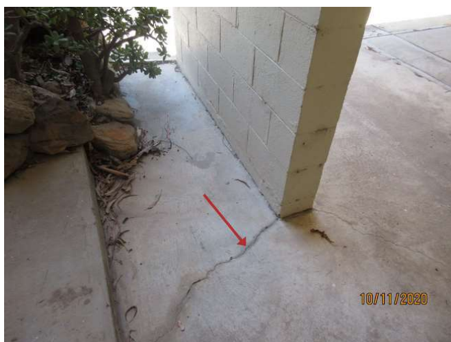
No 1-3_192_Note the cracking damage
