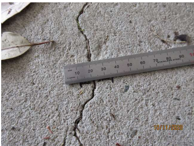
No 5_179_Note an estimated 1.5mm cracking width at representative location
