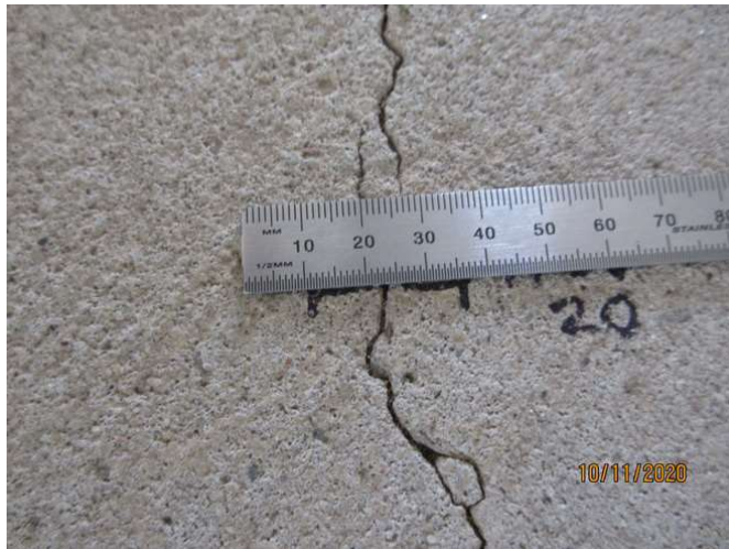
No 5_151_Note an estimated 1.5mm cracking width at representative location
