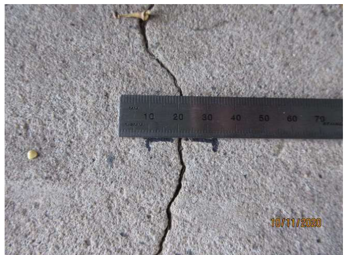
No 7_228_Note an estimated 1.0mm cracking width at representative location
