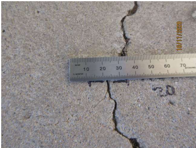
No 1-3_531_Note an estimated 1.0mm cracking width at representative location
