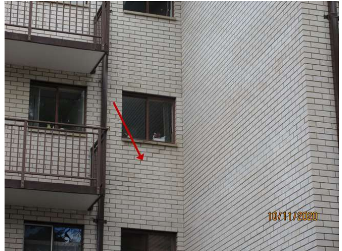
No 7_020_Note stepped cracking to wall
