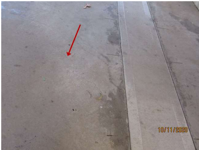
No 1-3_525_Note the cracking damage
