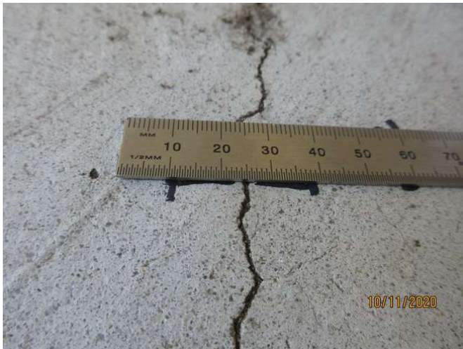
No 1-3_351_Note an estimated 1.5mm cracking width at representative location
