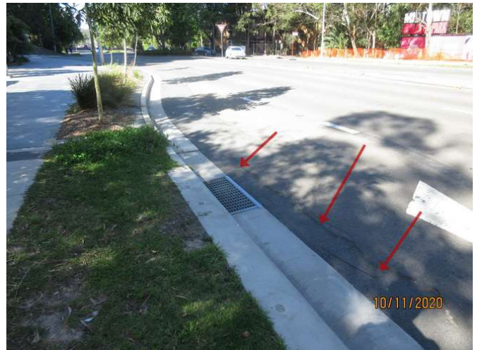
148_Note cracking damage
