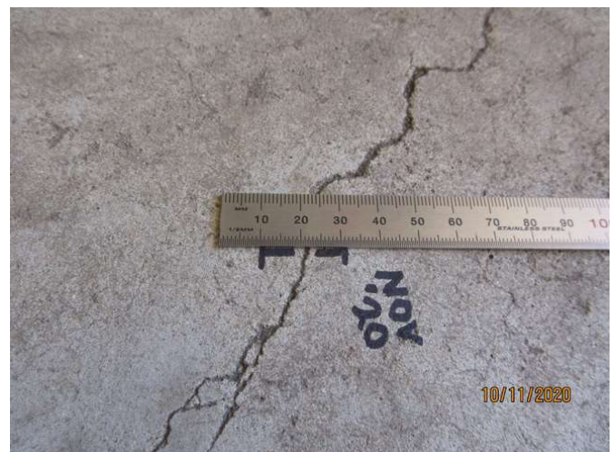
No 1-3_198_Note an estimated 1.5mm cracking width at representative location
