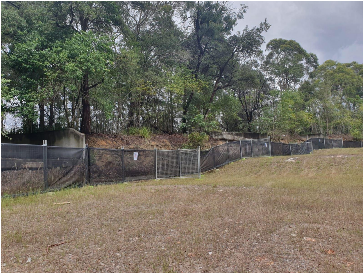
Plate 2: Representative example of chain mesh fence covered with black shade cloth used for Tree Protection Fencing at base of contour – outside of Mainland Civils limit of works and at outer extension of TPZ.
