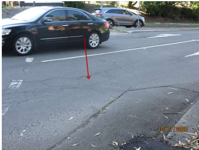
031_Note cracking damage
