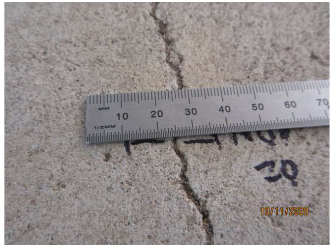
No 1-3_538_Note an estimated 1.0mm cracking width at representative location
