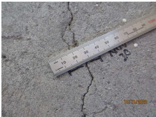
No 1-3_465_Note an estimated 1.0mm cracking width at representative location
