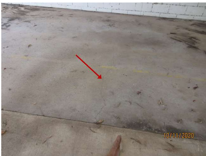
No 1-3_491_Note the cracking damage
