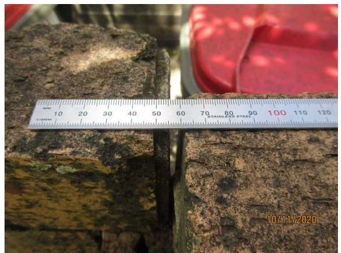
No 3_006_Note an estimated 13.0mm cracking width on top
