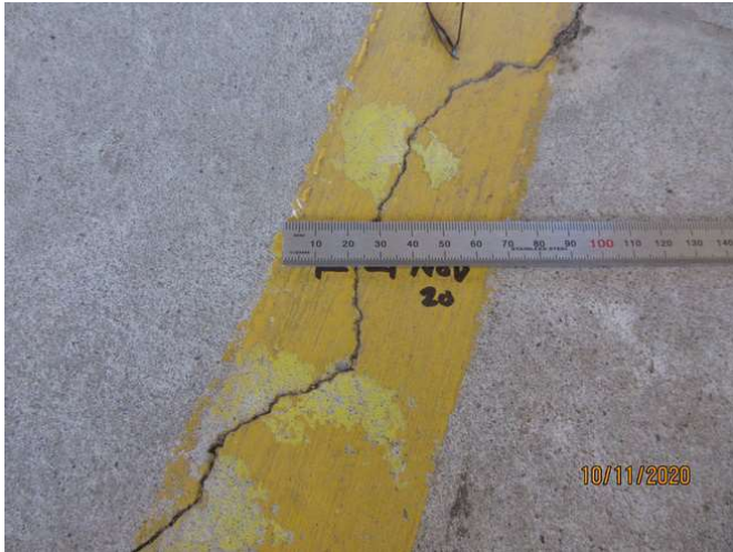
No 1-3_319_Note an estimated 1.5mm cracking width at representative location
