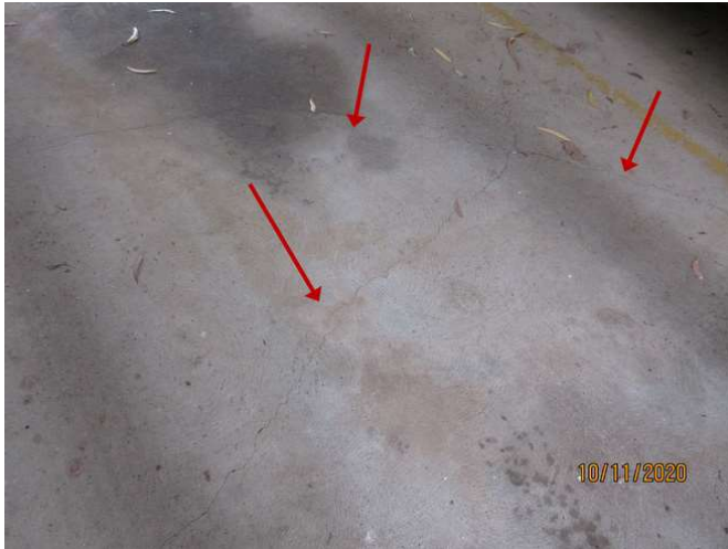
No 5_121_Note cracking generally noted to concrete slab
