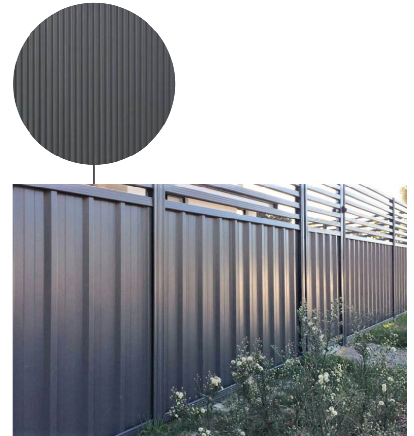
Fencing Type 03 Residential Boundary Fencing: Colourbond (0% transparency) 1.5m high with 0.3m high horizontal slats
