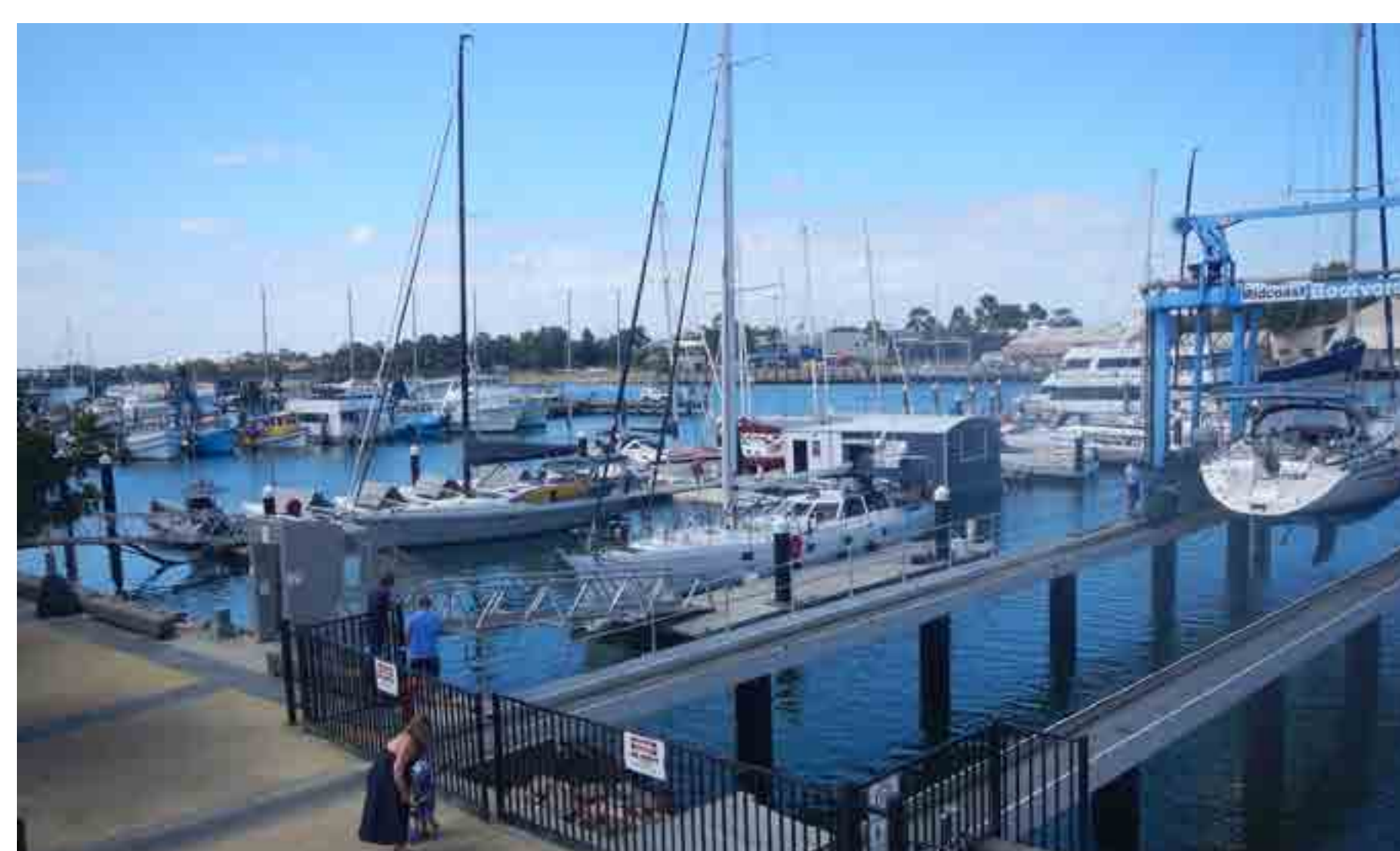
Example of a travel lift and safety gate at Midcoast Boatyard Newcastle
