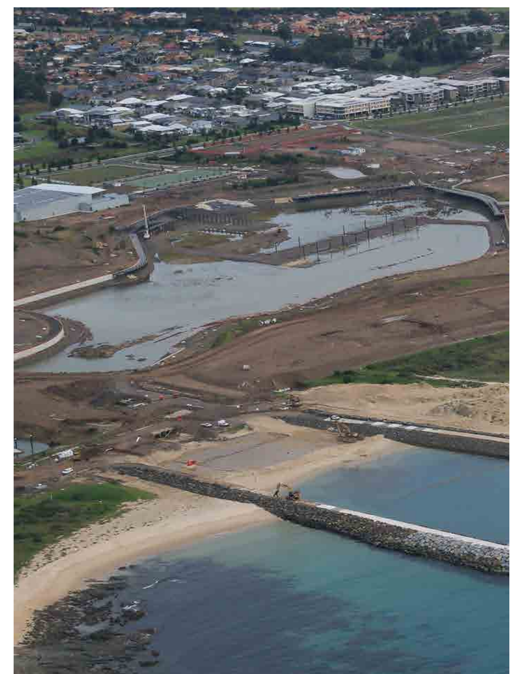
Aerial view of Inner Harbour construction April 2019
