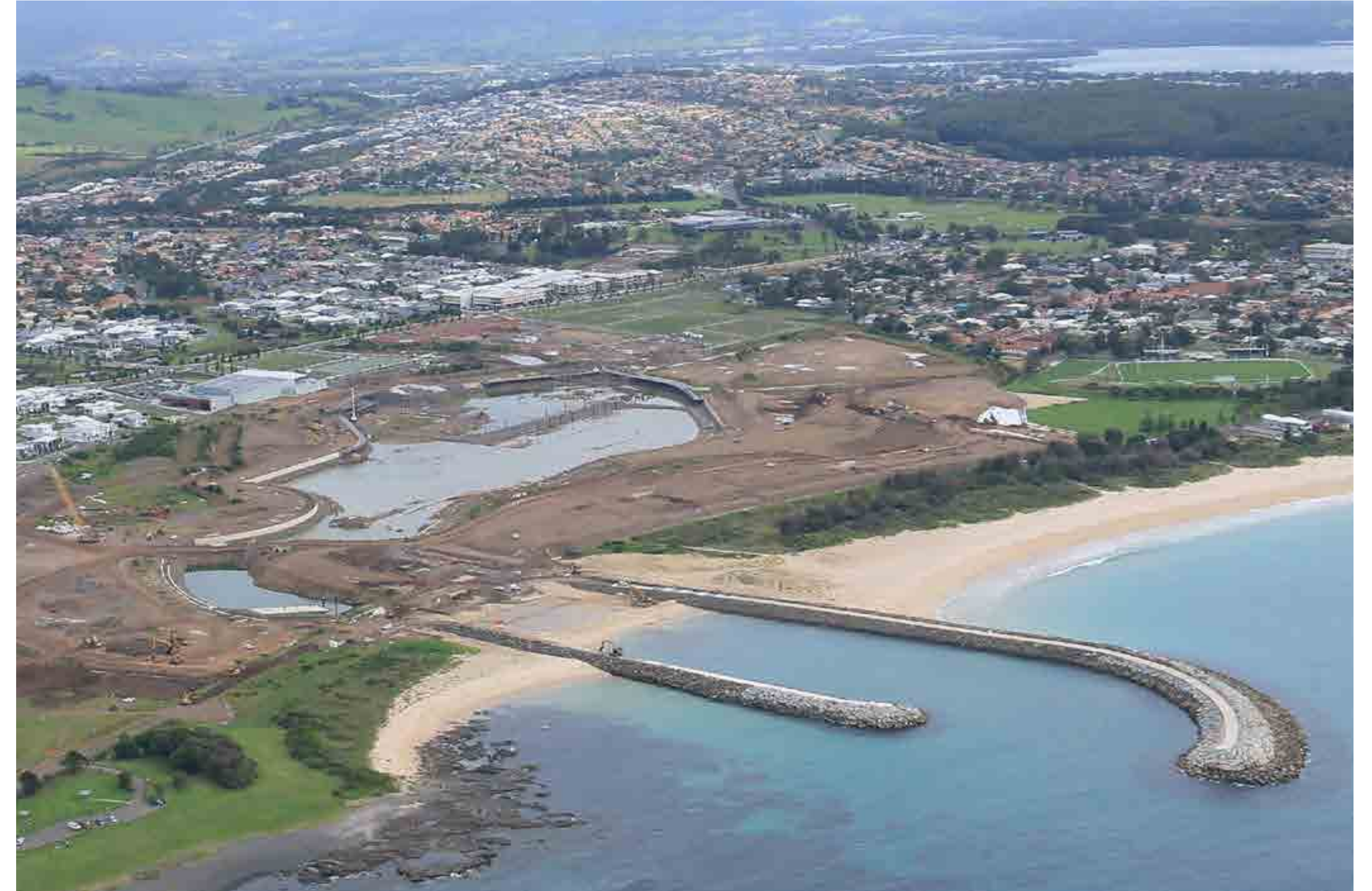
Aerial image of breakwater and groyne April 2019
